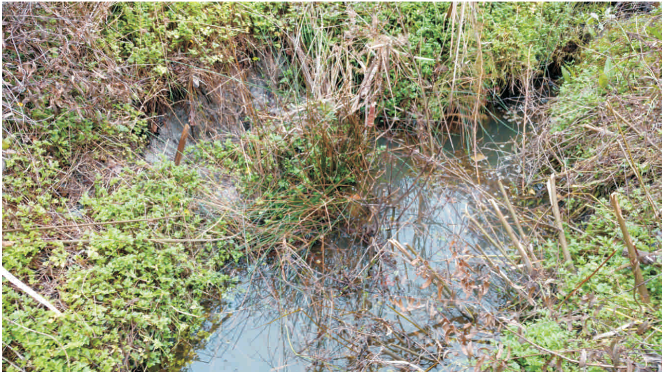
Reach 1A - Stream Problem Area #3; scour
