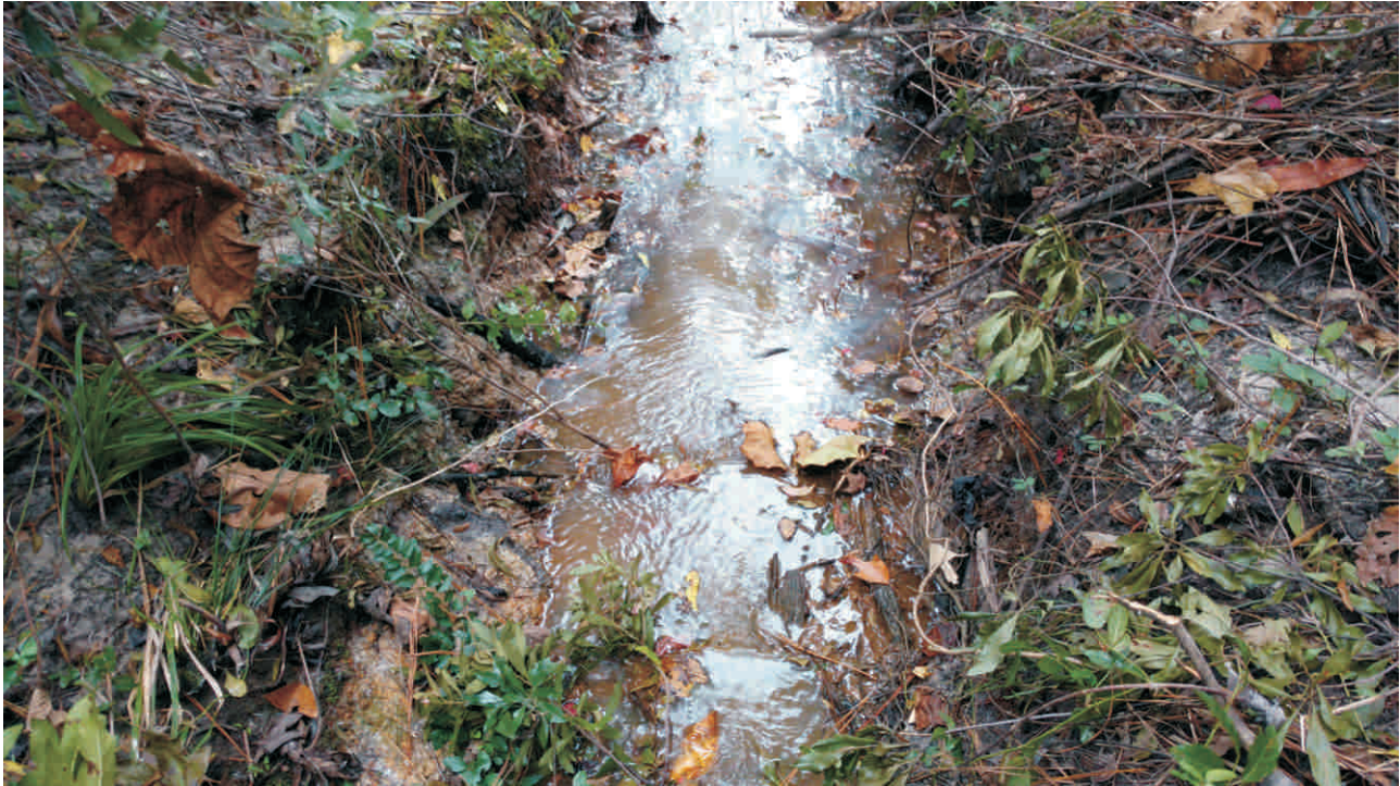
Reach 1A - Stream Problem Area #23; Degradation
