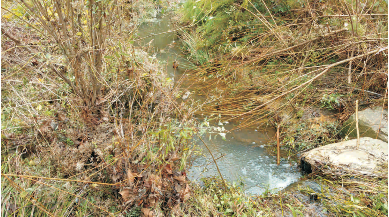
Reach 2A - Stream Problem Area #50; Undercut
