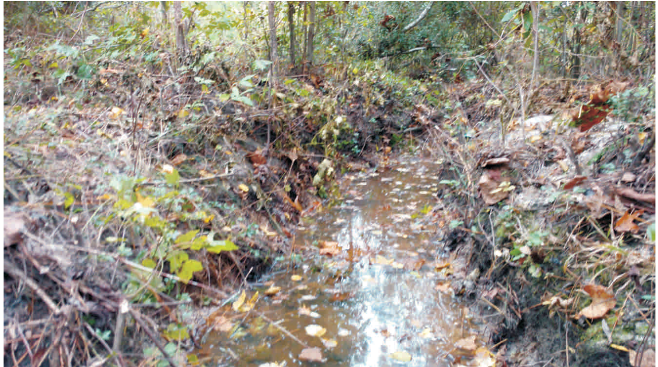
Reach 1A - Stream Problem Area #22; Degradation
