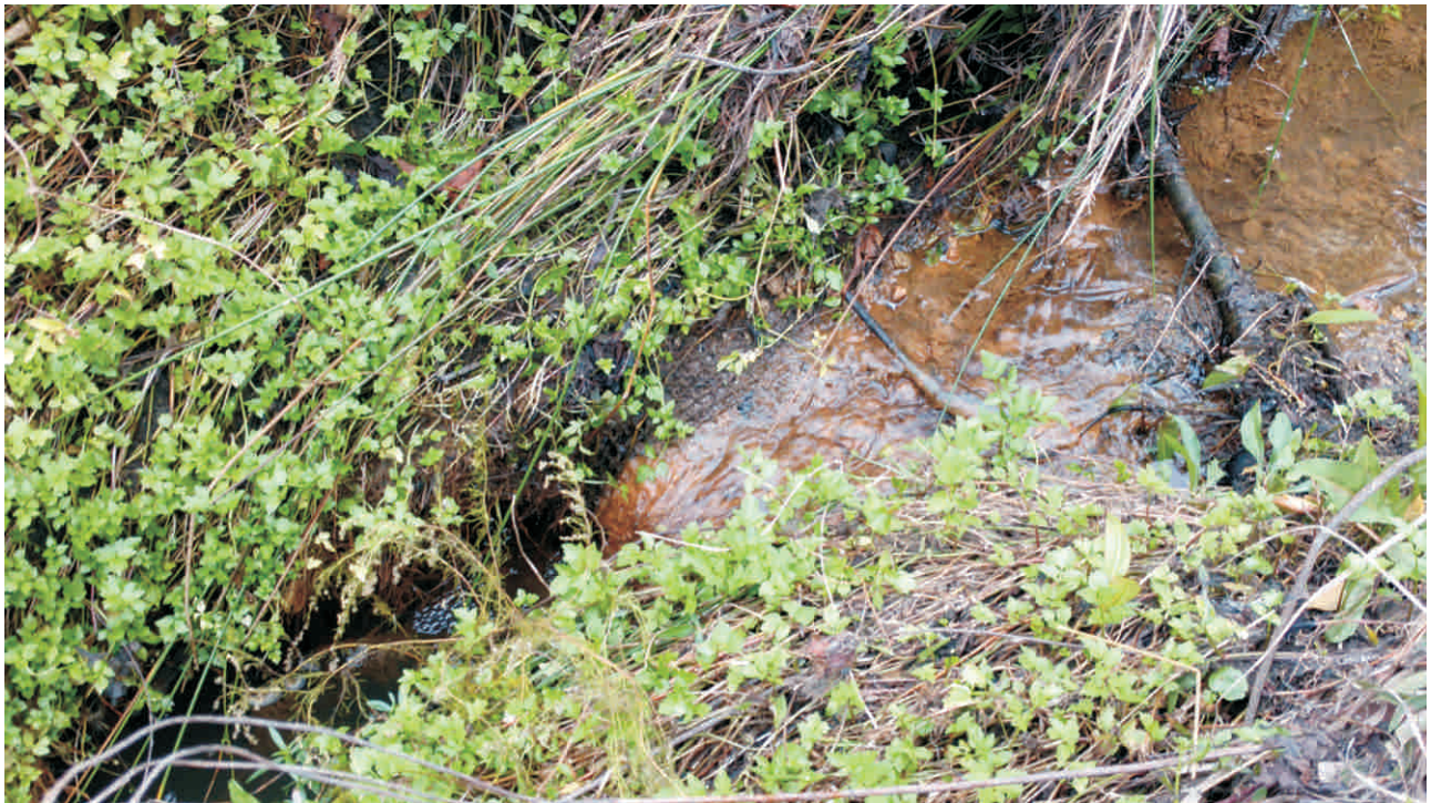
Reach 1A - Stream Problem Area 2; Undercut near Log Vane Structure
