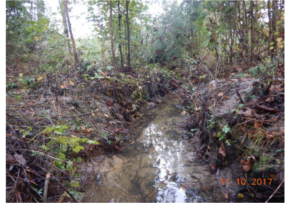
Looking downstream at CS 5 (November 2017)
