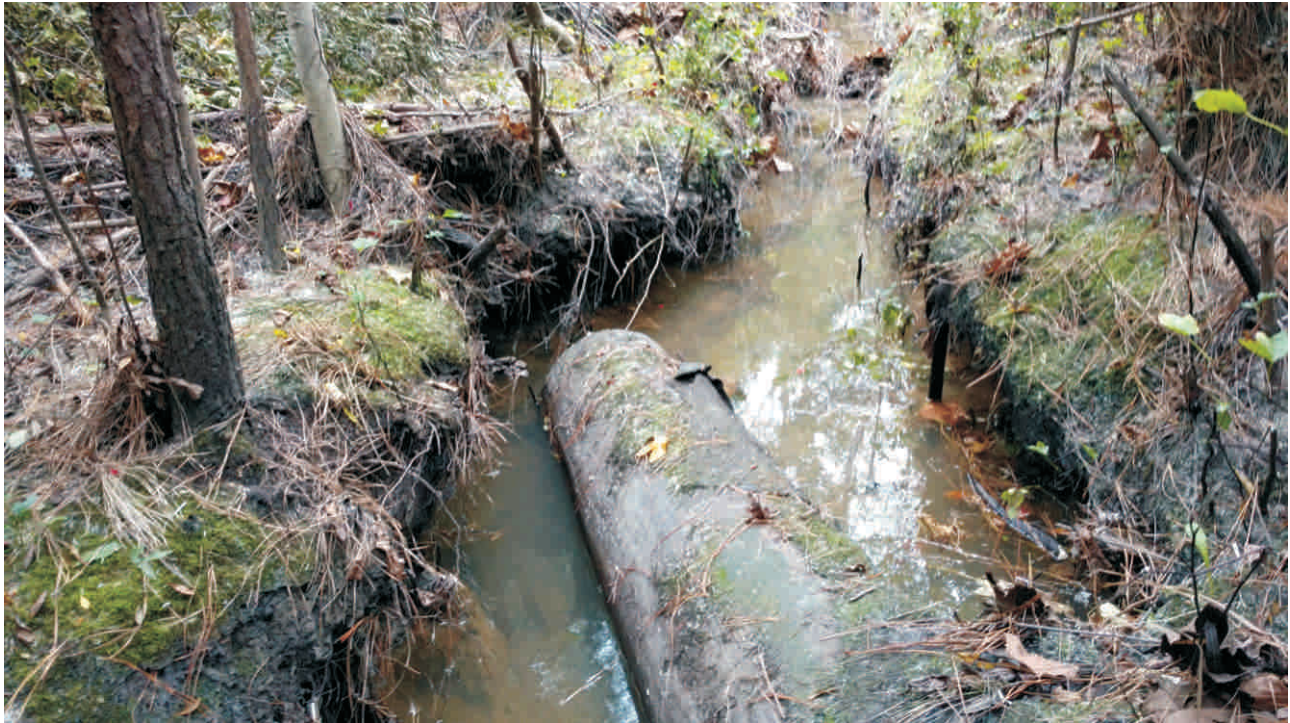
Reach 2A - Stream Problem Area #35; Log Vane Mass Wasting
