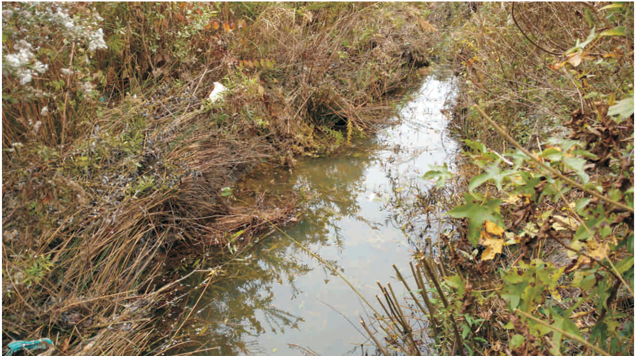
Reach 1A - Stream Problem Area #13a; Scour
