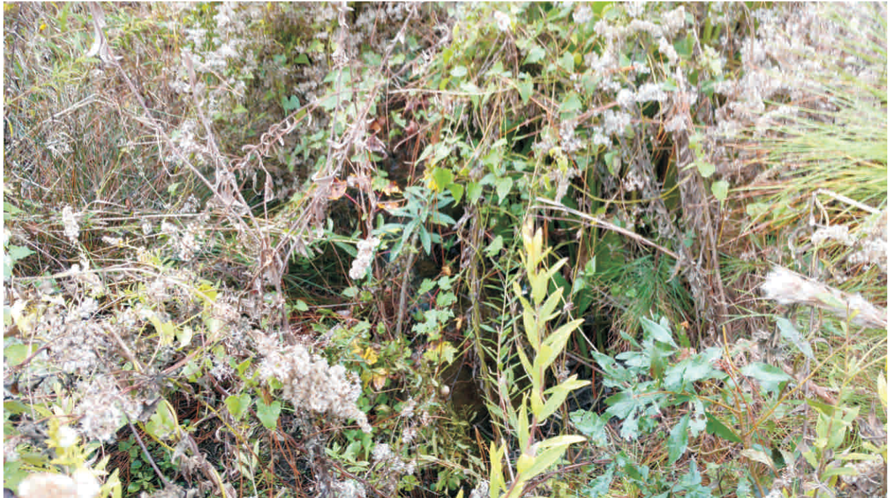
Enhancement Reach - Stream Problem Area #57c; Scour (difficult to see through vegetation)
