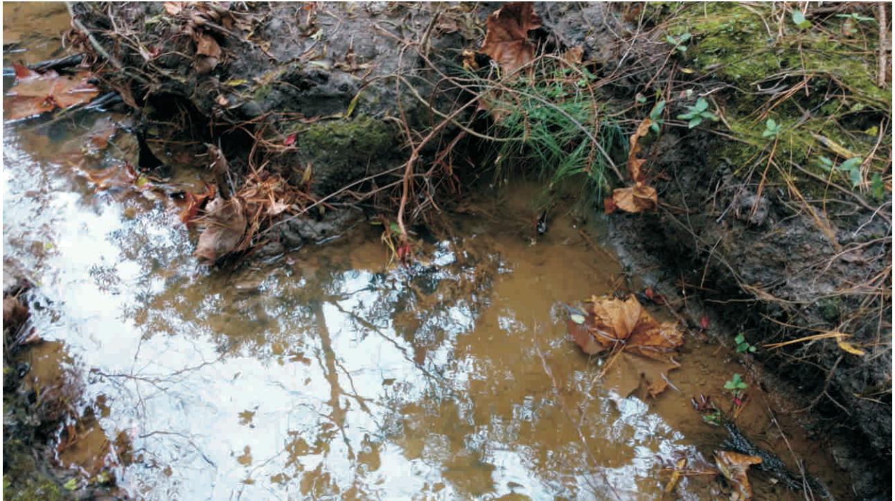
Reach 2A - Stream Problem Area #33; Scour
