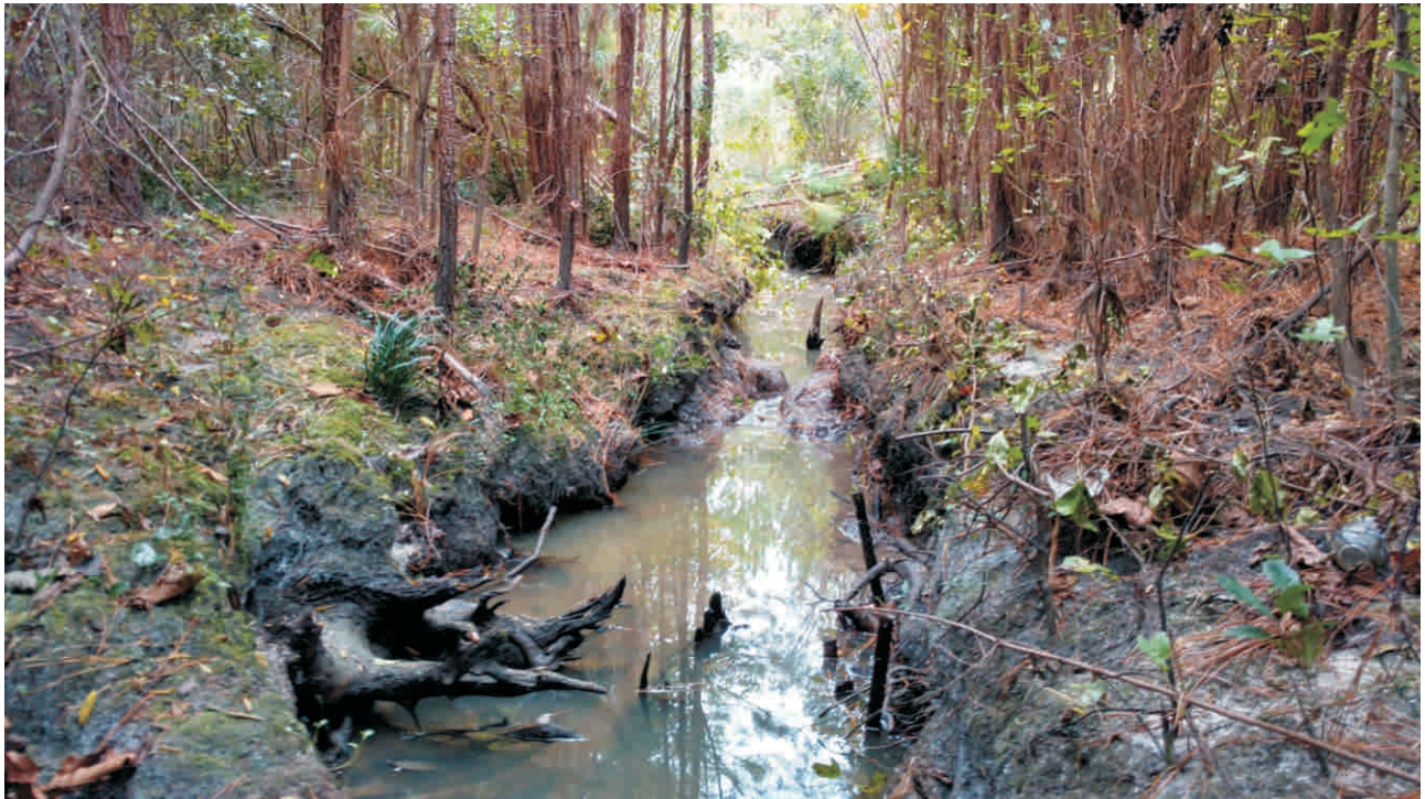
Reach 2A - Stream Problem Area #36; Degradation
