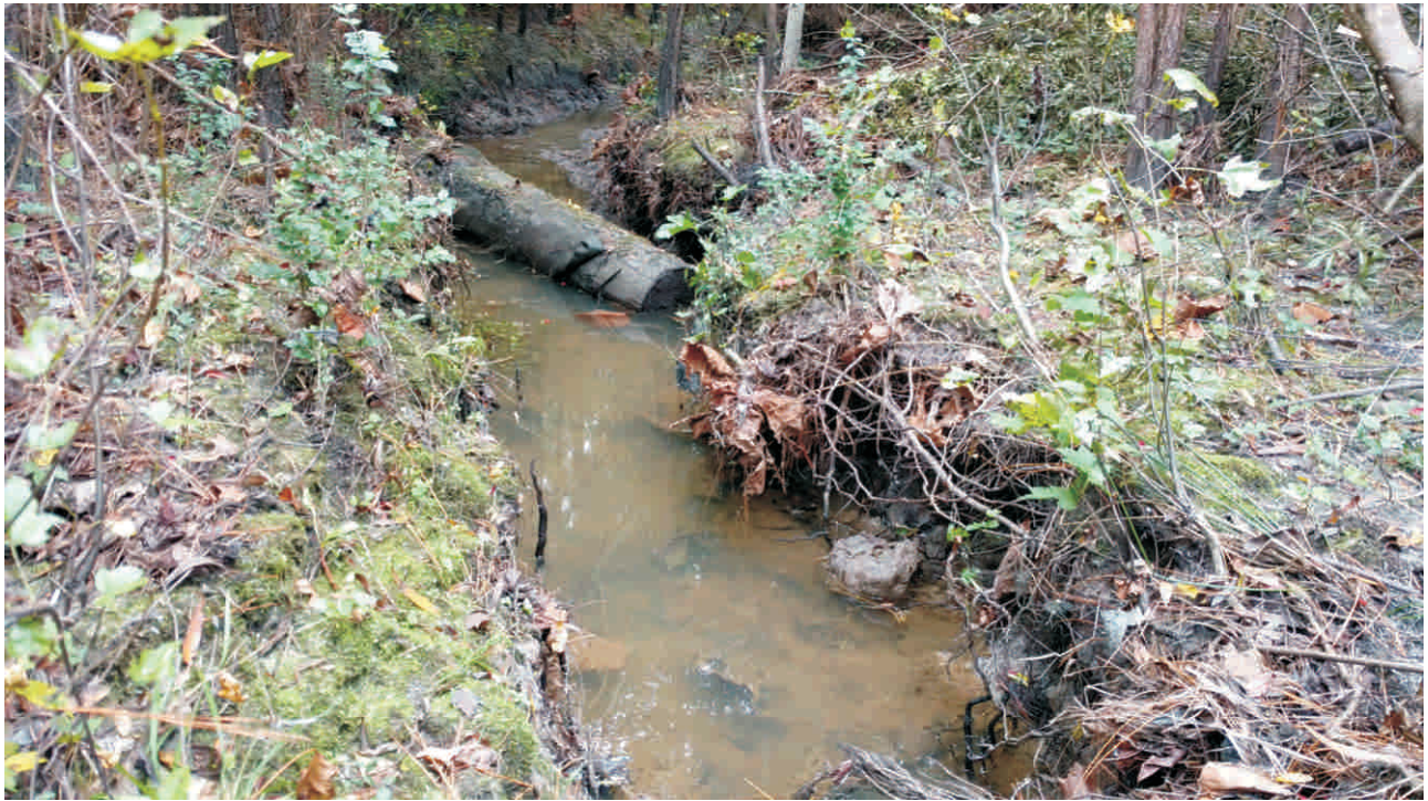
Reach 2A - Stream Problem Area #34; Log Vane Undercut
