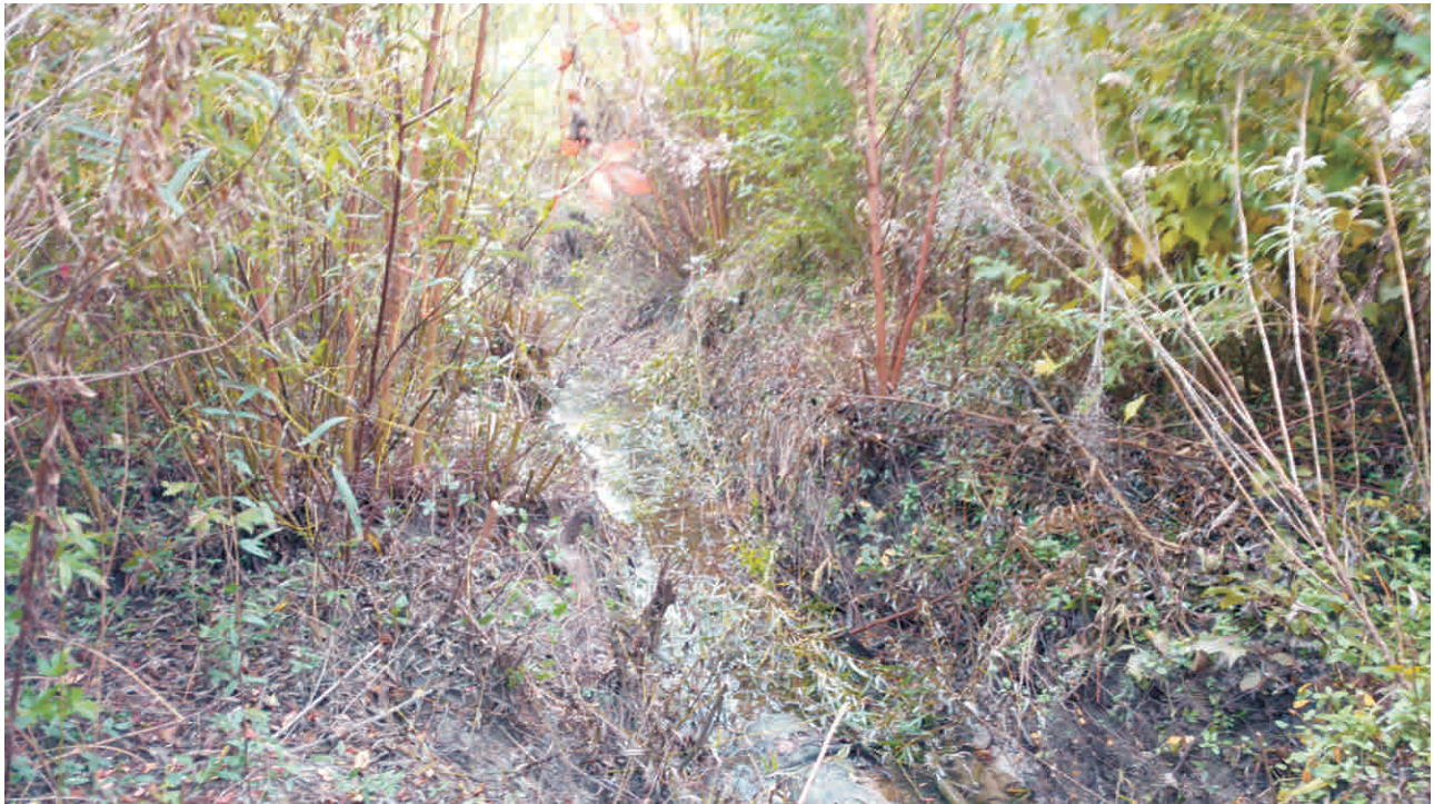
Reach 1A - Stream Problem Area #17; Degradation
