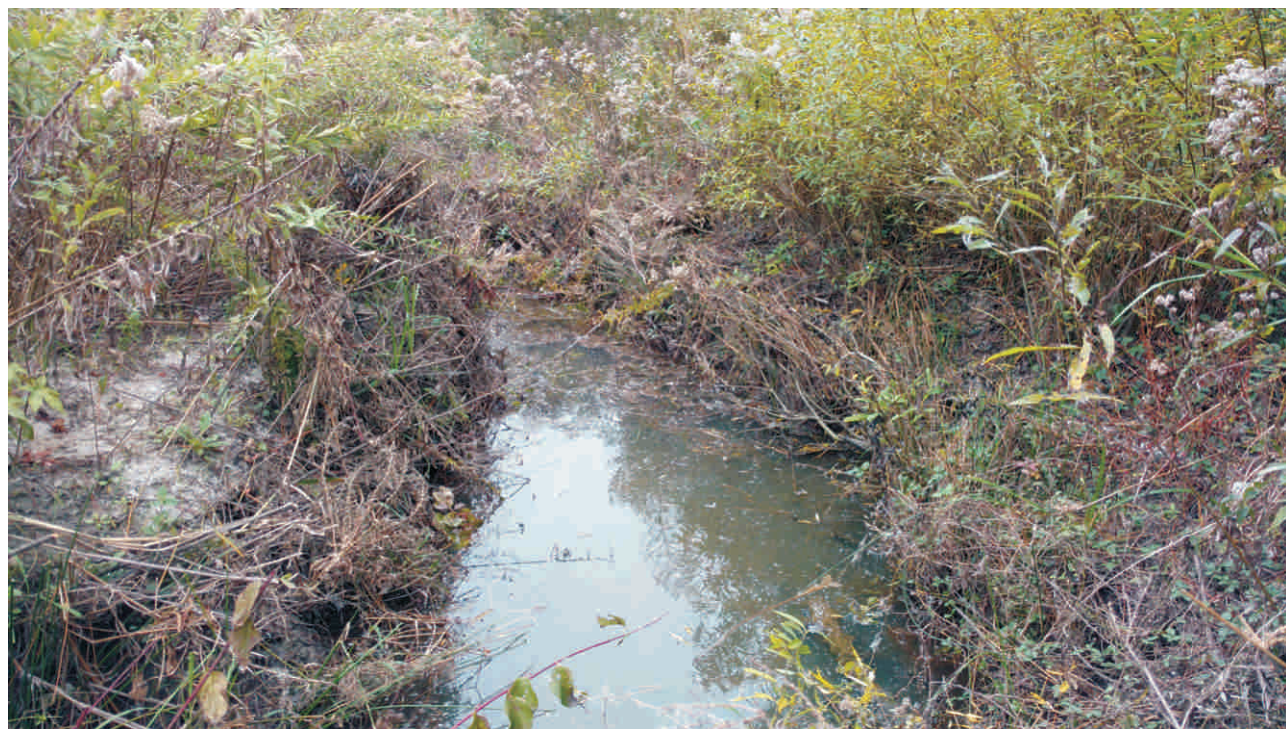
Reach 1A - Stream Problem Area #13b; Degradation
