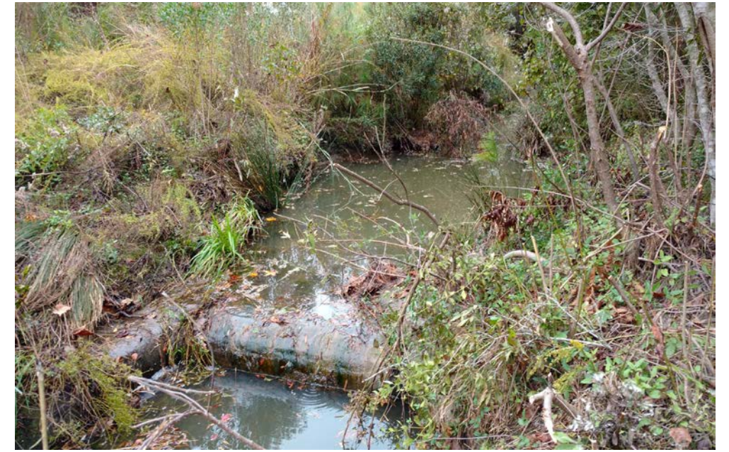
Looking downstream at CS-X3 (November 2017)
