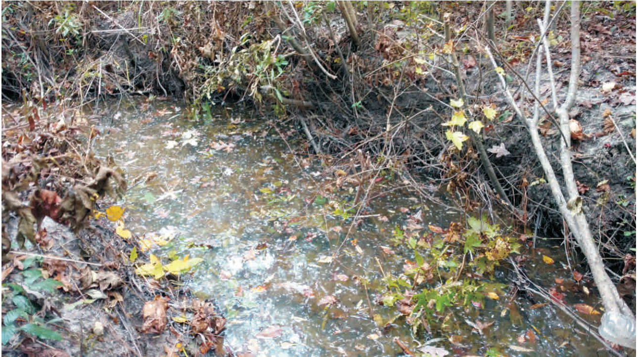
Reach B - Stream Problem Area #55; Undercut becoming Scour
