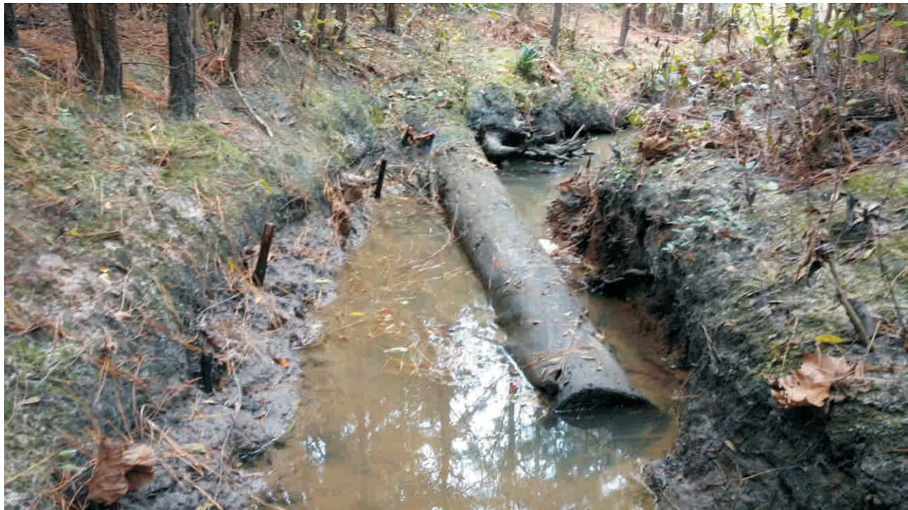
Reach 2A - Stream Problem Area #35a; Log Vane Scour
