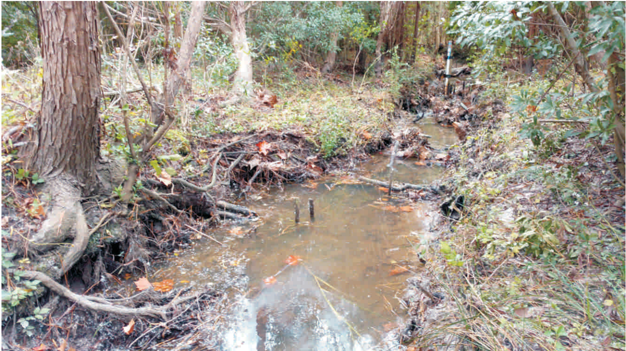
Reach 2A - Stream Problem Area #29; Scour
