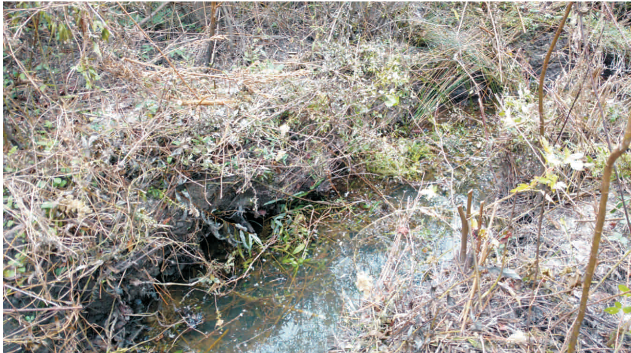
Reach 1A - Stream Problem Areas #18 & 19; Scour & Mass Wasting
