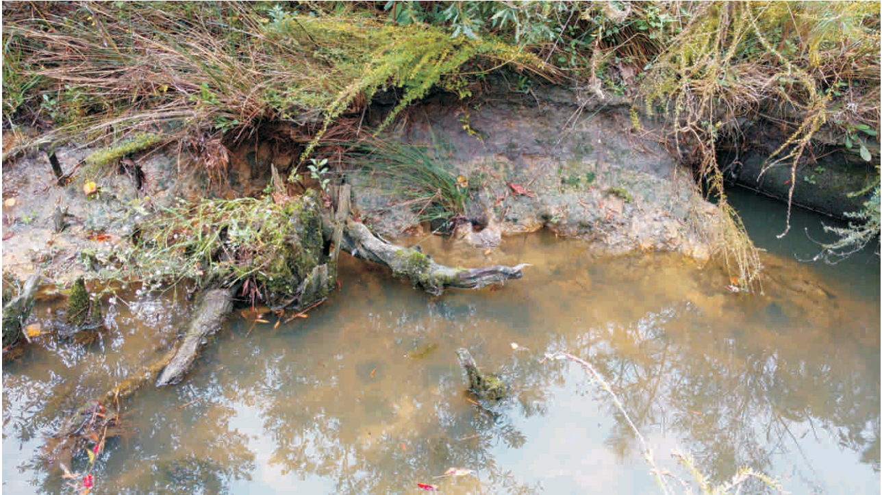
Reach 2A - Stream Problem Area #44; Scour
