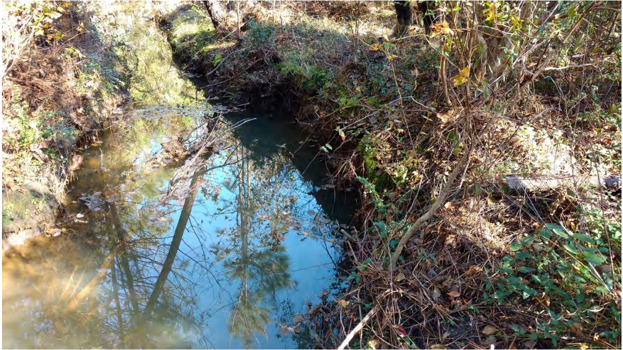
Reach 2A: Stream Problem Area 37a – Undercut
