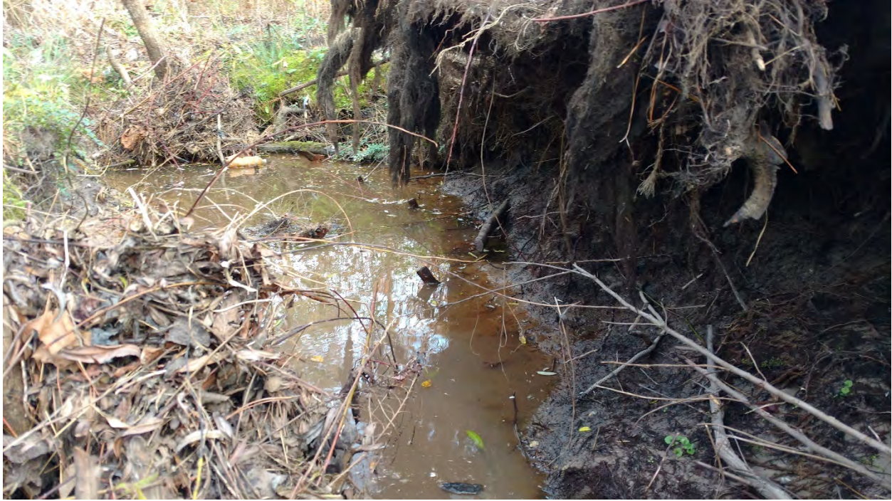
Reach 1A: Stream Problem Area 21 – Undercut
