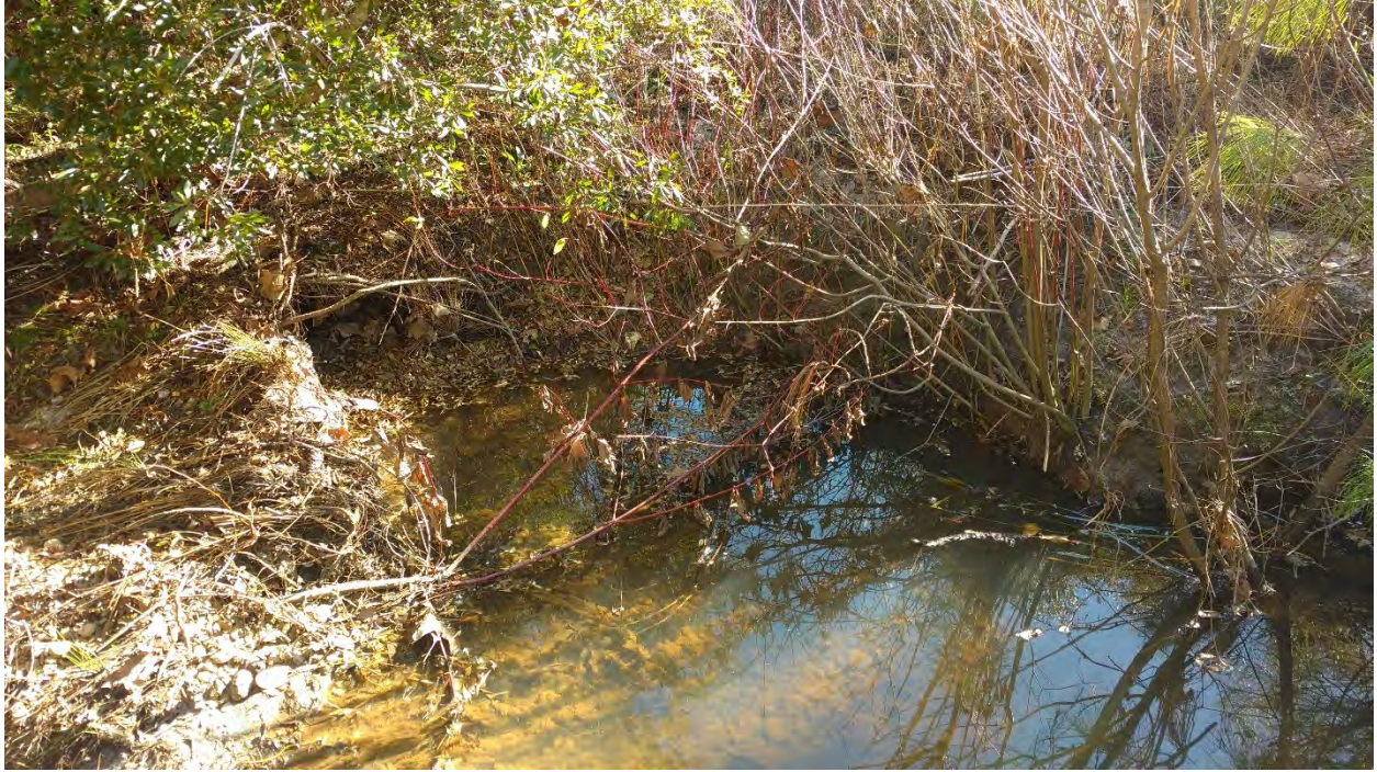
Reach 2A: Stream Problem Area 26 – Mass Wasting
