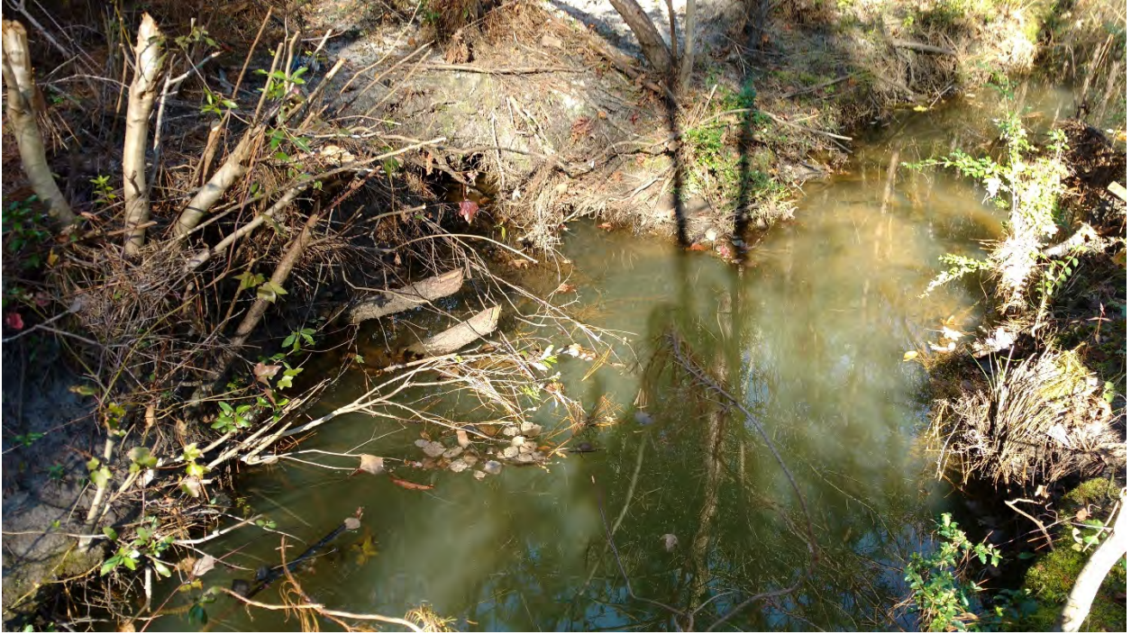
Reach 2A: Stream Problem Area 39 – Mass Wasting
