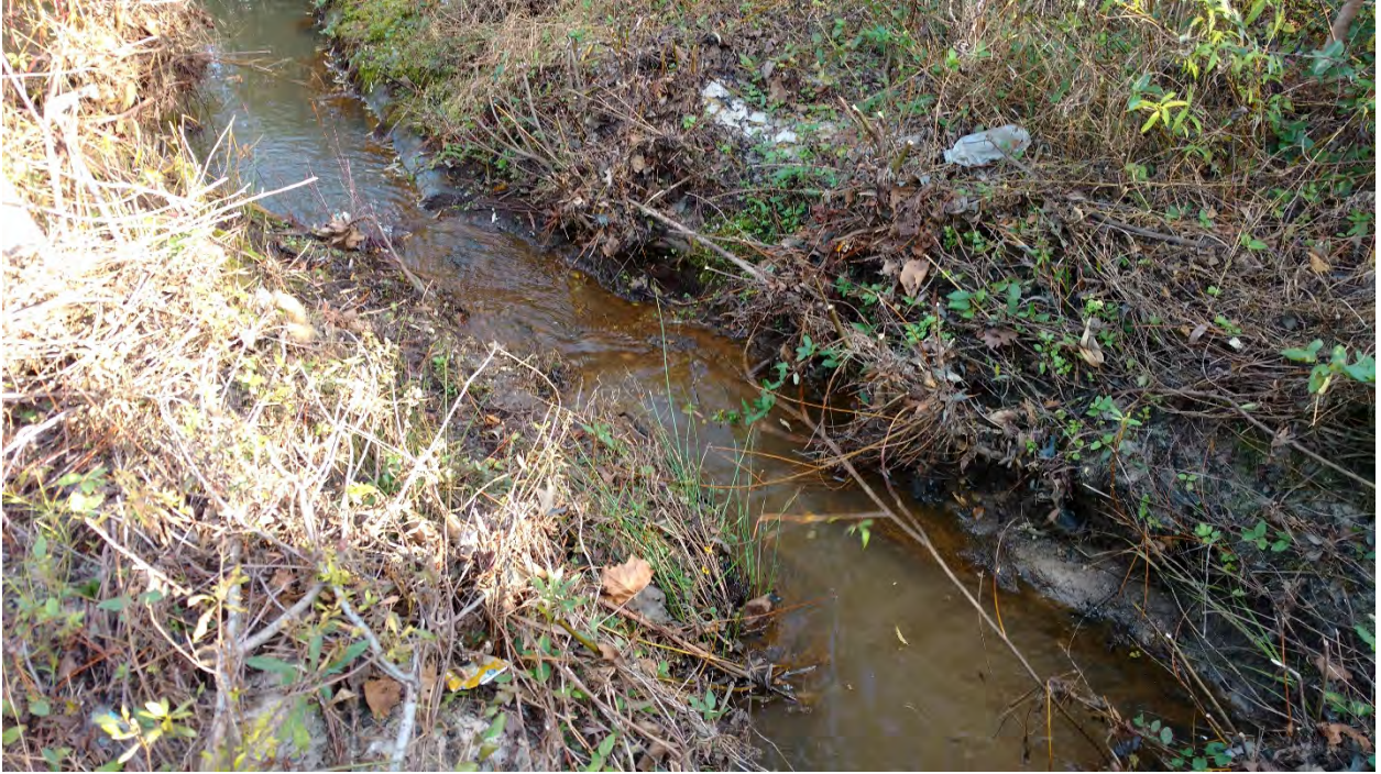
Reach 1A: Stream Problem Area 13aa – Aggradation
