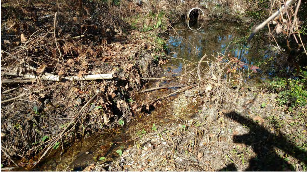
Reach C: Stream Problem Area 58 – Aggradation
