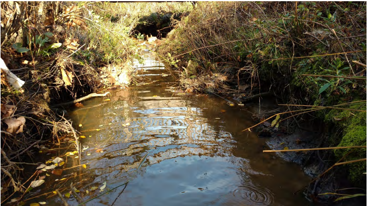
Reach 1A: Stream Problem Area 6b – Scour and Undercut
