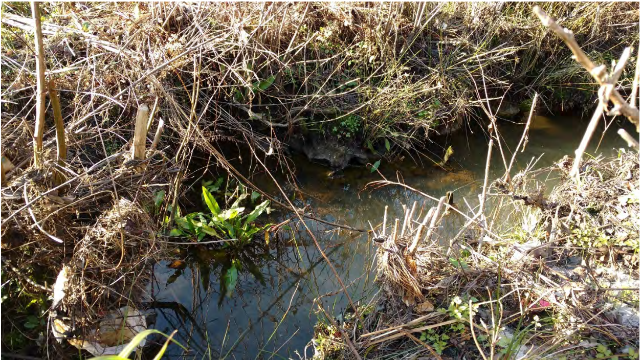
Reach 1A: Stream Problem Area 3a – Mass Wasting
