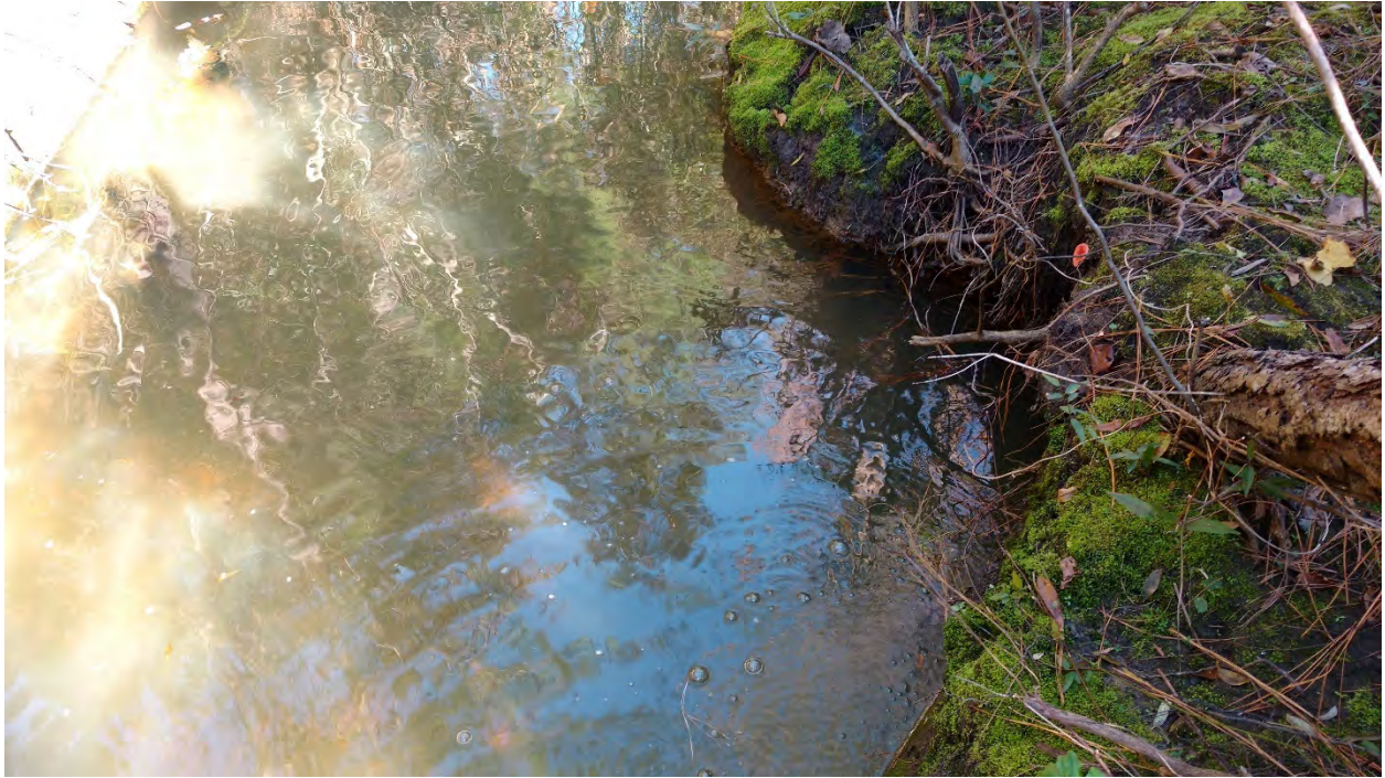
Reach 2A: Stream Problem Area 41 – Scour
