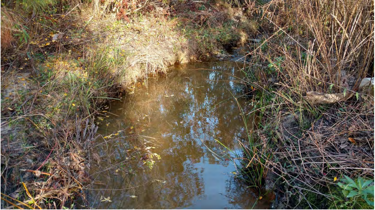
Reach 1A: Stream Problem Area 14 – Scour
