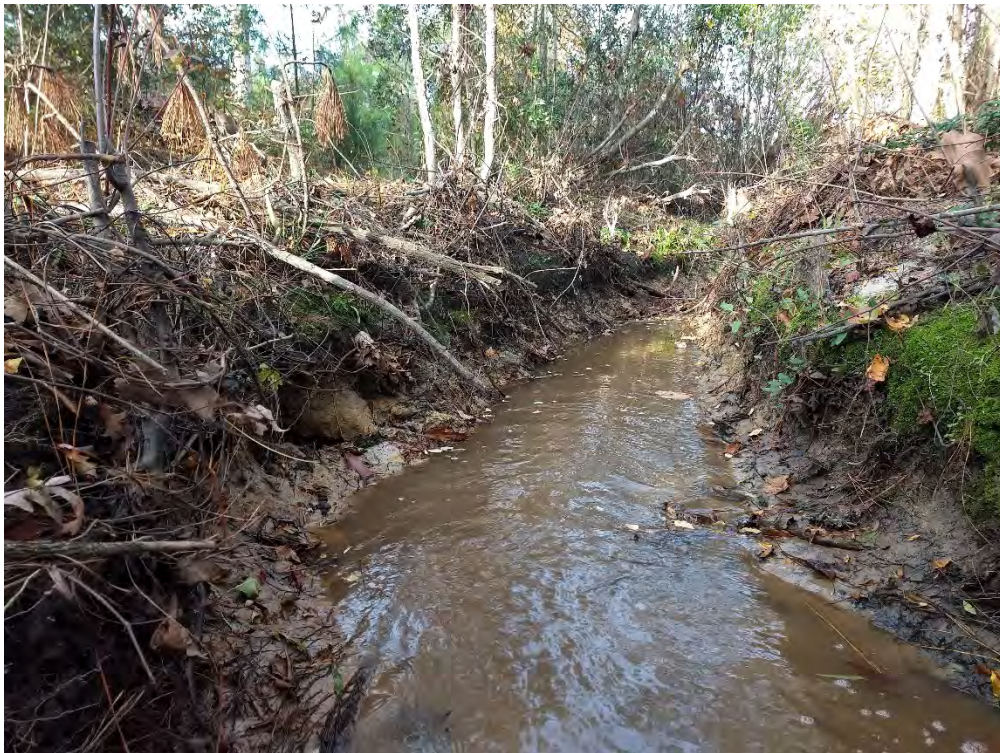
Reach 1A: Stream Problem Area 22 – Degradation
