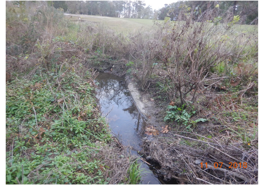
Looking downstream at CS-8 (November 2018)
