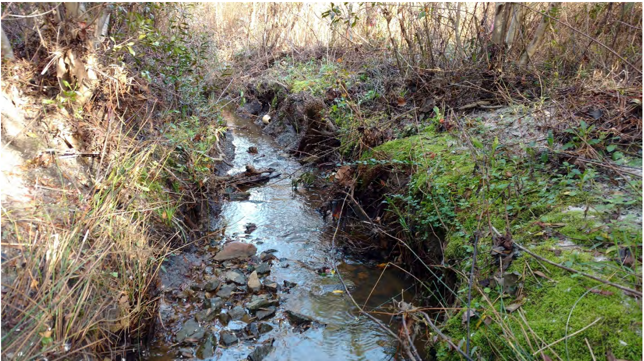
Reach 1A: Stream Problem Area 14a – Degradation
