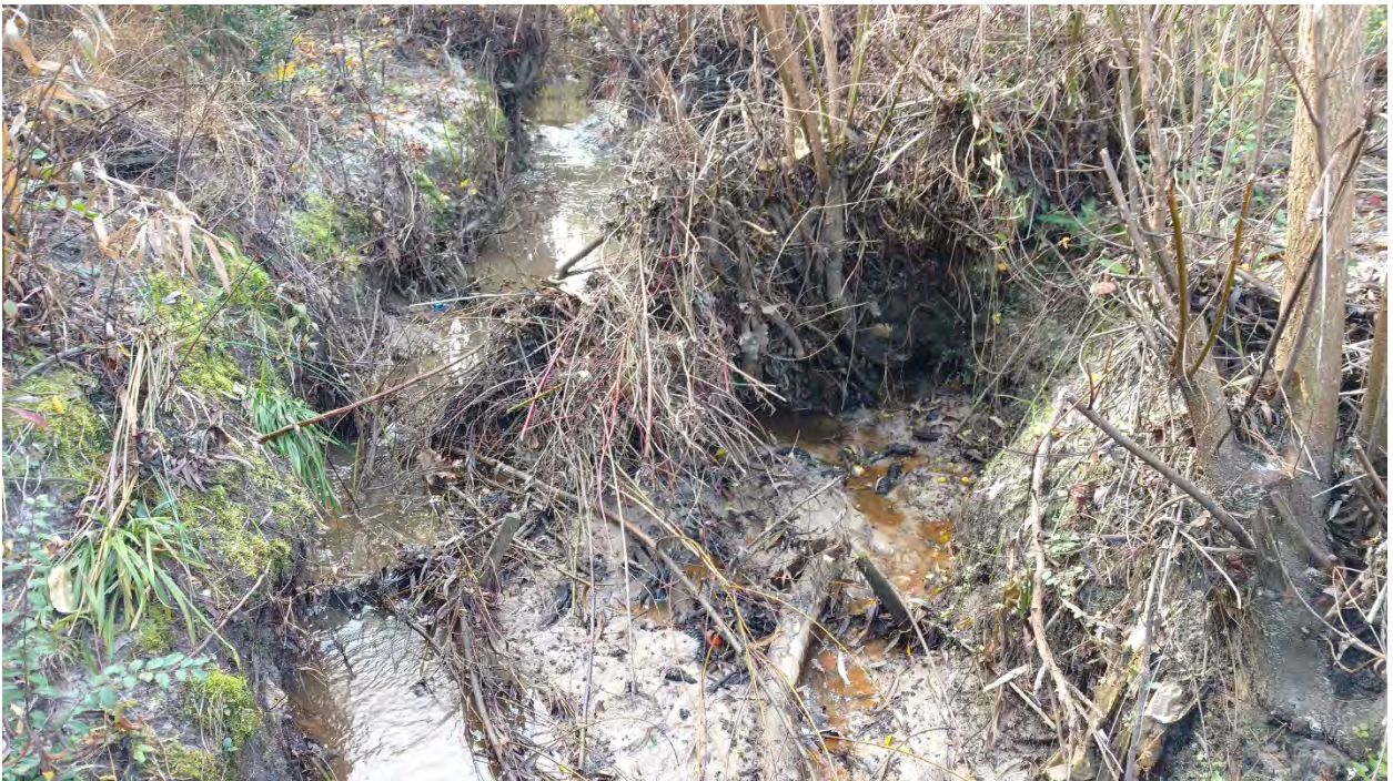
Reach 1A: Stream Problem Area 19 – Aggradation caused by Mass Wasting
