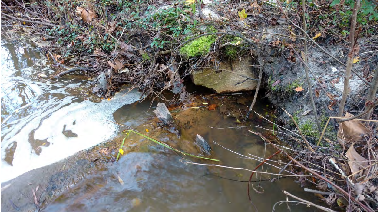
Reach 1A: Stream Problem Area 11 – Scour and Undercut
