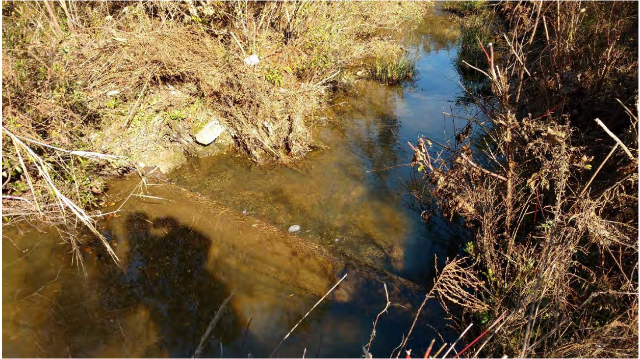
Reach 2A: Stream Problem Area 45a – Scour
