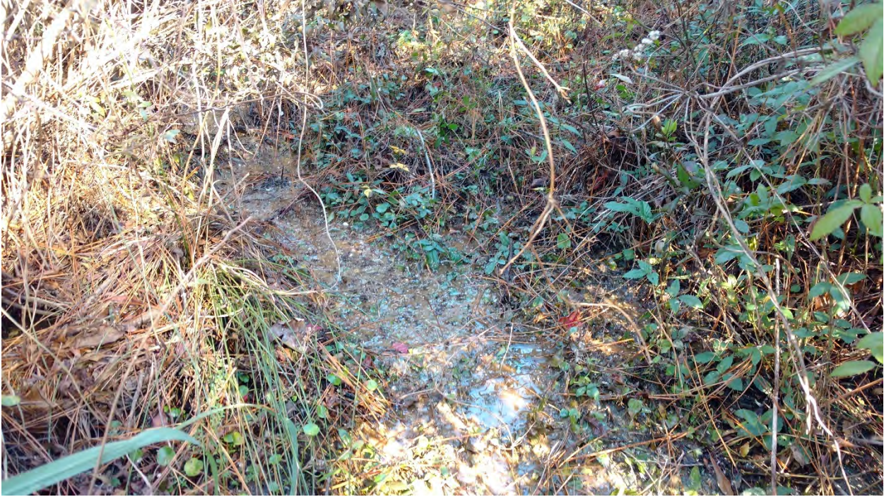
Enhancement Reach: Stream Problem Area 57 – Aggradation
