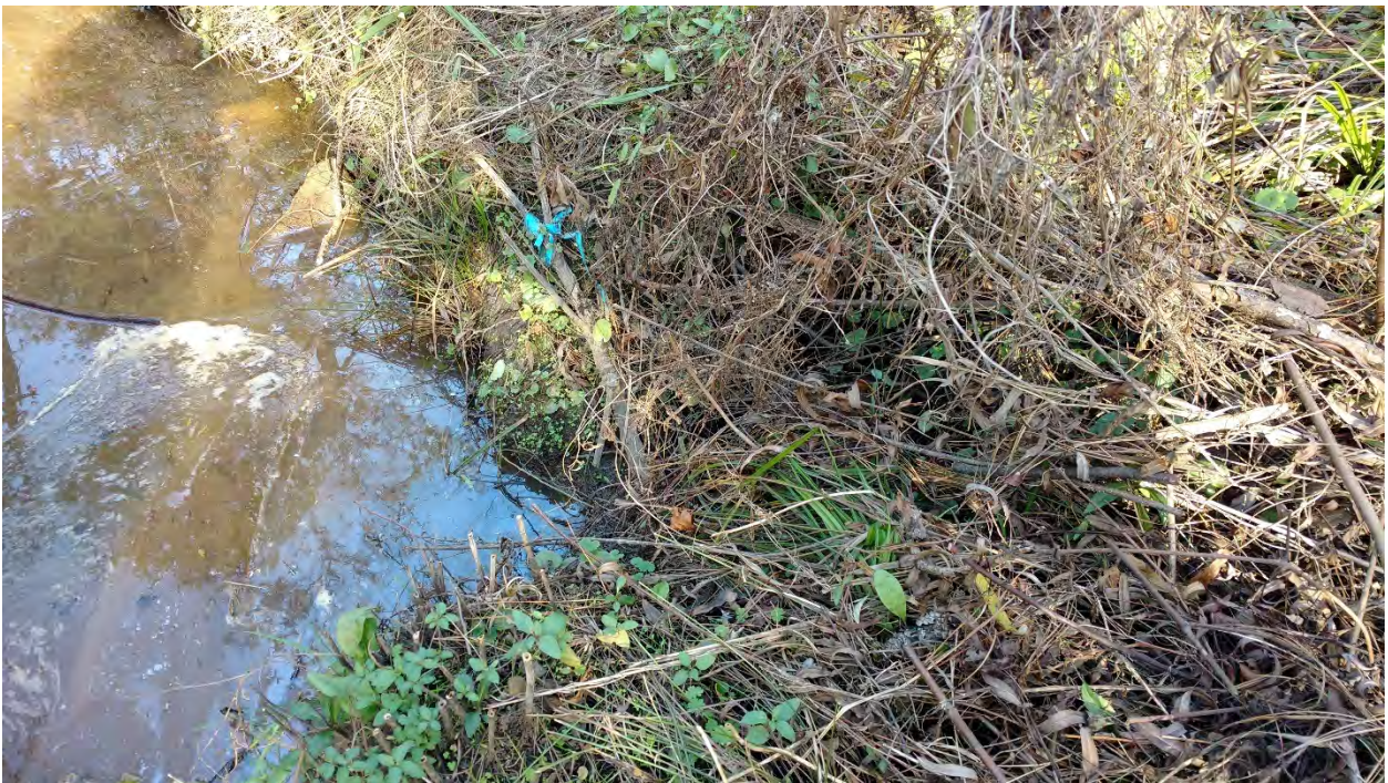
Reach B: Stream Problem Area 52 – Mass Wasting
