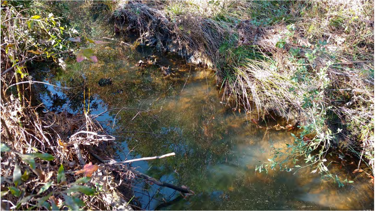
Reach 2A: Stream Problem Area 43 – Degradation
