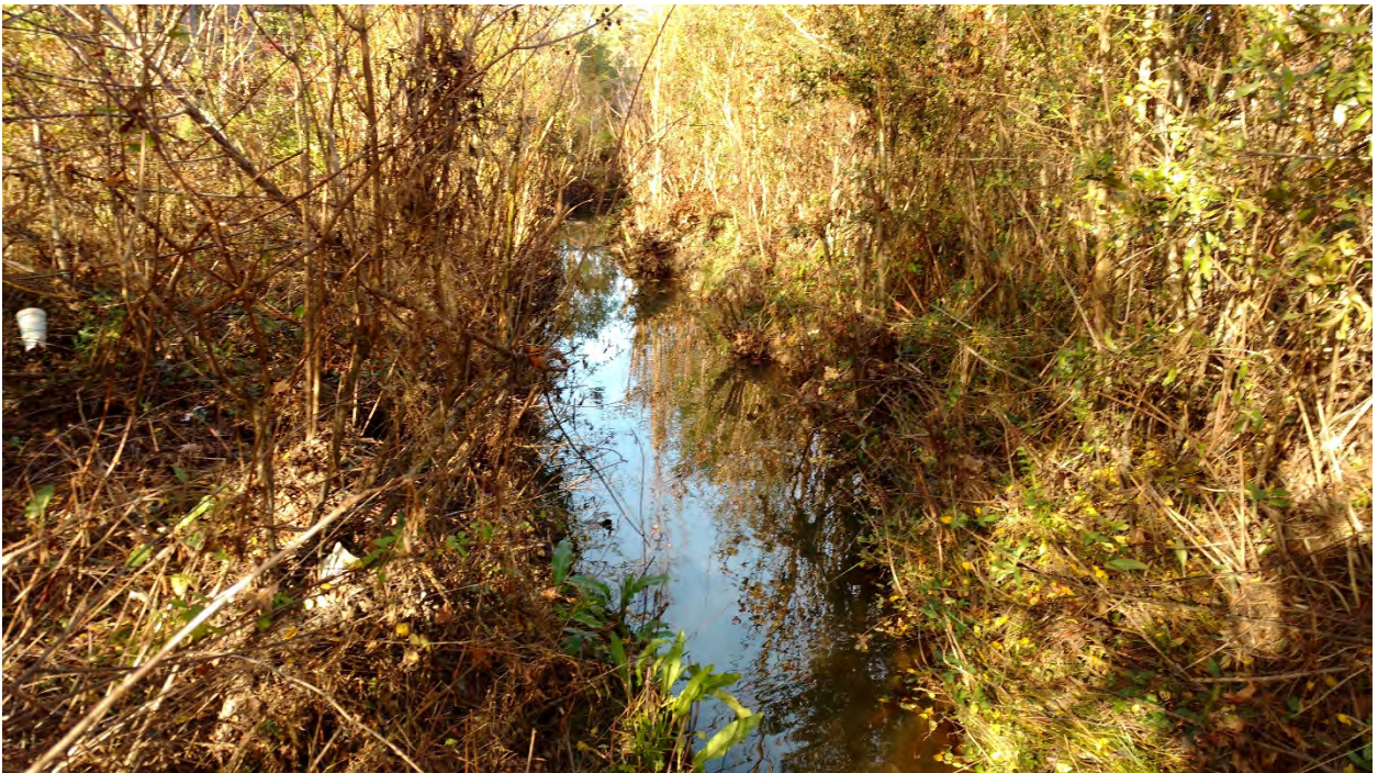
Reach 1A: Stream Problem Area 8 – Degradation
