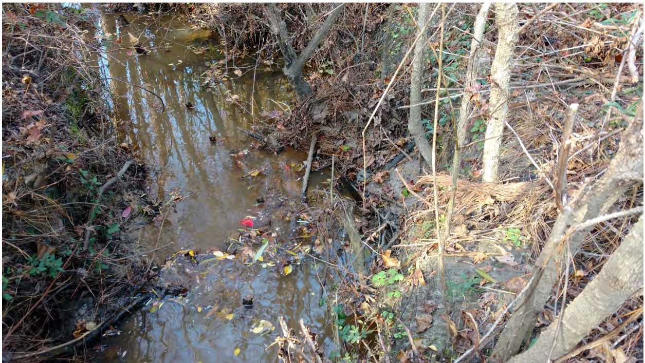
Reach B: Stream Problem Area 55 – Scour
