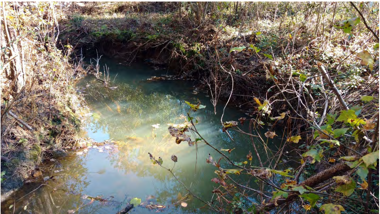
Reach 2A: Stream Problem Area 37 – Mass Wasting
