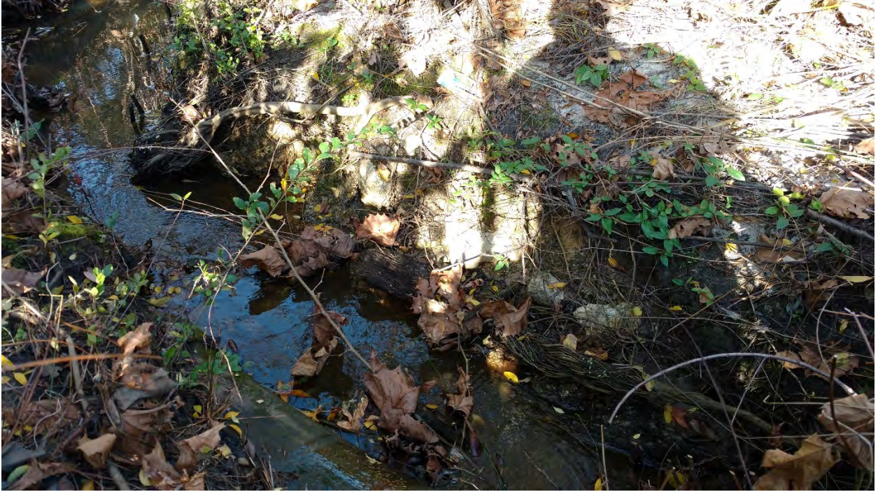
Reach 1A: Stream Problem Area 6a – Scour
