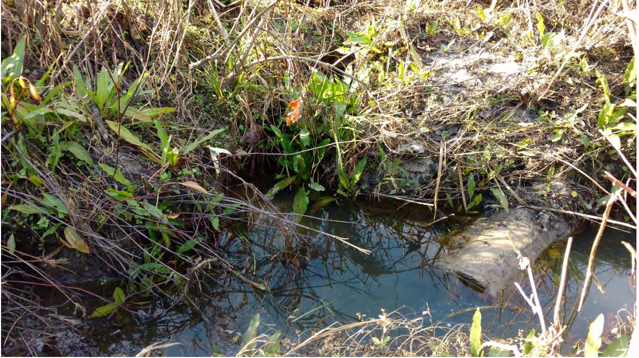
Reach 1A: Stream Problem Area 3 – Mass Wasting where channels come together
