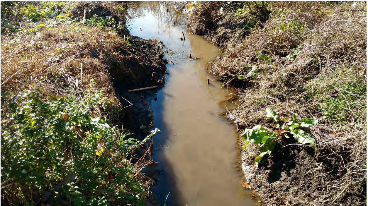
Reach C: Stream Problem Area 61 – Degradation
