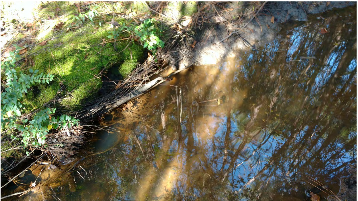
Reach 2A: Stream Problem Area 35a – Scour
