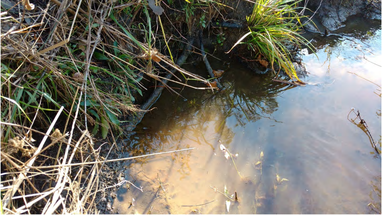
Reach C: Stream Problem Area 60 – Scour
