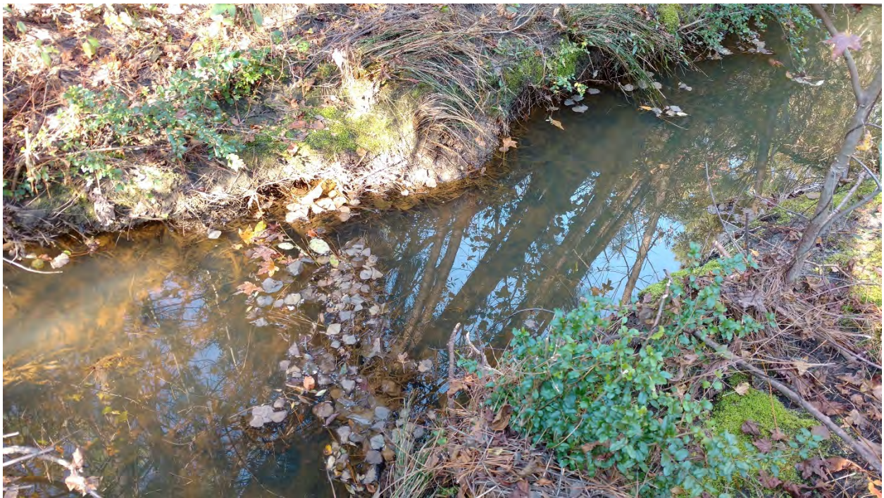
Reach 2A: Stream Problem Area 38 – Degradation
