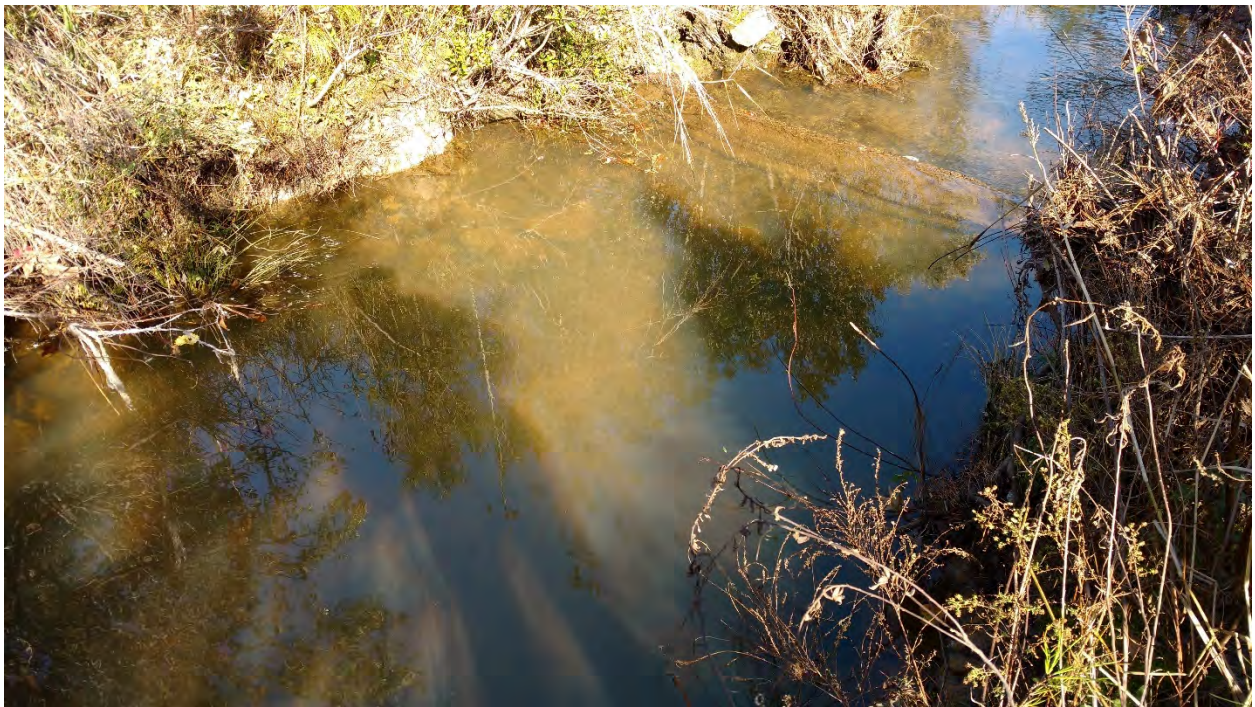
Reach 2A: Stream Problem Area 45 – Scour
