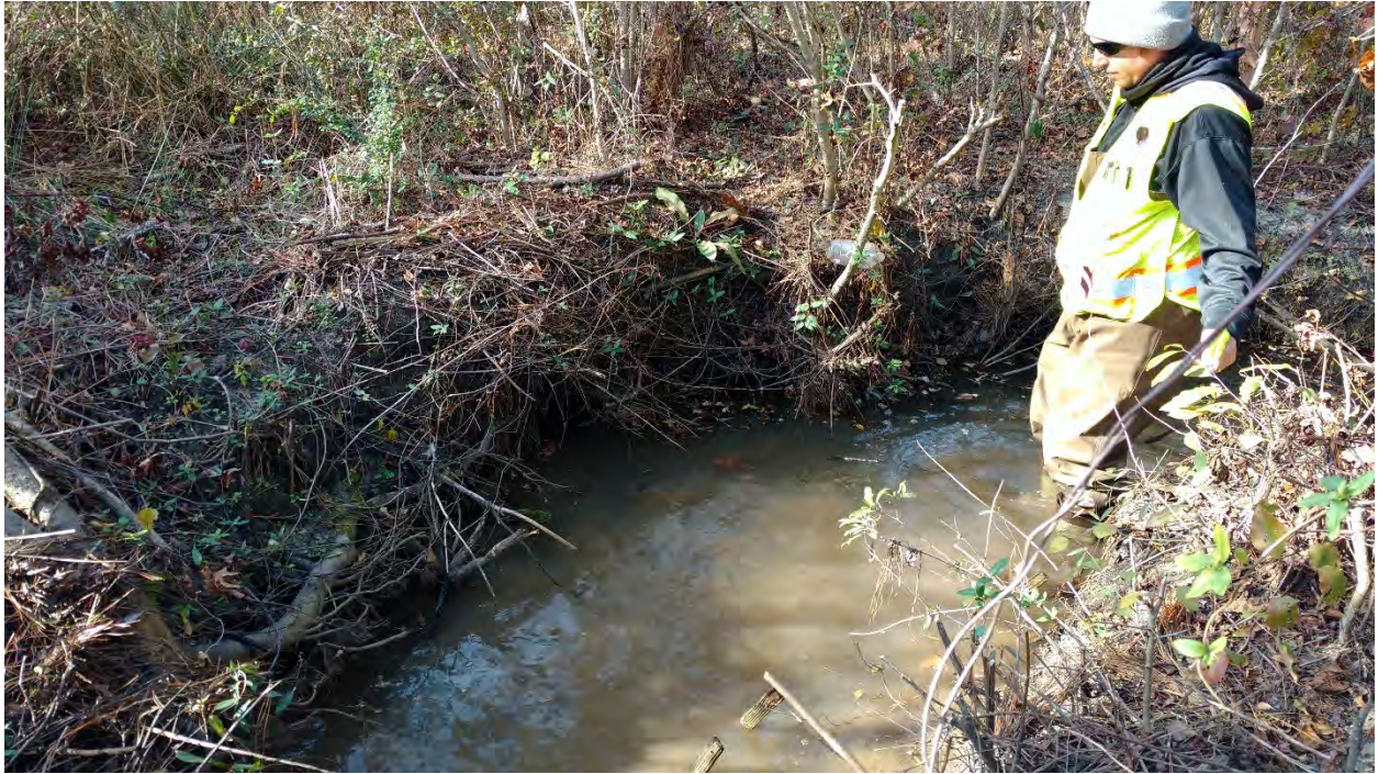
Reach B: Stream Problem Area 54 – Under Cut
