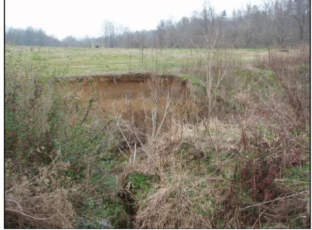
Looking at an eroded bank on T2-2. 2/10/2012
