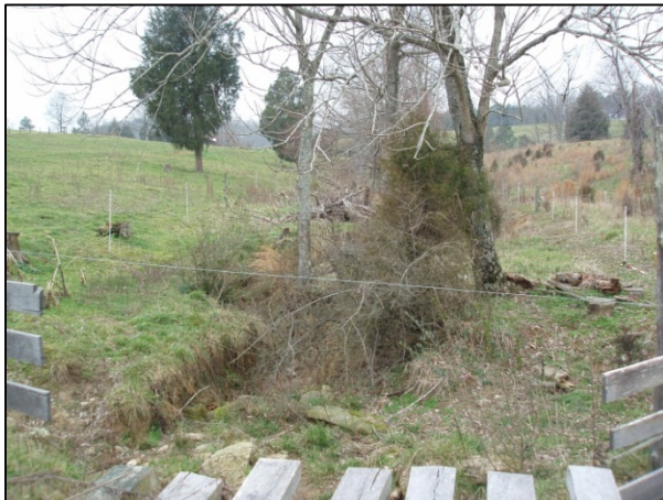
Looking downstream at the start of T1A-1. 2/10/2012
