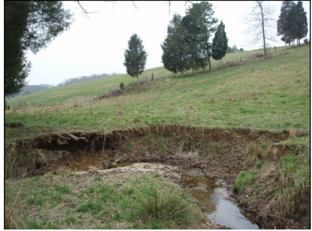
Looking downstream at degraded bank on T1-1. 2/10/2012
