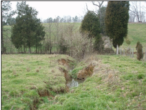
Looking downstream at the head cut section of T1A-3. 2/10/2012
