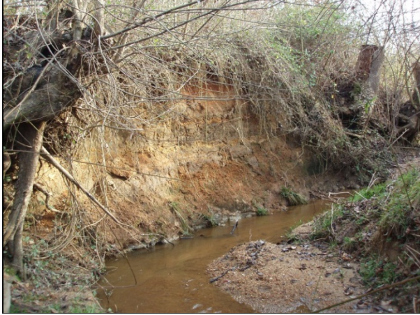
Looking downstream at eroded bank on T2-2. 2/10/2012
