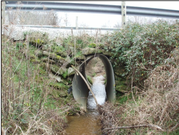
Looking downstream at culvert at the end of reach T2-2. 2/10/2012
