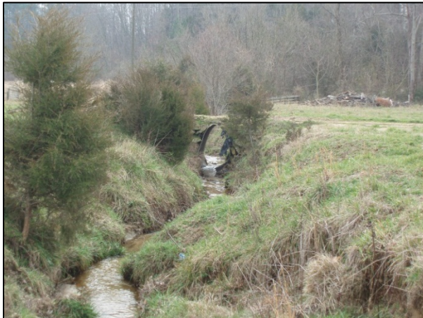
Looking downstream at culvert on T1-2. 2/10/2012
