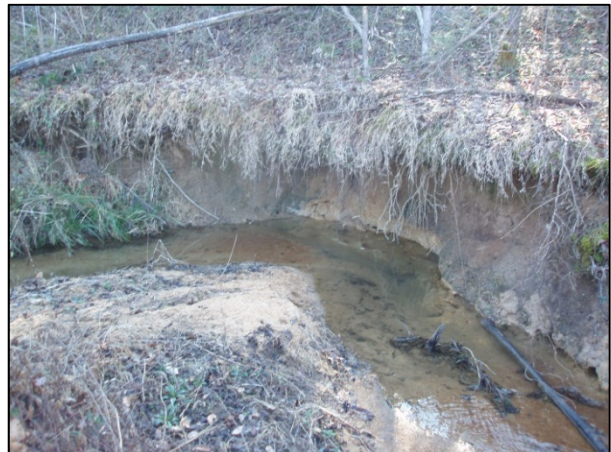
Looking at an eroded bank on T2-1. 2/10/2012
