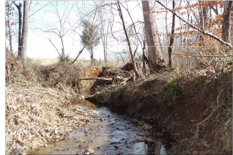
Jacob's Landing Stream Restoration Site XS6
