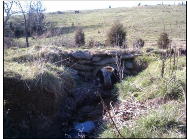
Looking downstream at a culvert on T2-1. 2/15/2012
