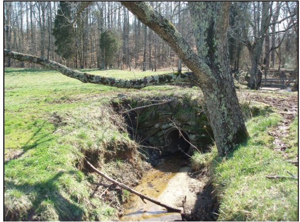
Looking downstream at the culvert on T1-3. 2/21/2012
