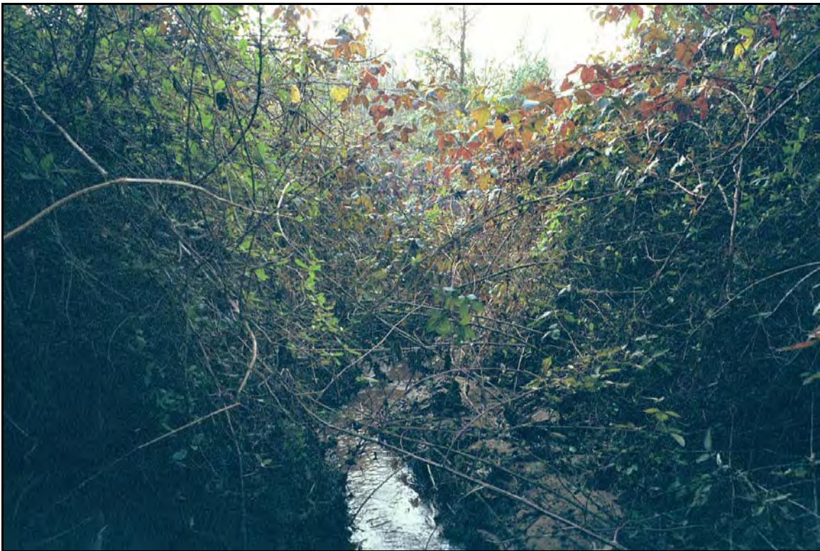
Photograph 18 – Typical view downstream of the pipe (approximately Station 24+00). Banks are greater than six feet high.
