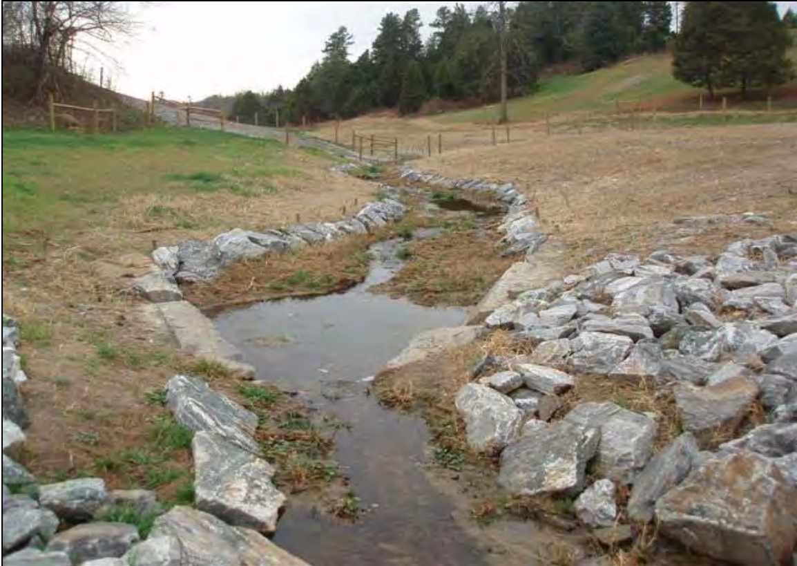
Photo Point 2b: View looking downstream taken at Station 10+00. 12/13/07 – As-Built
