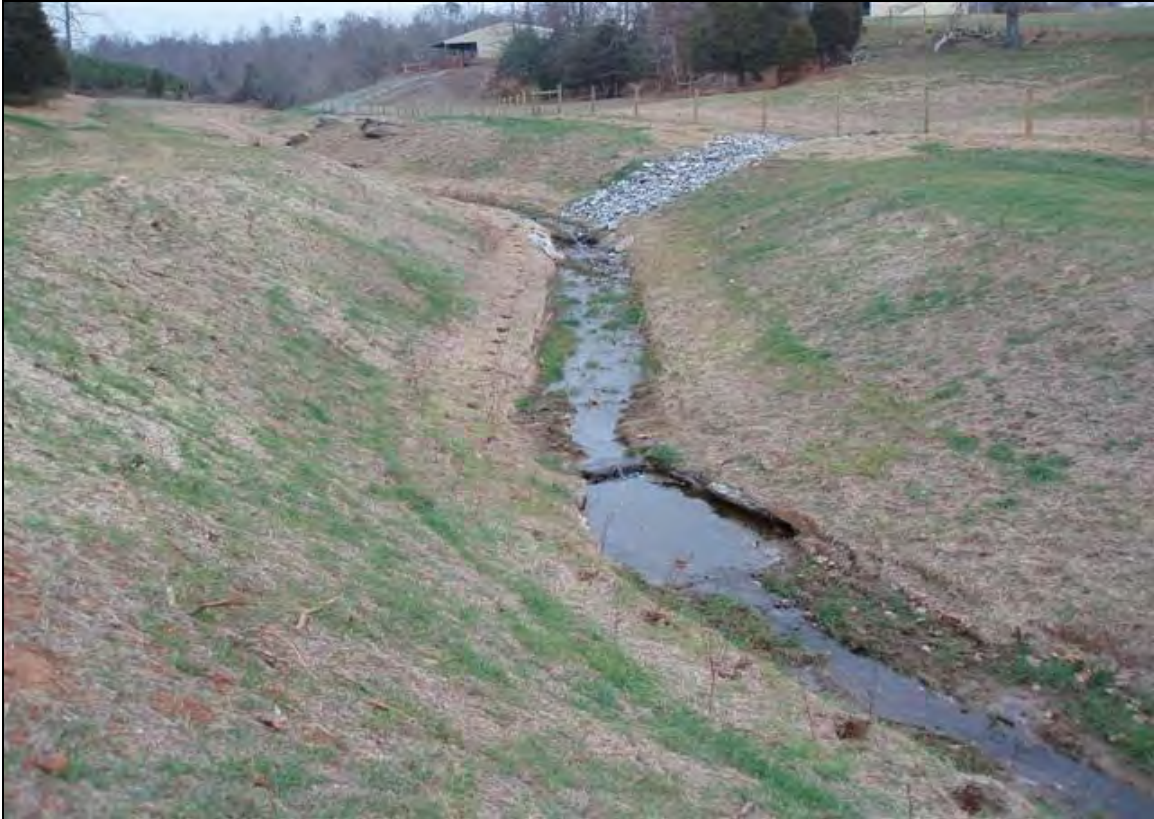
Photo Point 7a: View looking upstream taken near Station 17+80. 12/13/07 – As-Built
