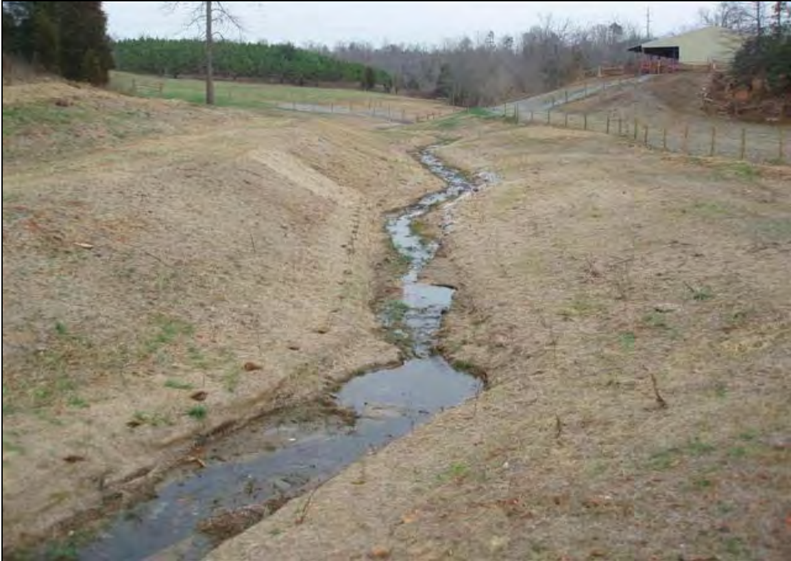
Photo Point 6a: View looking upstream taken near Station 15+75. 12/13/07 – As-Built
