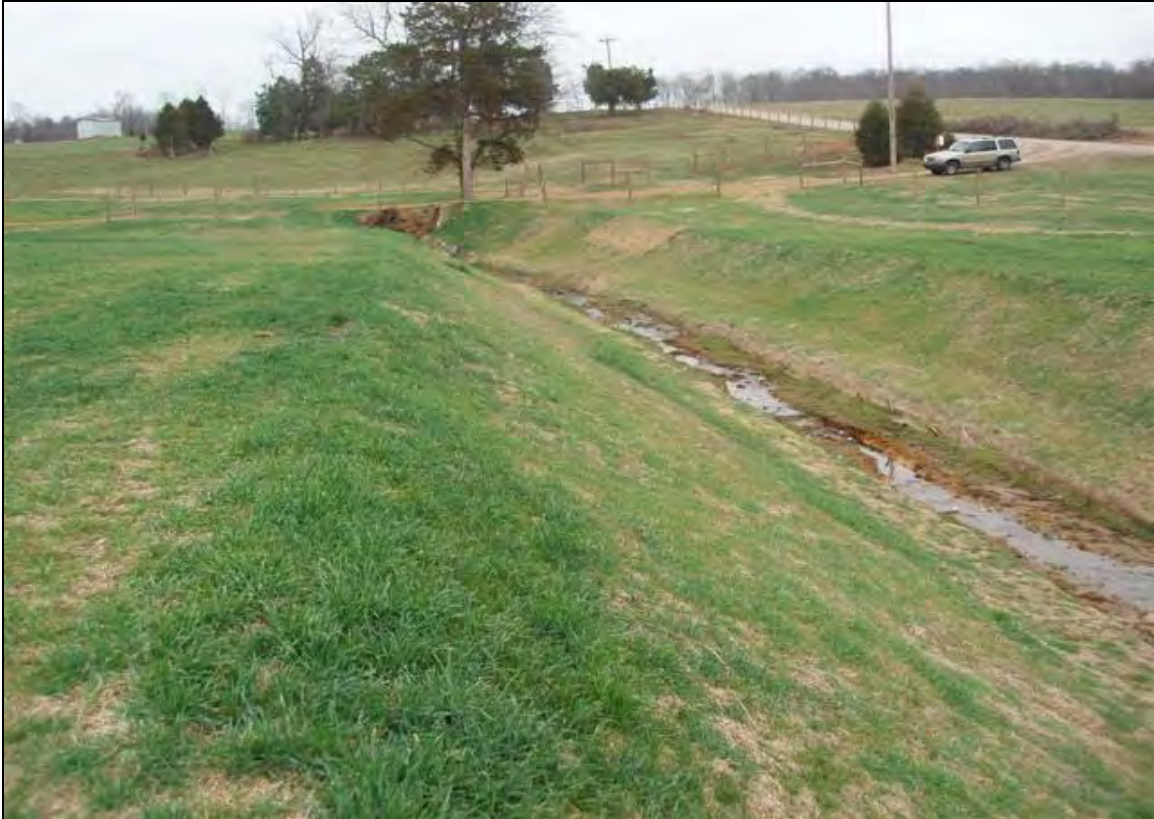
Photo Point 10a: View looking upstream taken near Station 25+00. 12/13/07 – As-Built
