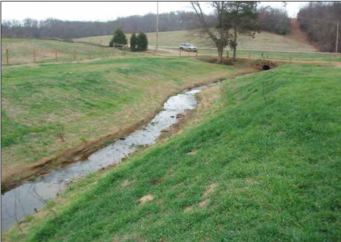
Photo Point 8b: View looking downstream taken near Station 20+75. 12/13/07 – As-Built
