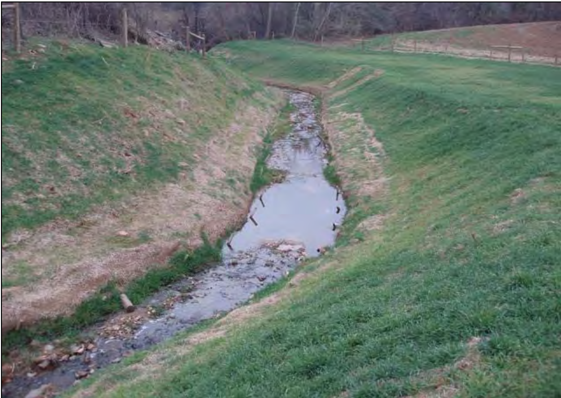
Photo Point 11b: View looking downstream taken near Station 27+65. 12/13/07 – As-Built
