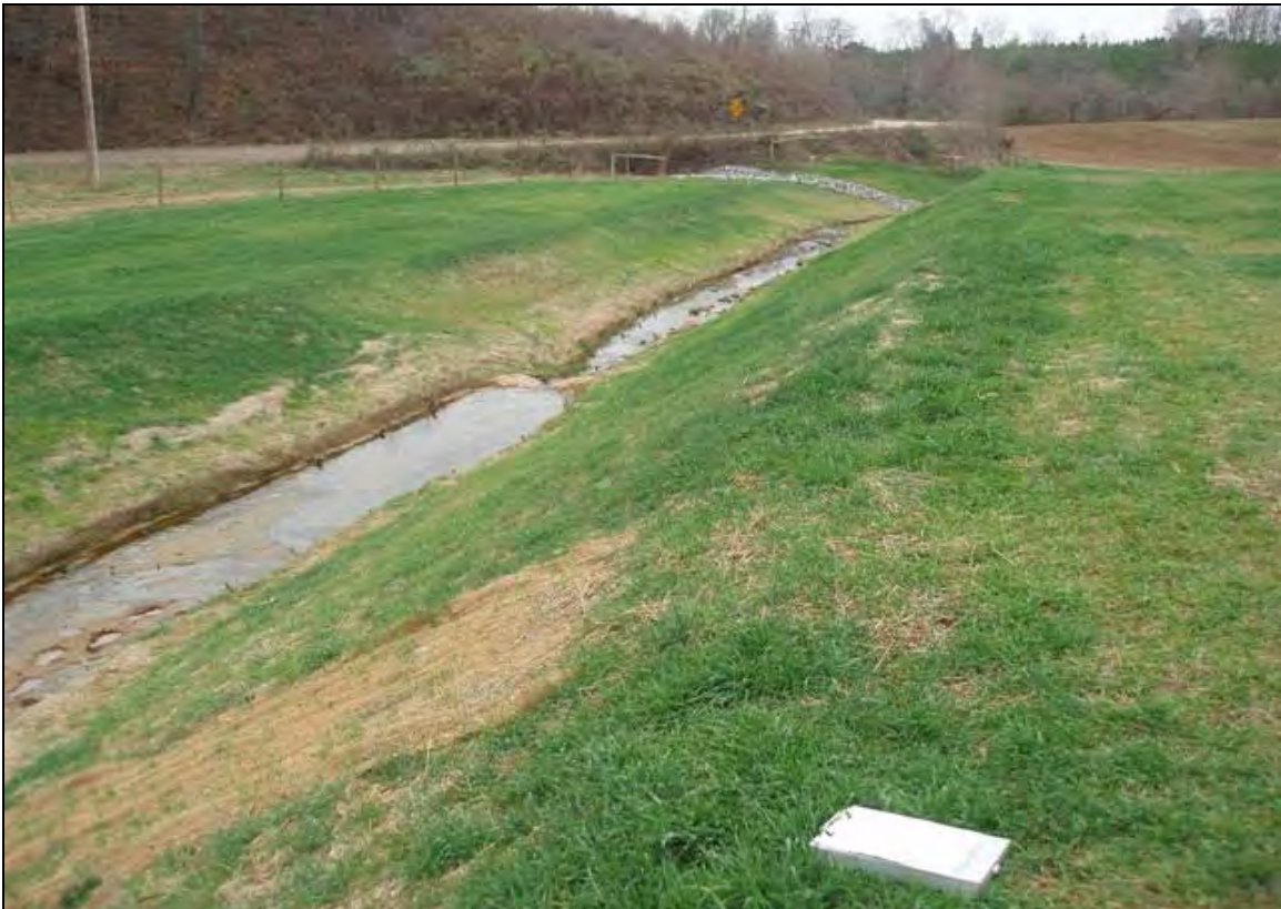
Photo Point 10b: View looking downstream taken near Station 25+00. 12/13/07 – As-Built
