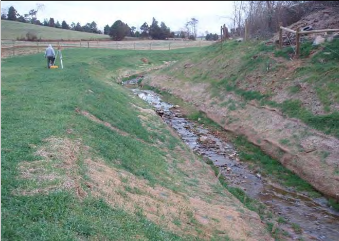
Photo Point 12a: View looking upstream taken near Station 30+25. 12/13/07 – As-Built
