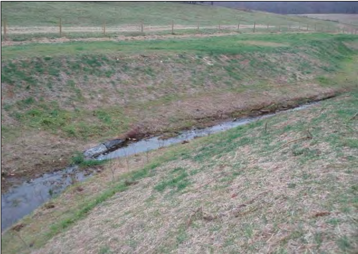
Photo Point 7b: View looking downstream taken near Station 17+80. 12/13/07 – As-Built
