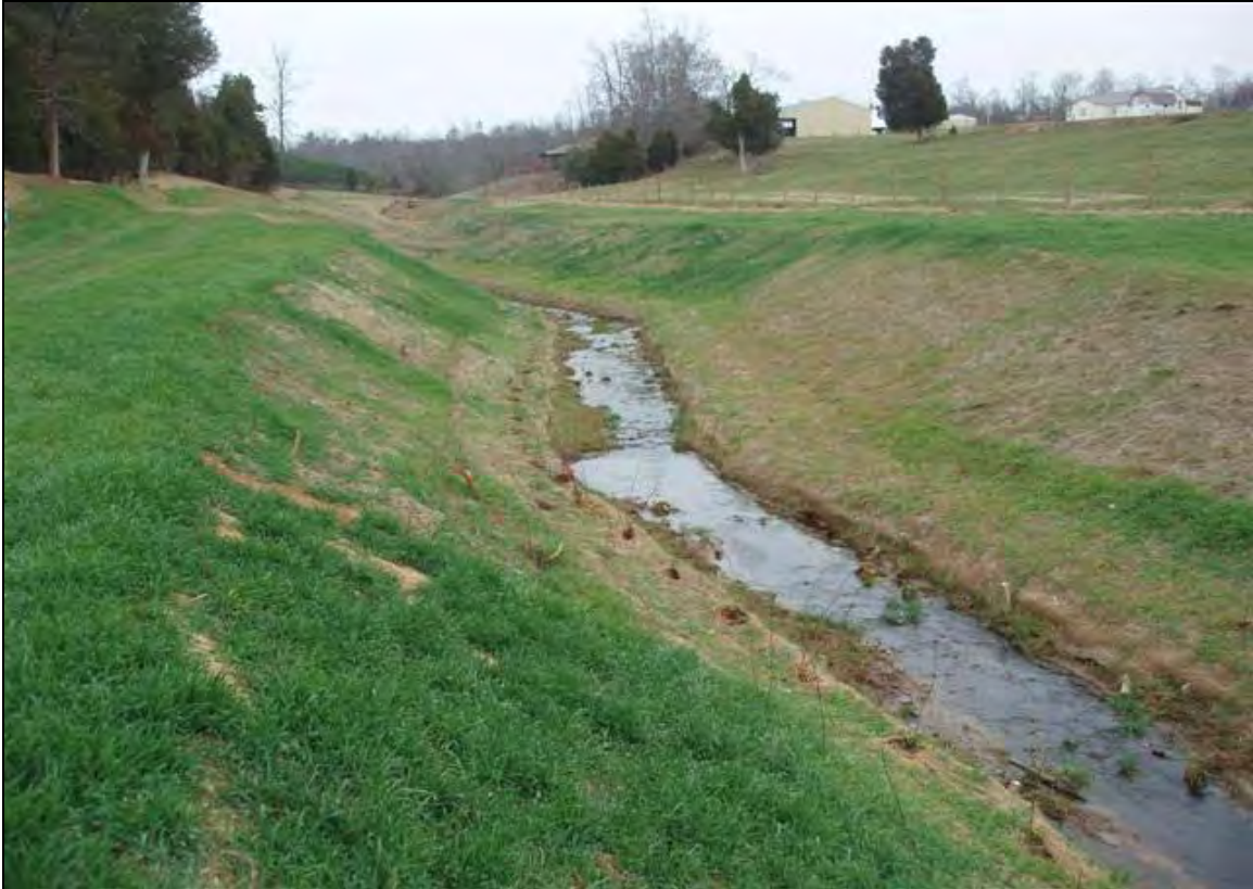
Photo Point 8a: View looking upstream taken near Station 20+75. 12/13/07 – As-Built
