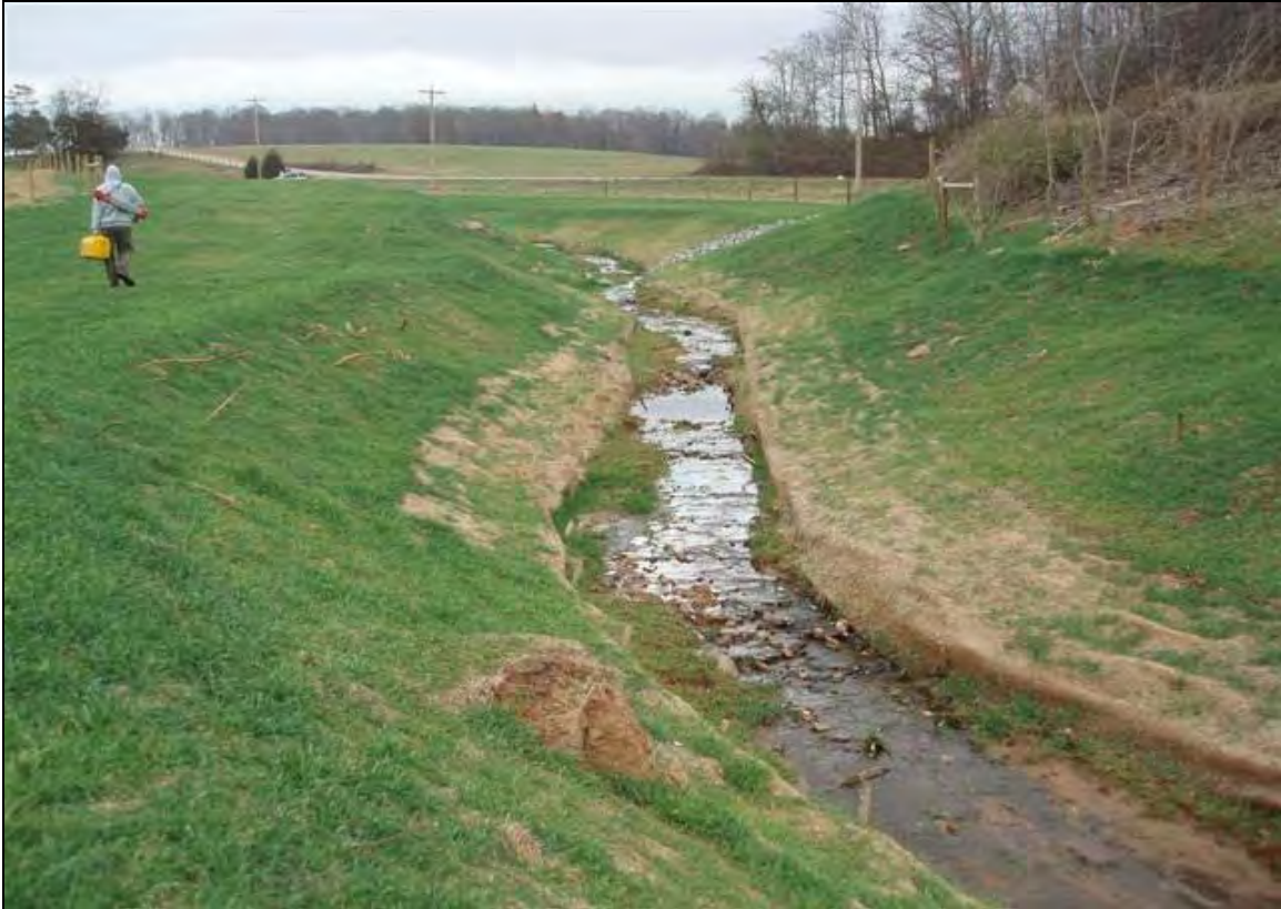
Photo Point 11a: View looking upstream taken near Station 27+65. 12/13/07 – As-Built
