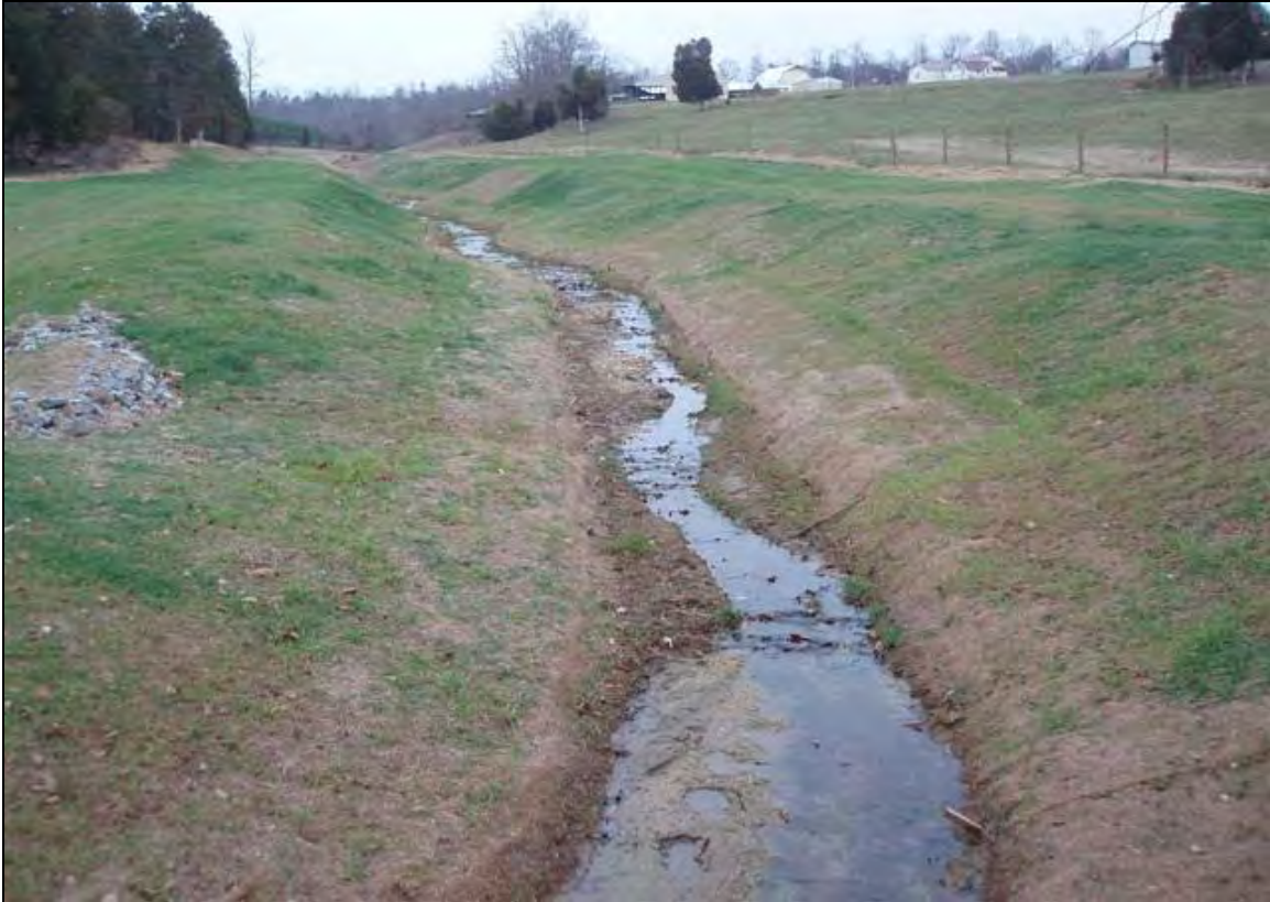
Photo Point 9a: View looking upstream from culvert. 12/13/07 – As-Built
