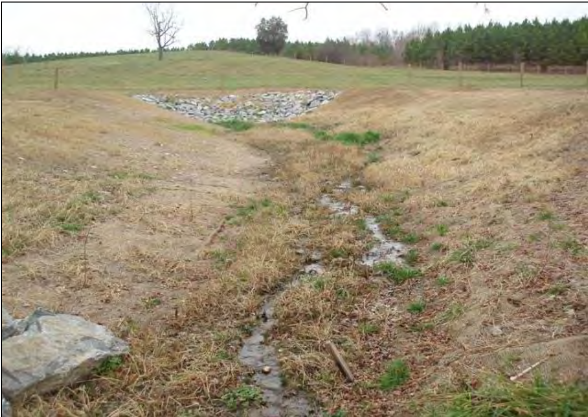
Photo Point 2a: Looking upstream on Tributary 1 at Station 10+00. 12/13/07 – As-Built
