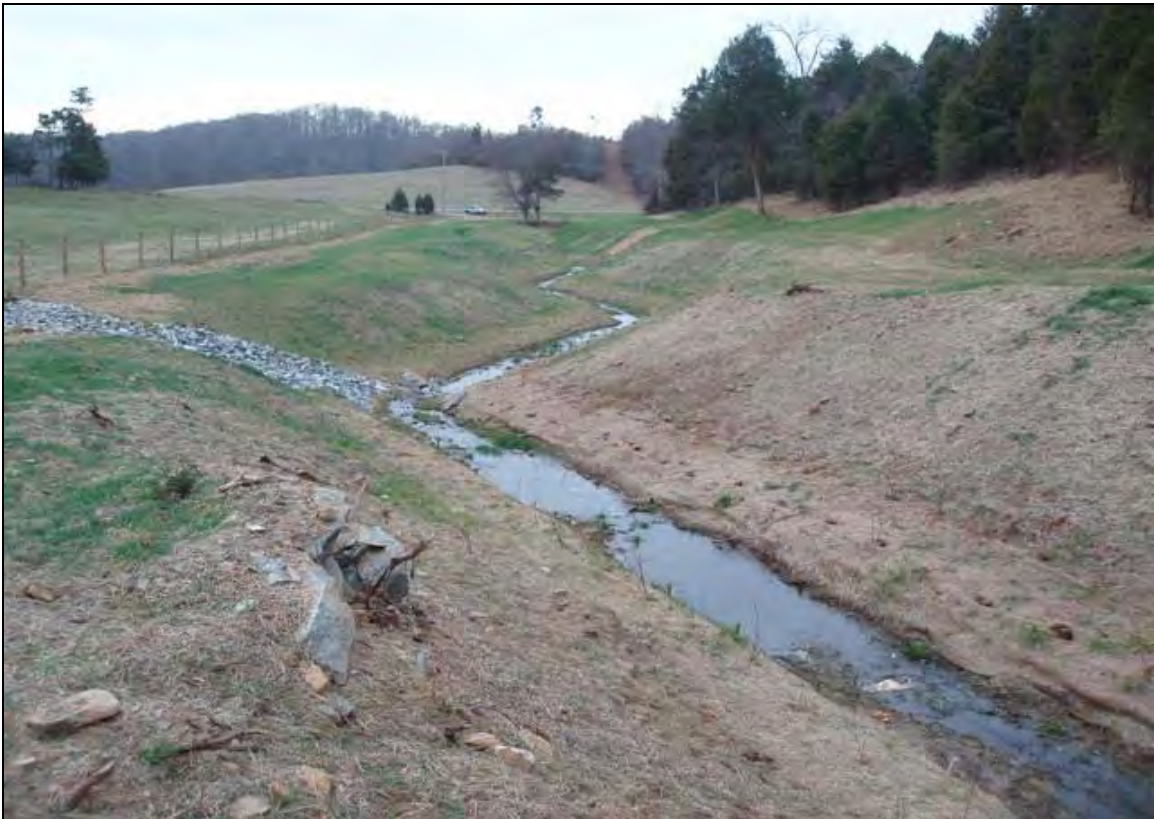
Photo Point 6b: View looking downstream taken near Station 15+75. 12/13/07 – As-Built
