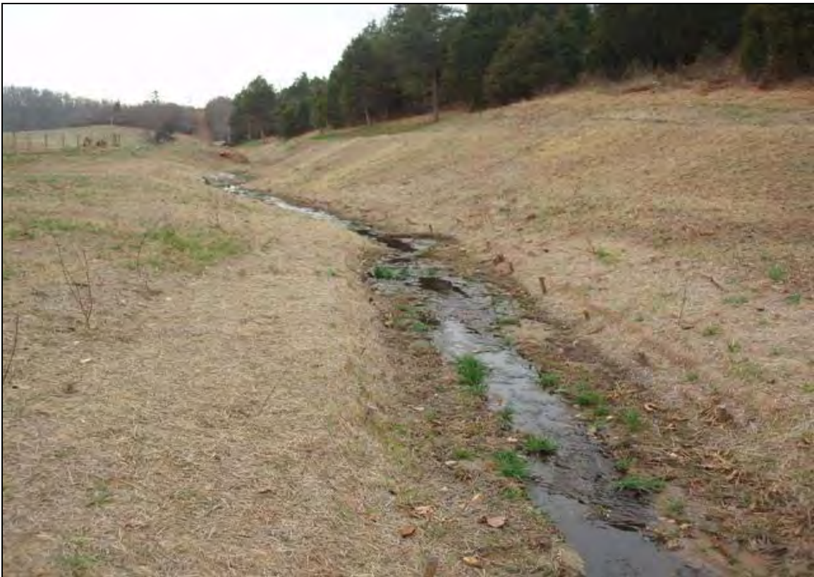
Photo Point 5b: View looking downstream taken near Station 12+50. 12/13/07 – As-Built
