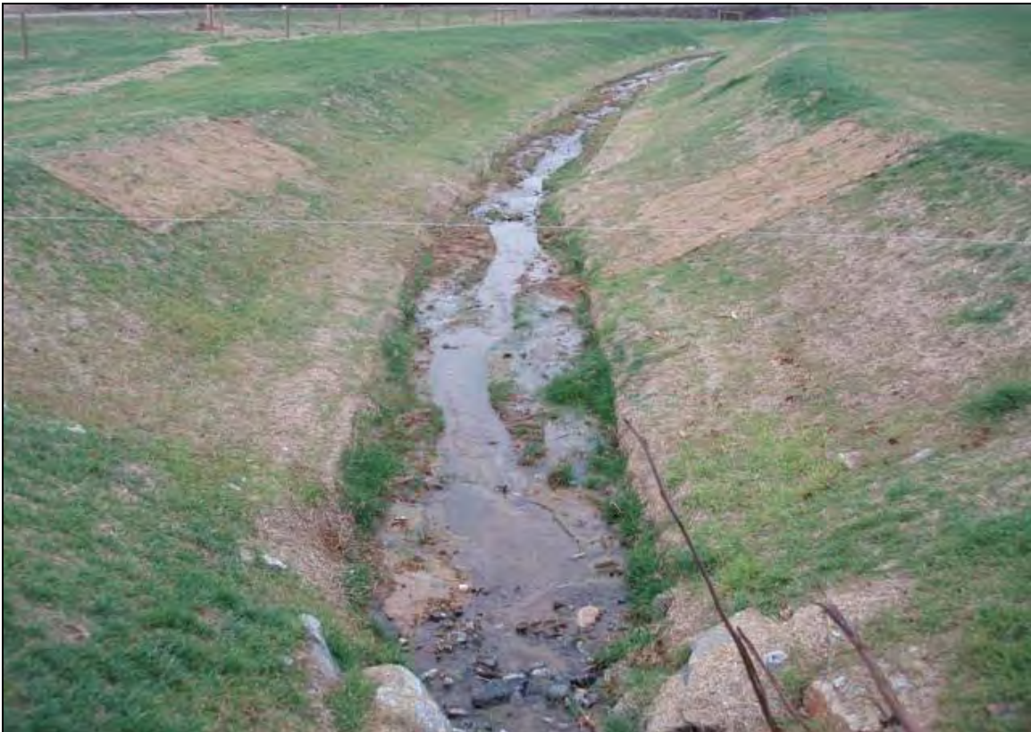
Photo Point 9b: View looking downstream from culvert. 12/13/07 – As-Built
