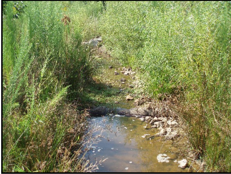
Photo 3. Typical log weir structure.
