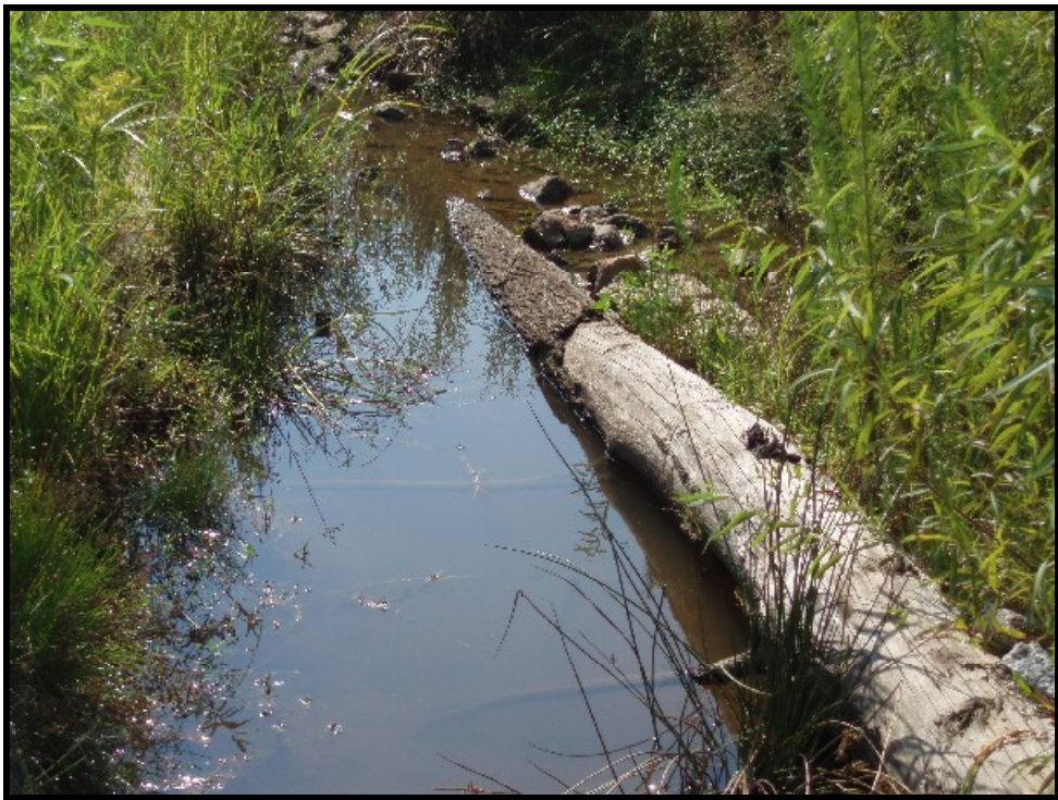
Photo 2. Typical log vane.
