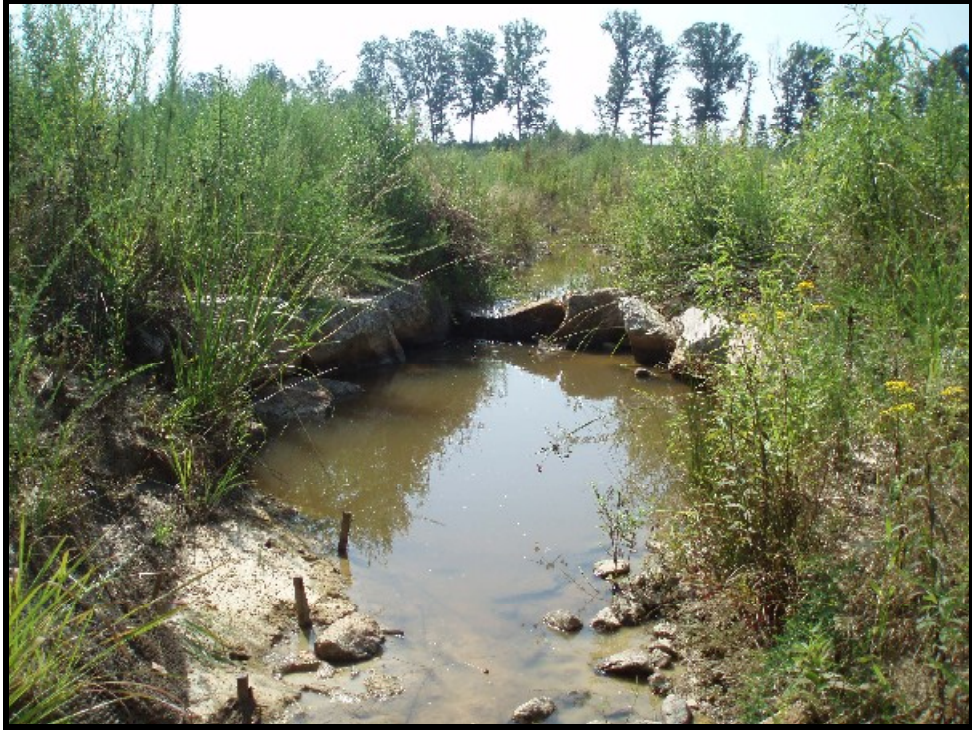
Photo 5. Typical rock cross vane.
