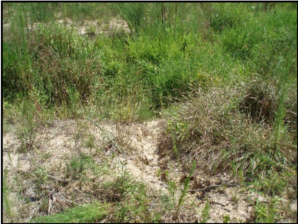
SPA 6. Mill Branch. STA 11+80, erosion occurring on right bank.
