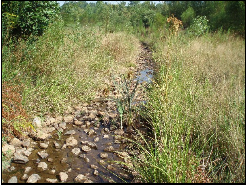
Photo 1. Typical constructed riffle structure.
