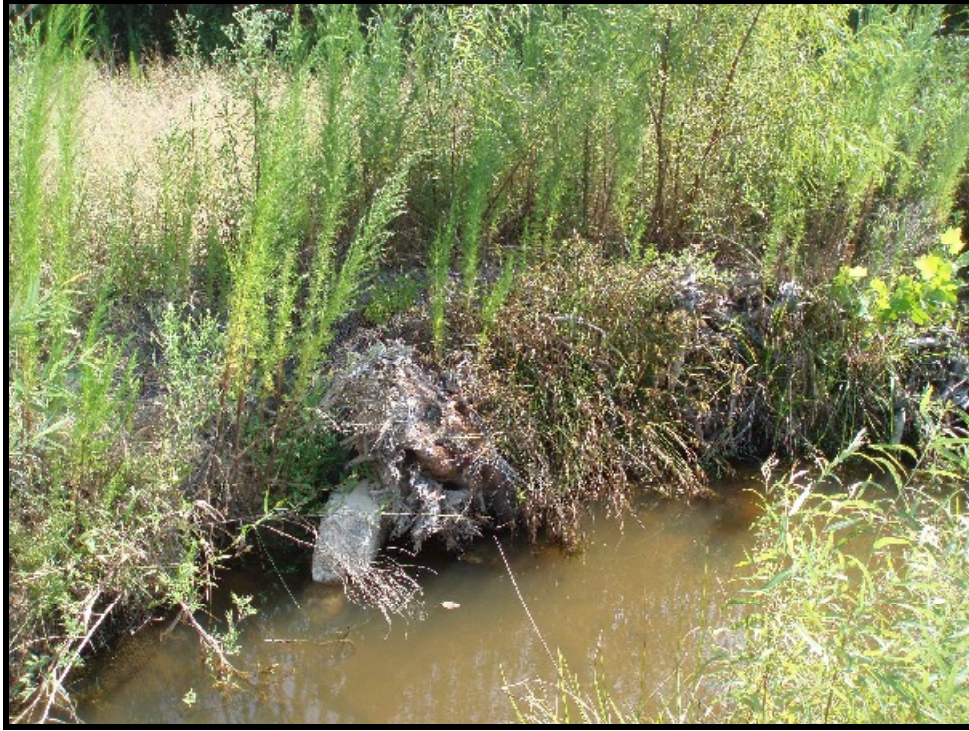
SPA 1. UT1. STA 11+50, minor erosion on right bank downstream of root wad structure.
