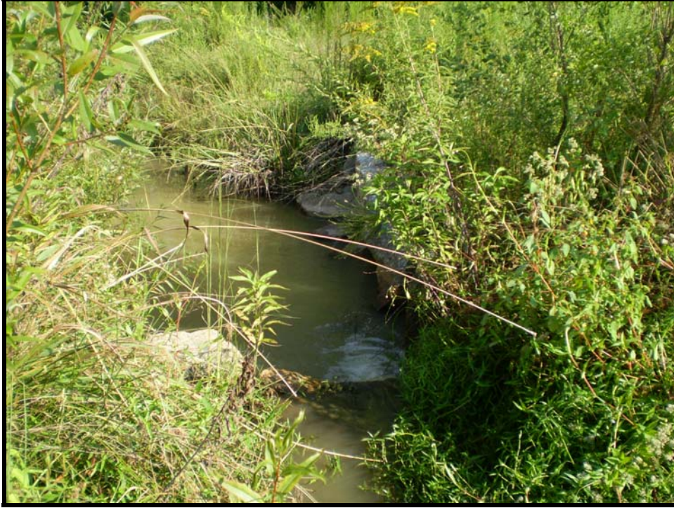
Rock cross vane facing downstream (typ.)
