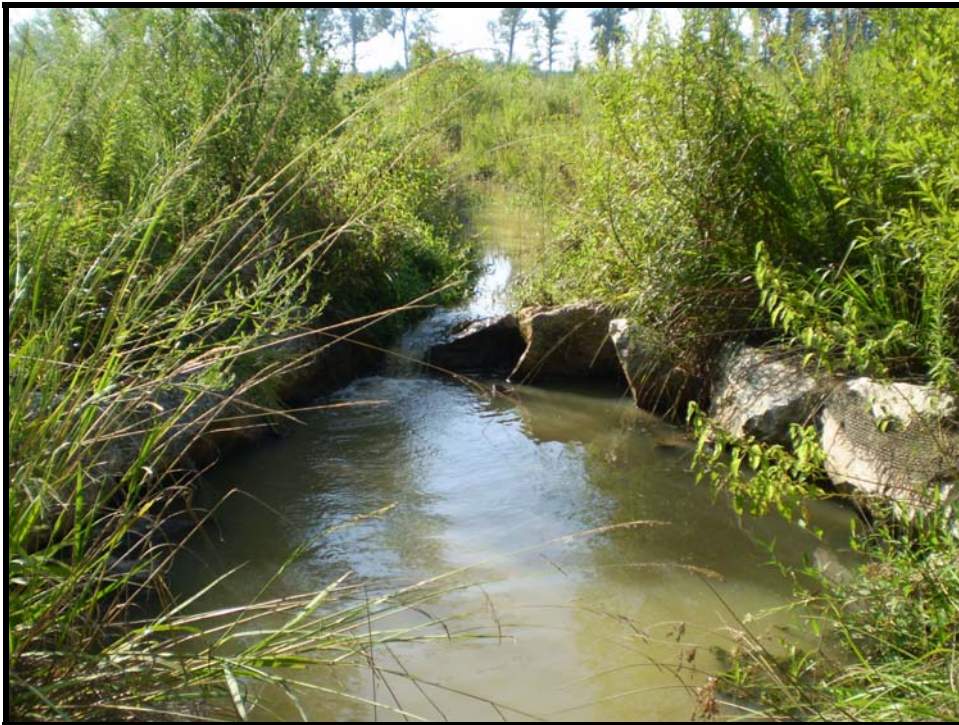
Rock cross vane facing upstream (typ.)
