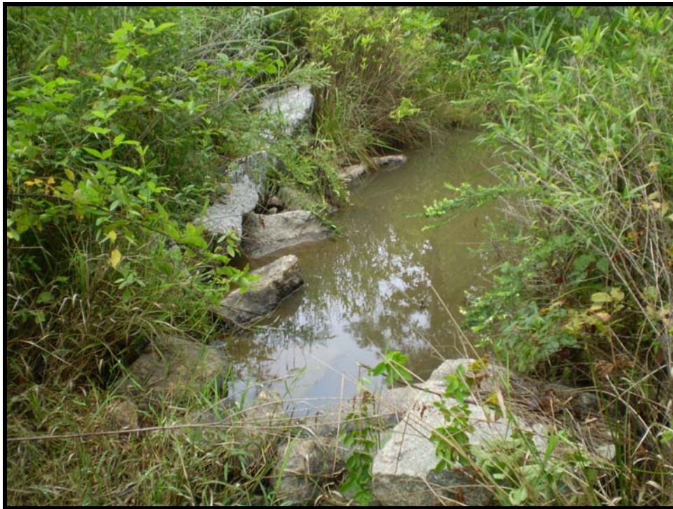
Rock cross vane facing downstream (typ.)
