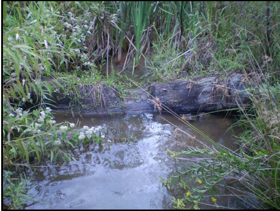
SPA 1, UT1 Station 20+25 – Log weir washed out; left and right bank erosion.
