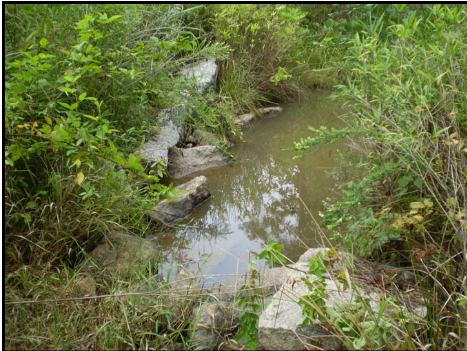
Rock cross vane facing downstream (typ.)
