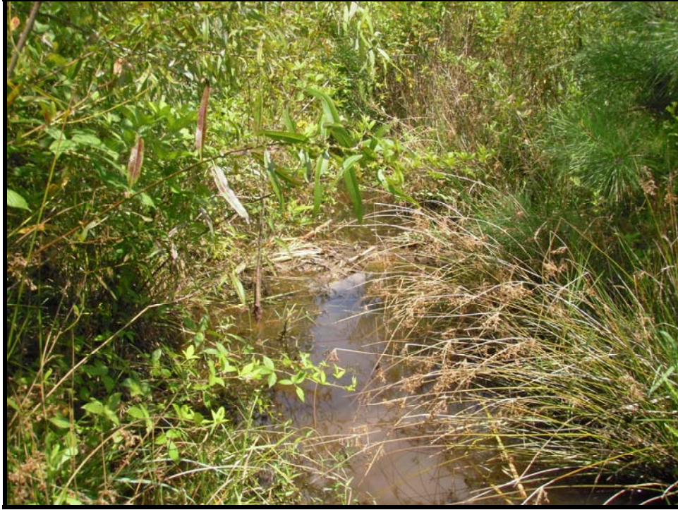
SOA 1, Mill Branch Station 17+25 – Beaver Dam
