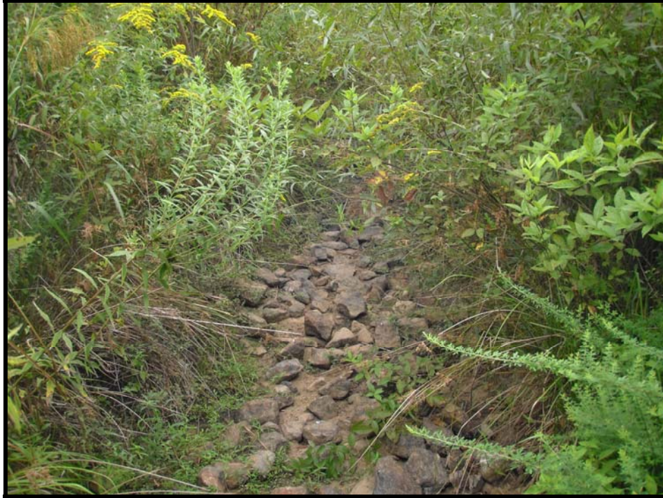
Constructed riffle facing upstream on UT1 (typ.)
