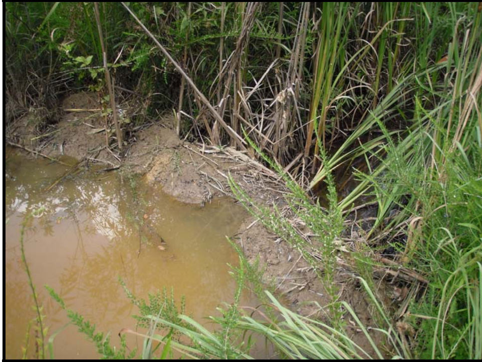
SOA 3, Mill Branch Station 19+50 – Beaver Dam
