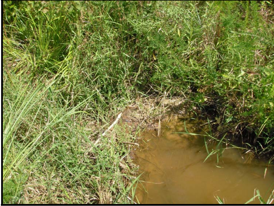
SOA 5, Mill Branch Station 27+00 – Beaver Dam
