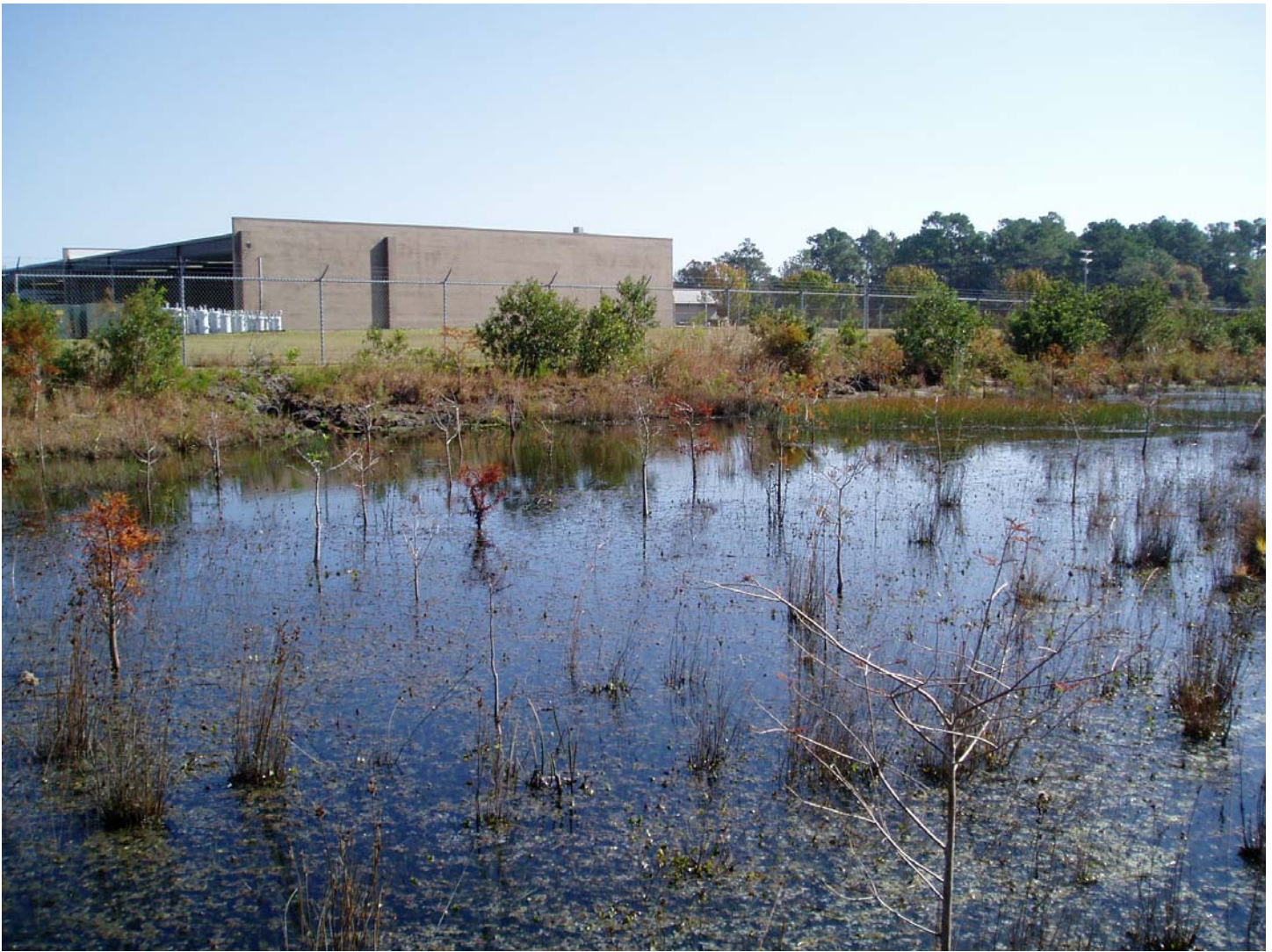
Photo 3. West Cell - above weir
