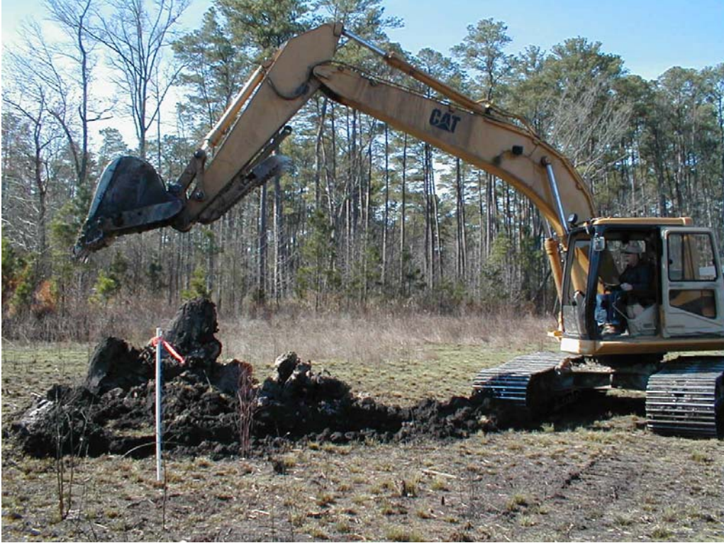
Figure 10. Soil pit excavation.
