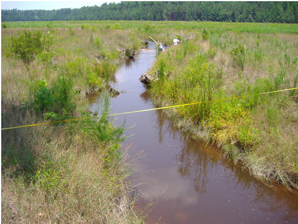
Photo Station 10. End of Project – Upstream
