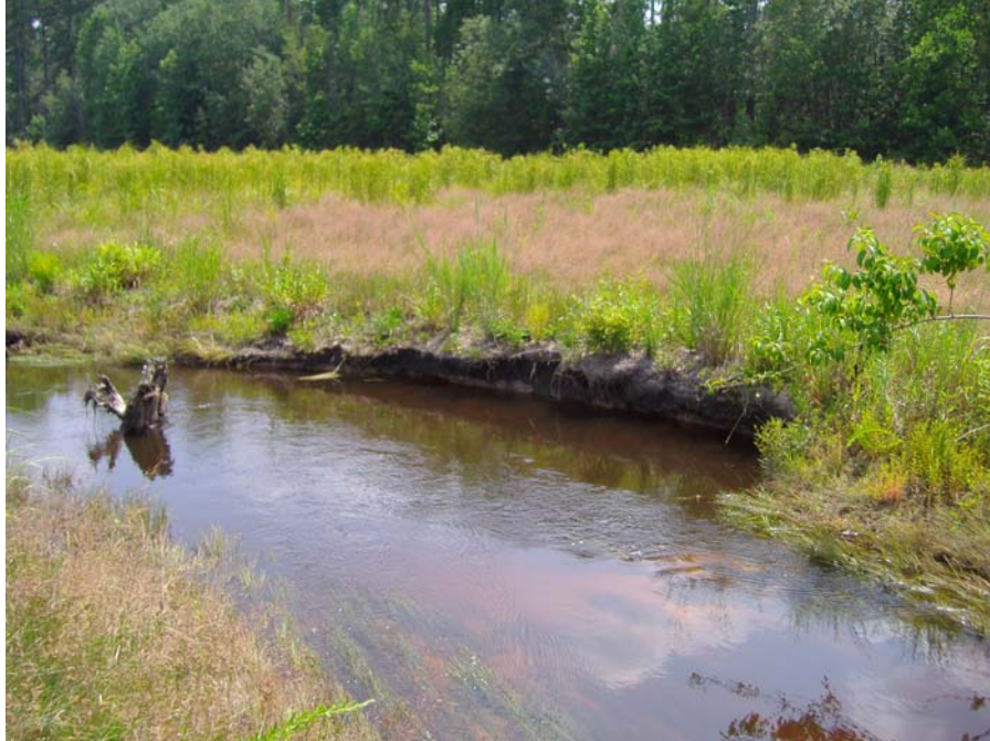
Photo 7. Bank erosion developing around the meander bends at various locations of the project (7/4/07)
