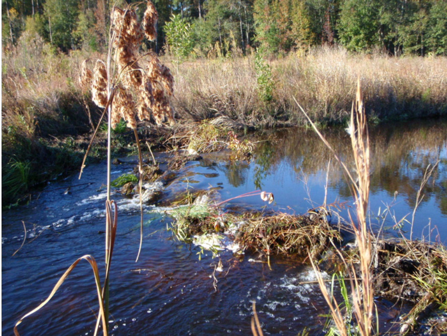
Photo 3. Beaver dam with scour on right bank (2/08/2008).
