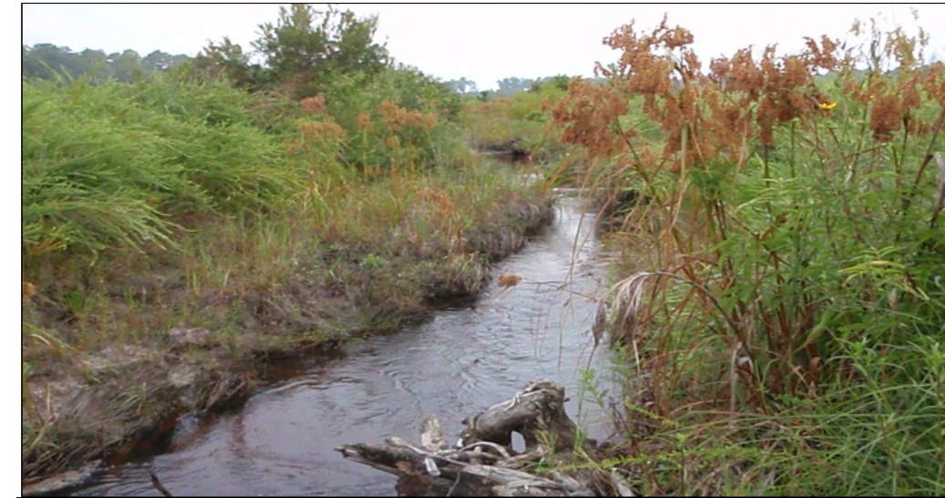
Photo of Cross-Section 7 - Looking Downstream @ STA 37+24
