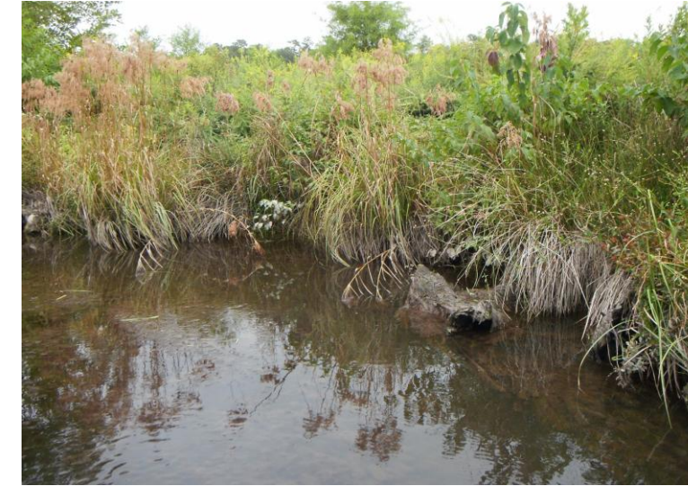
Photo of Cross-Section 4 - Looking Upstream @ STA 20+93
