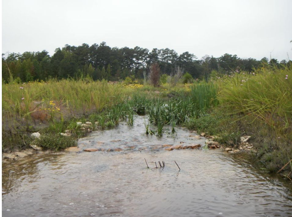
Photo 3. Repaired reach looking upstream near Station 35+50 (9/21/11)
