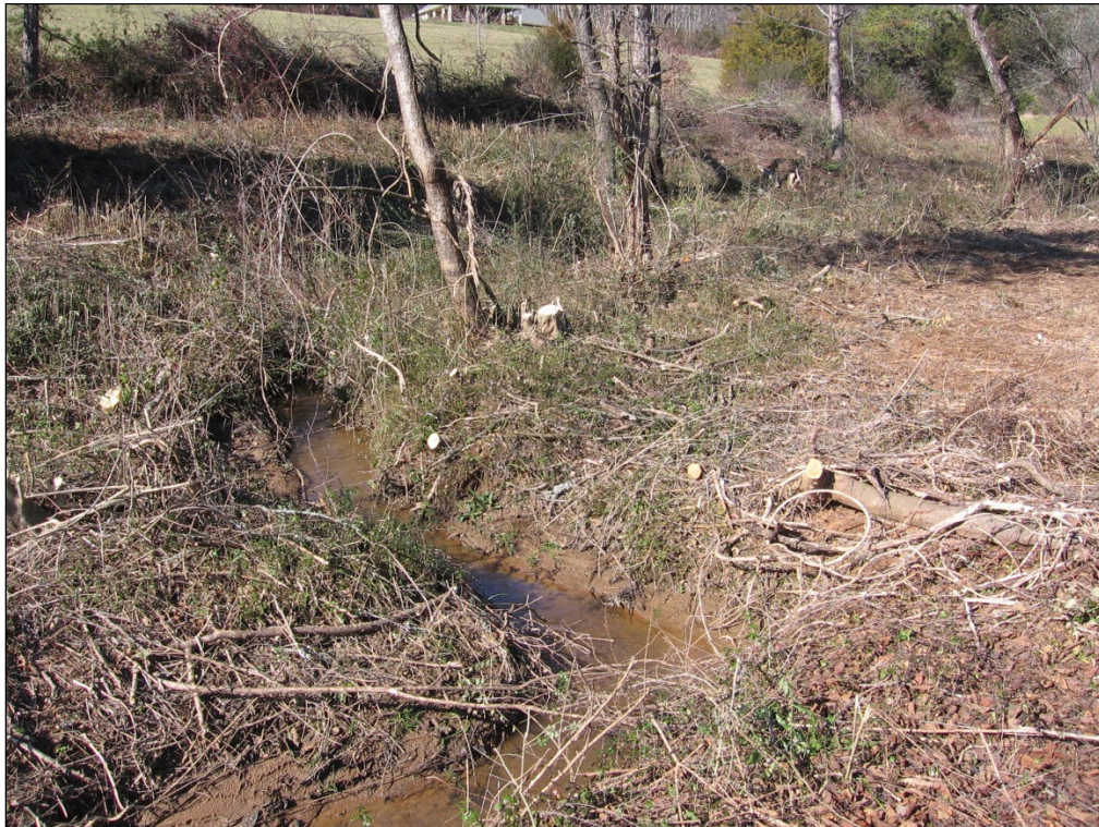
Upstream of Culvert on June's Branch @ Sta 213+00
