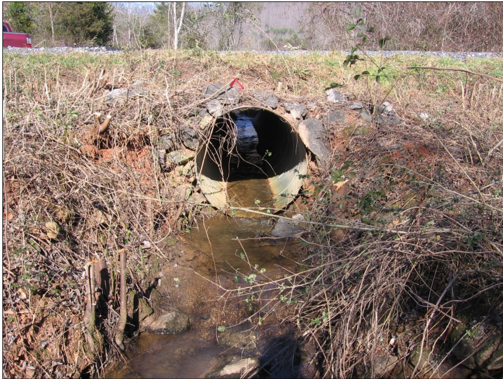
Culvert on June's Branch facing upstream @ Sta 213+00
