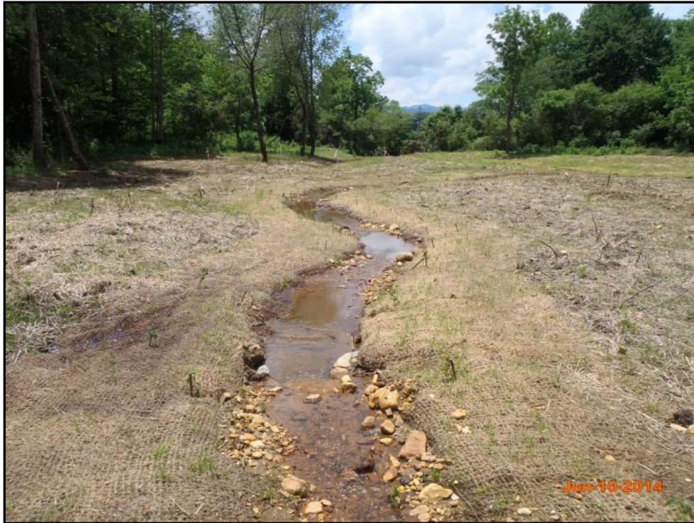
Higdon Creek – Permanent Photo Station 13 Station 302+80 - Downstream
