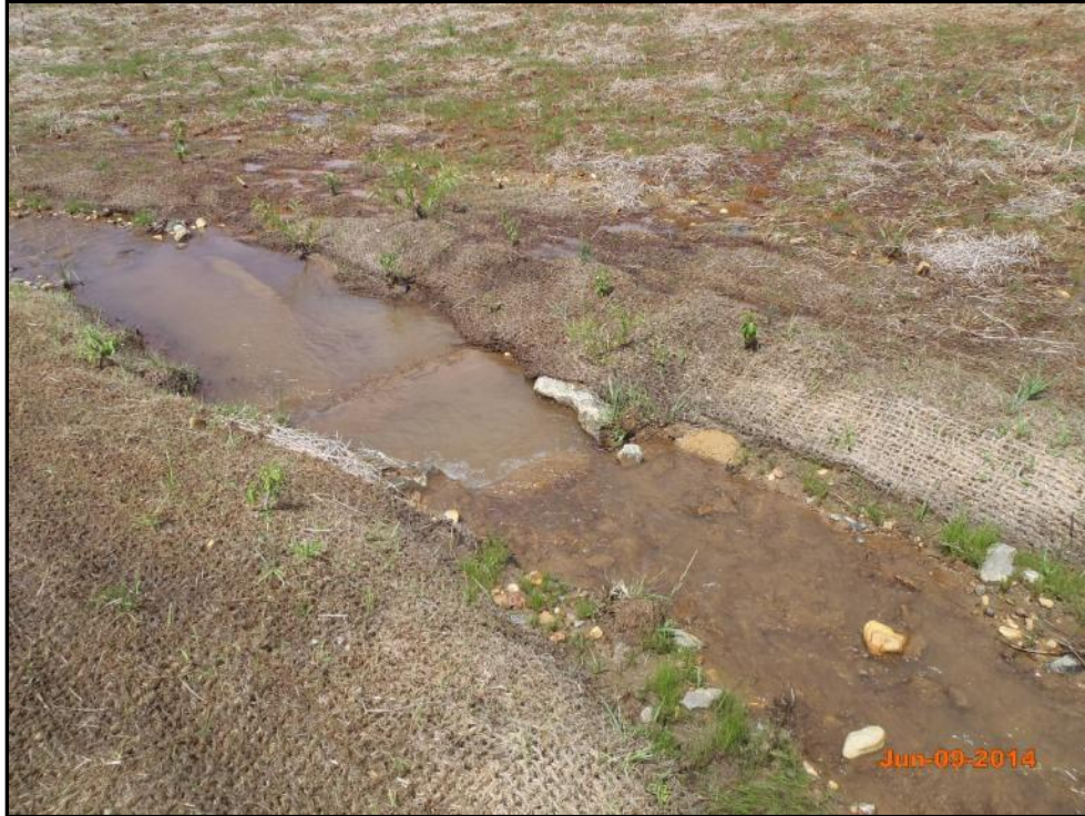
Junes Branch – Permanent Photo Station 4 Station 210+60 - Downstream
