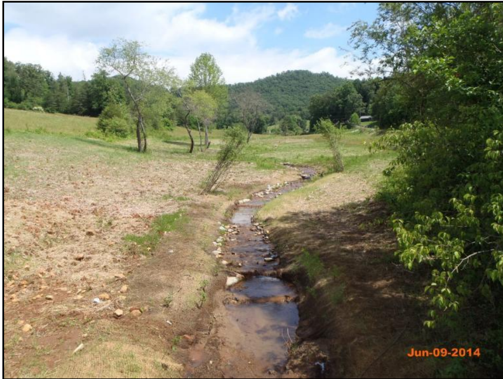
Junes Branch – Permanent Photo Station 6 Station 214+00 - Upstream
