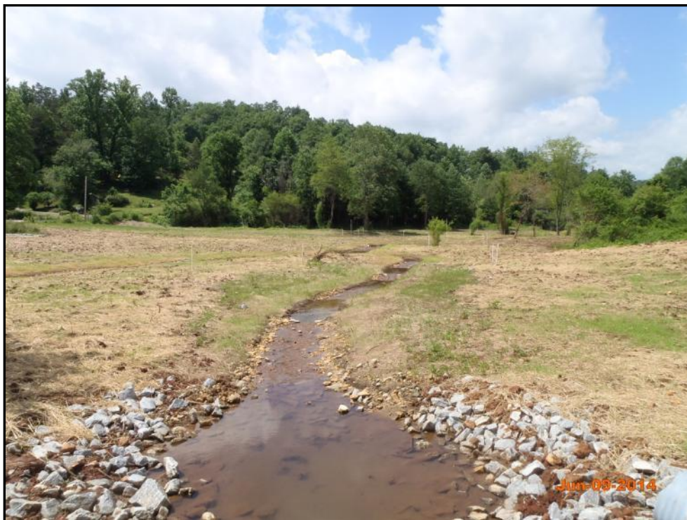
Junes Branch – Permanent Photo Station 6 Station 214+00 - Downstream
