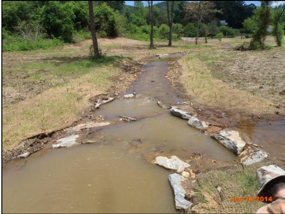
Bumgarner Branch II – Permanent Photo Station 11 Looking Upstream from Confluence with Higdon Branch
