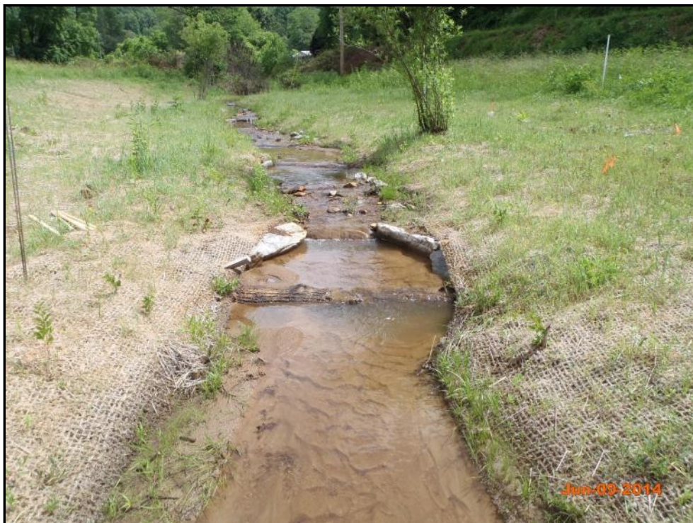
Junes Branch – Permanent Photo Station 1 Station 202+75 - Upstream
