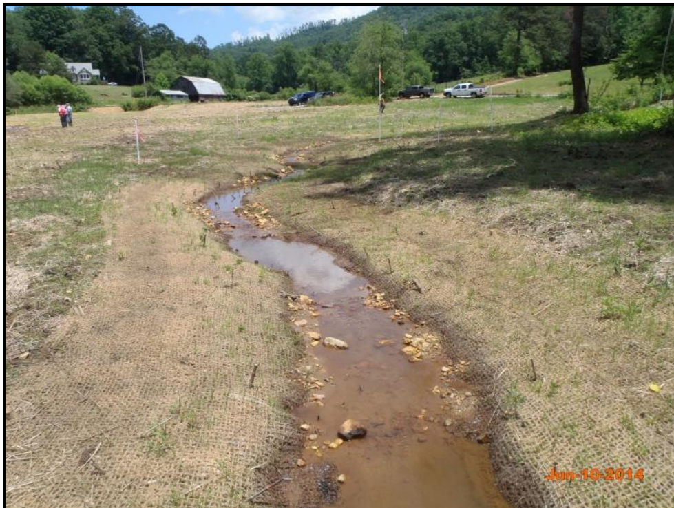
Higdon Creek – Permanent Photo Station 13 Station 302+80 - Upstream
