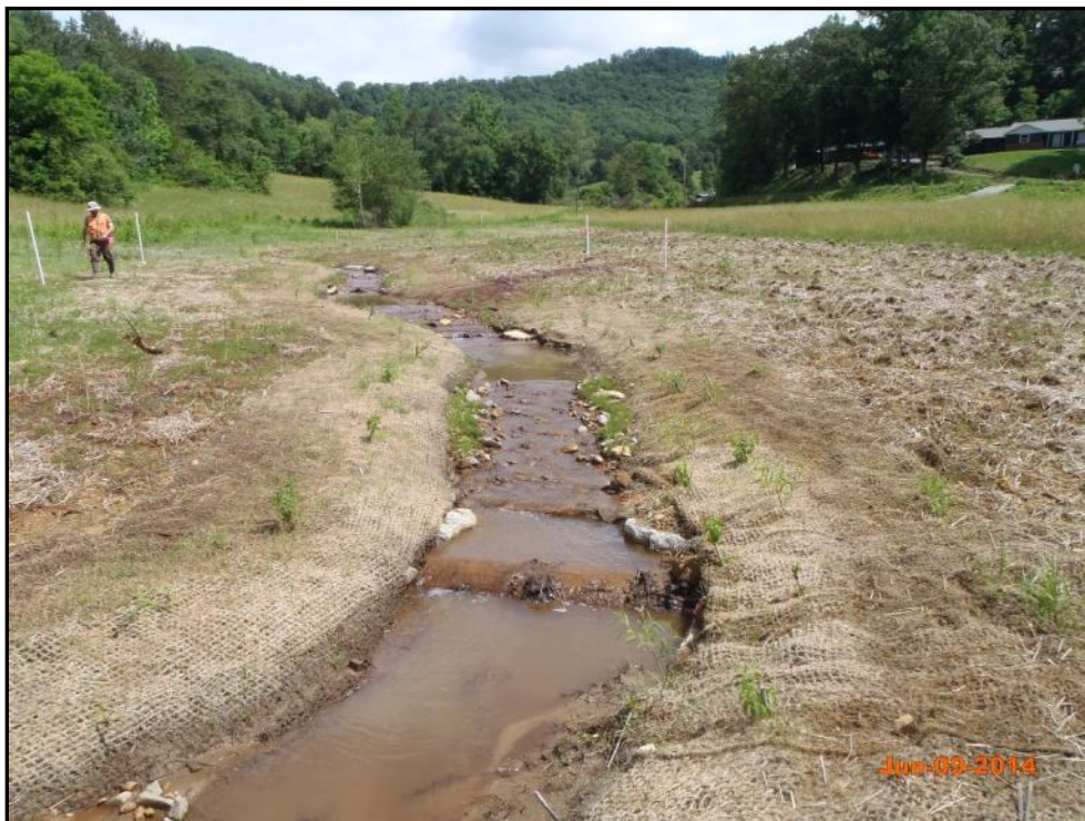
Junes Branch – Permanent Photo Station 4 Station 210+60 - Upstream
