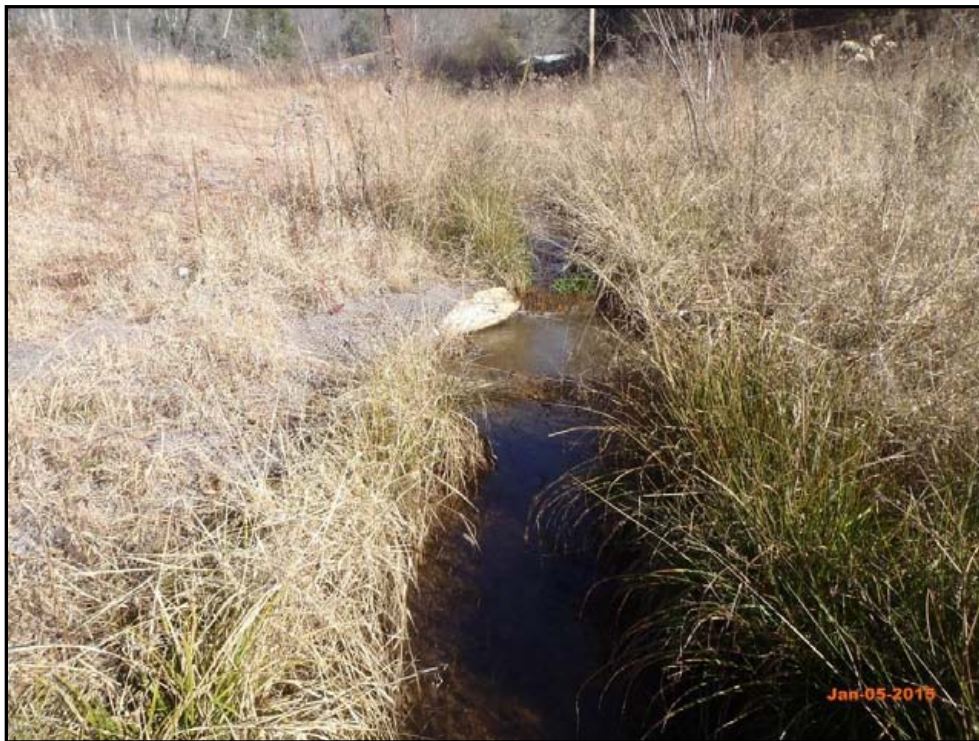
Junes Branch – Permanent Photo Station 1 Station 202+60 - Upstream
