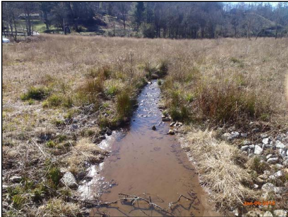
Junes Branch – Permanent Photo Station 6 Station 214+00 - Downstream
