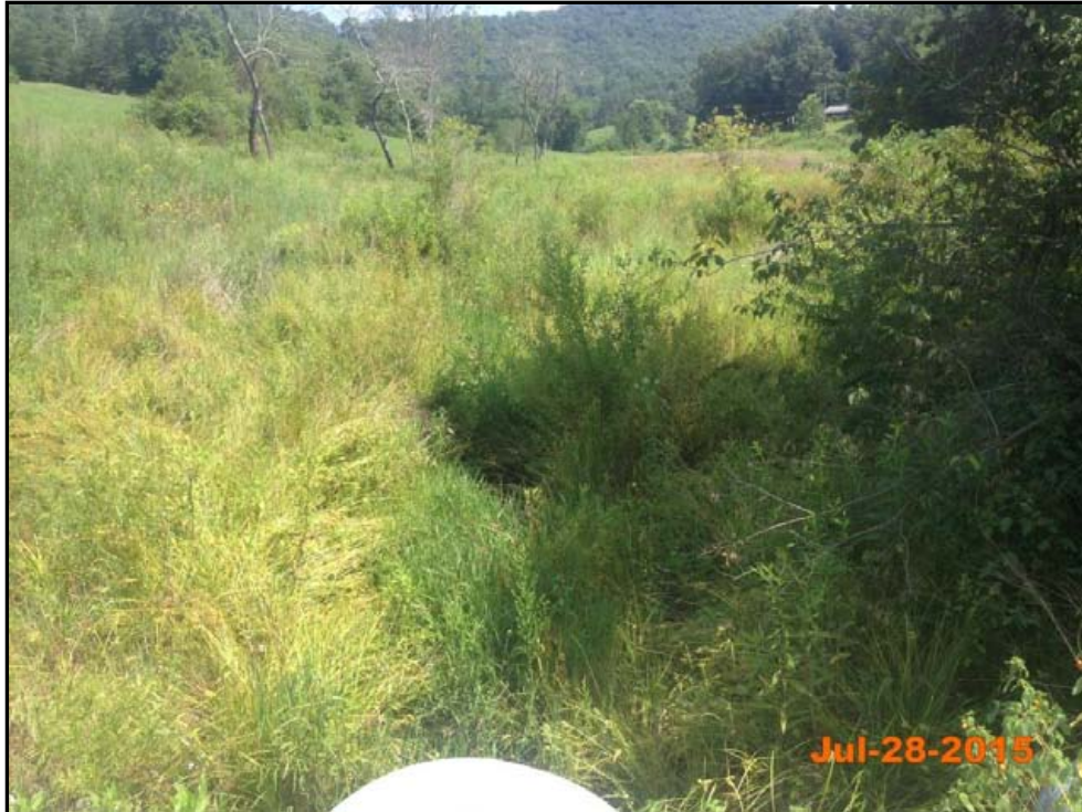
Junes Branch – Permanent Photo Station 6 Station 214+00 - Upstream
