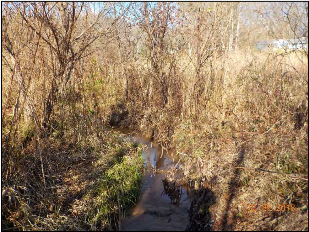
Junes Branch – Permanent Photo Station 2 Station 206+30 – Upstream
