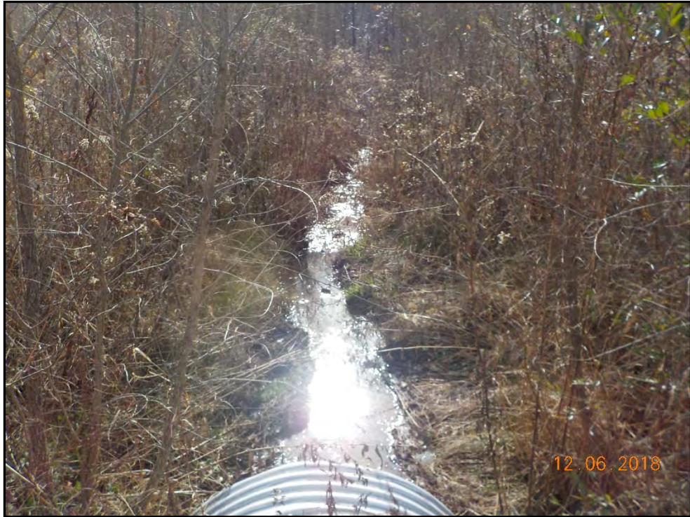
Junes Branch – Permanent Photo Station 6 Station 214+00 – Downstream
