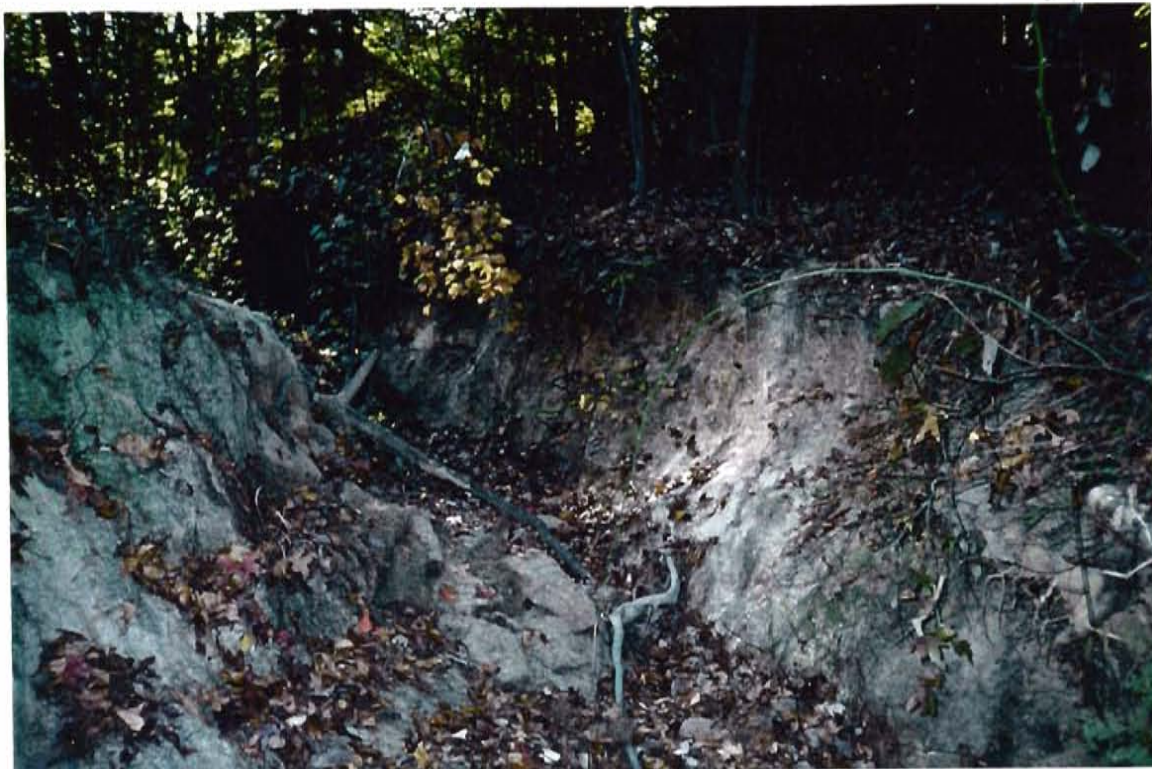
Unnamed Tributary to Bushy Branch looking upstream near culvert outlet.
