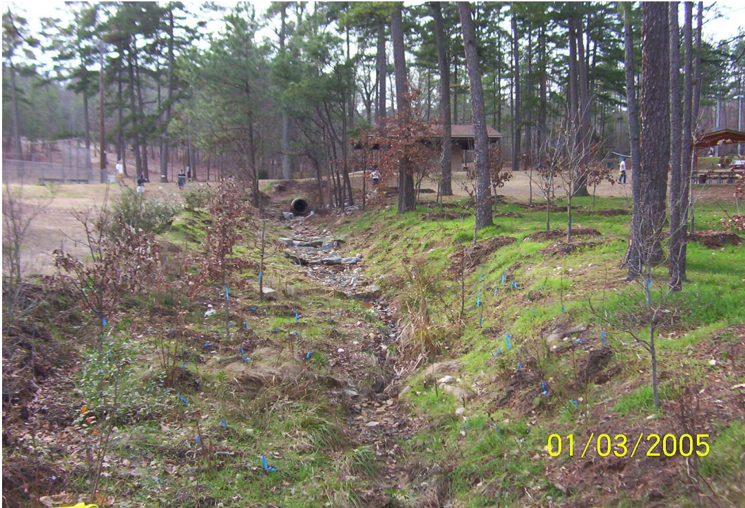
Photo Location 3: Standing on pedestrian bridge over UT looking upstream
