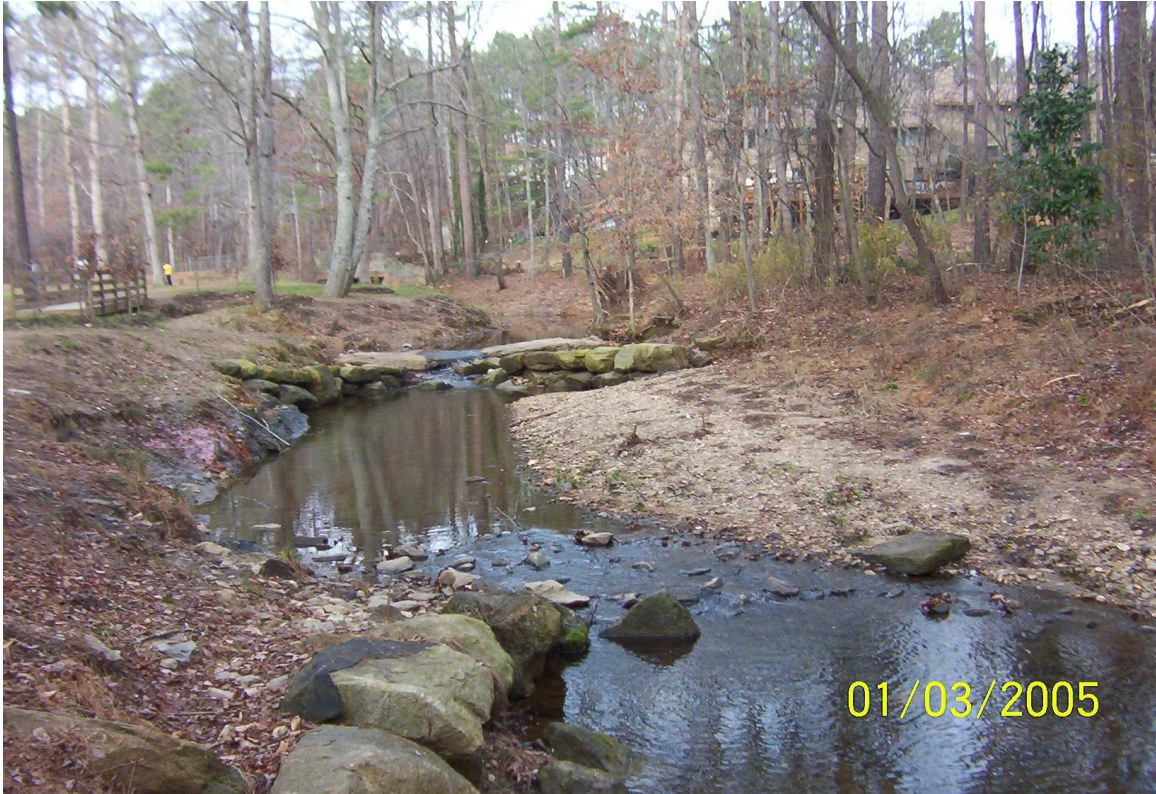
Photo Location 4: Looking upstream toward a J-hook, a cross vane, and the confluence.
