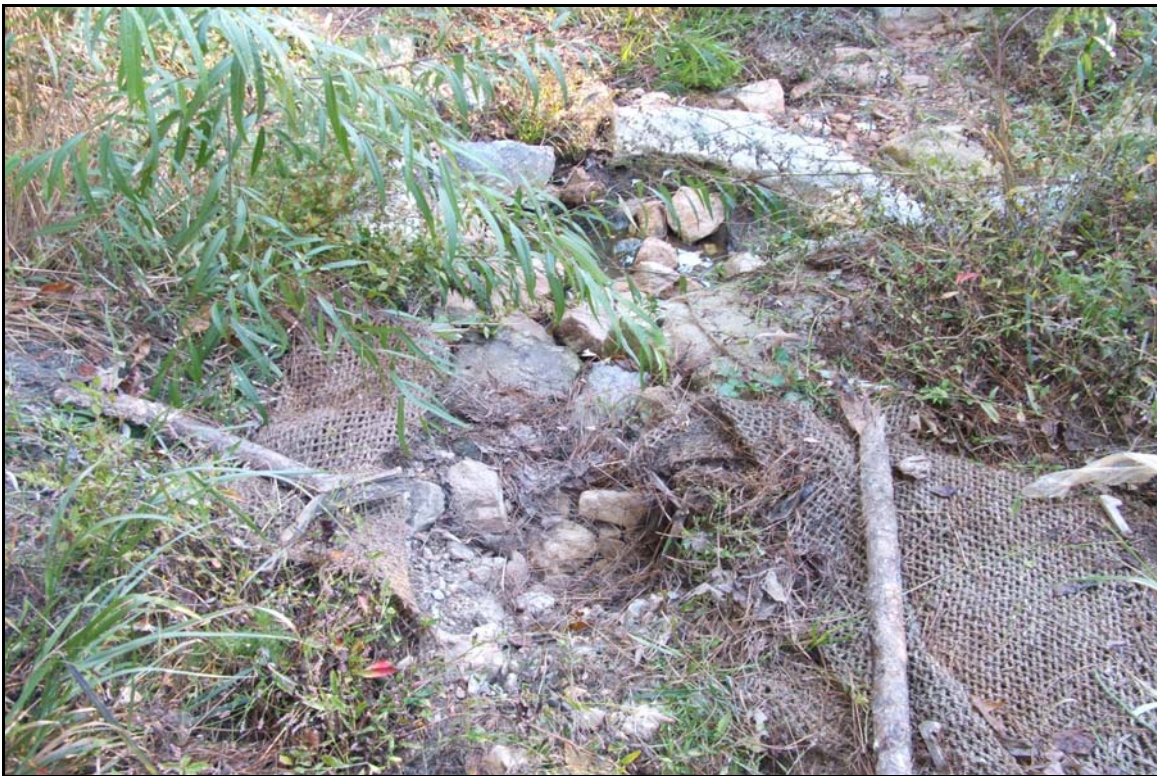
SP6 – Hole degrading on upstream side of cross vane. Photo taken near station 02+25. 10/27/05 - MY 01
