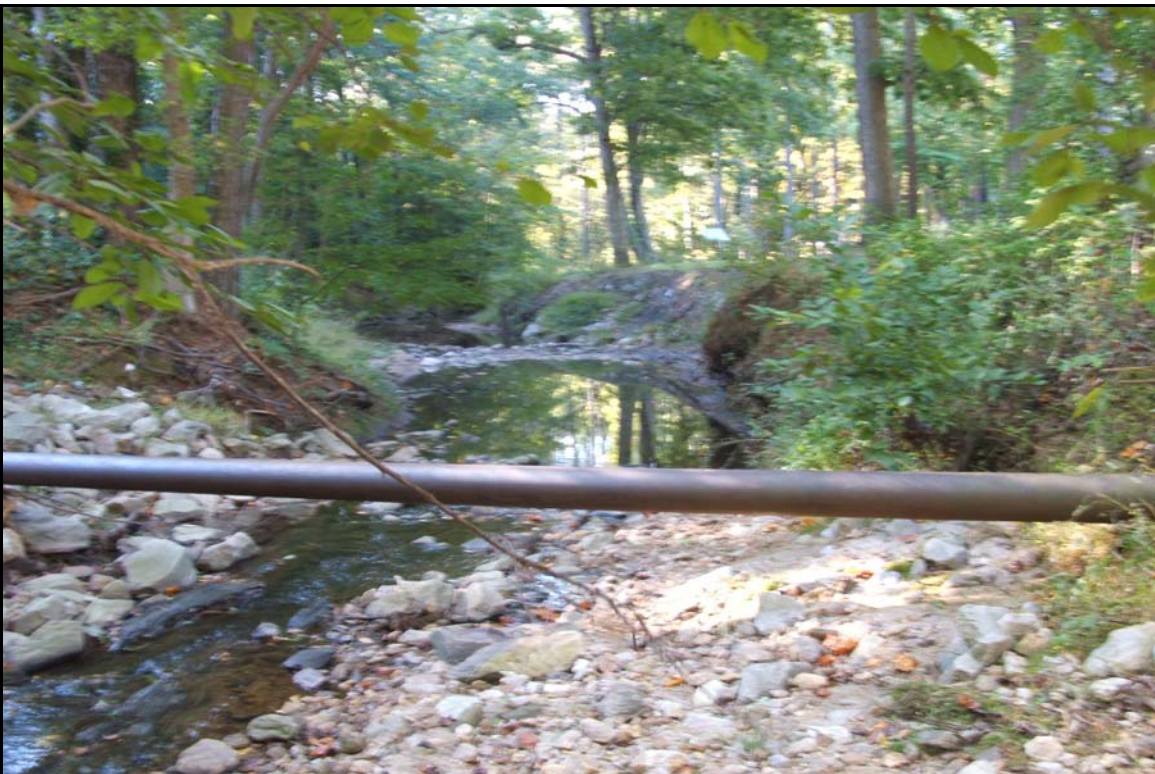
Photo Point 1, supplemental – Taken looking downstream from streambed in front of bridge on Kaplan Drive. 10/27/05 - MY 01
