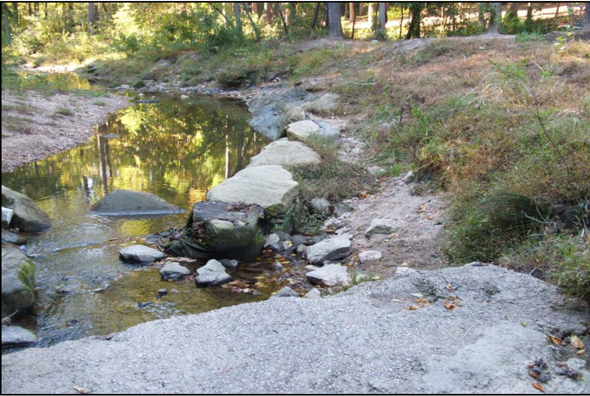
SP3 – Back arm scour on right arm of cross vane. Photo taken near station 12+60. 10/27/05 - MY 01
