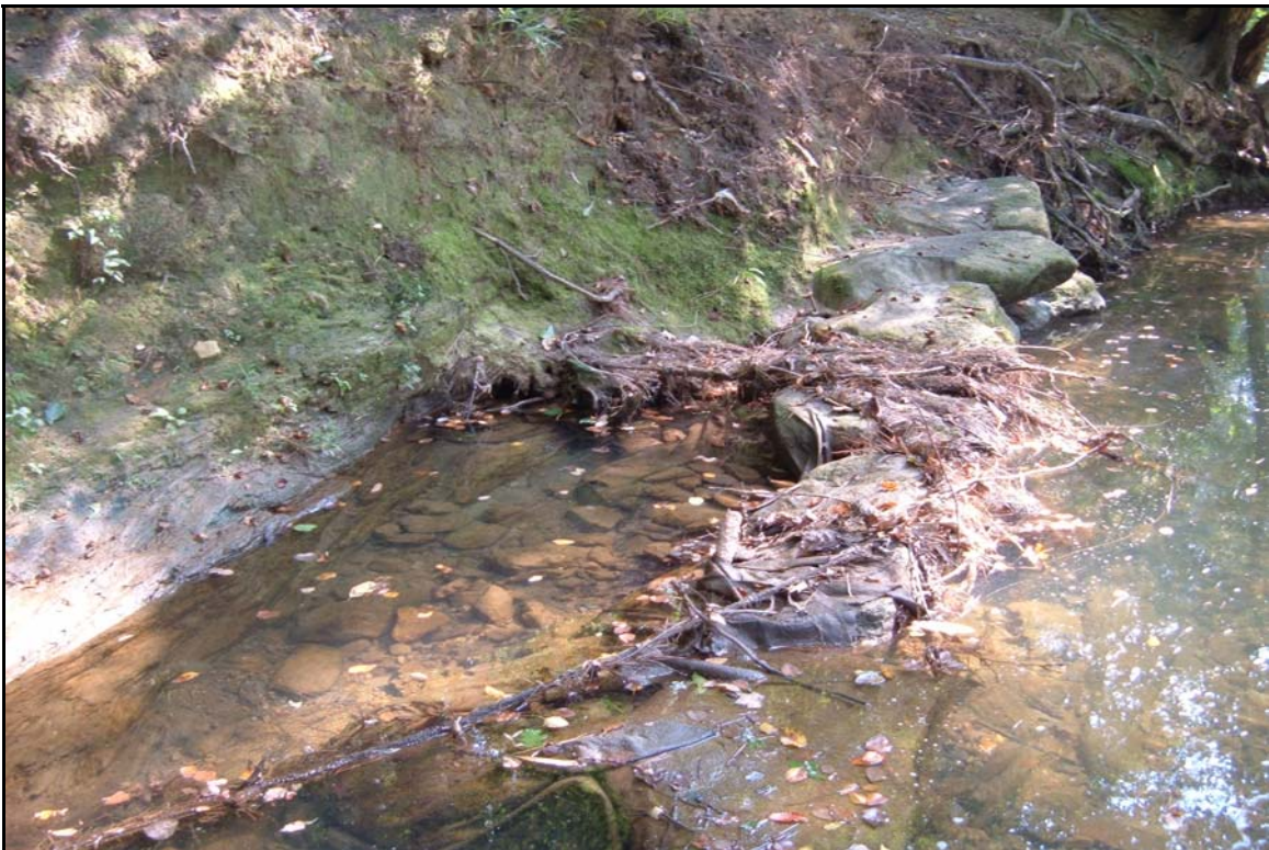
SP2 – Back arm scour on arm of j-hook. Photo taken near station 11+75. 10/5/06 - MY 02
