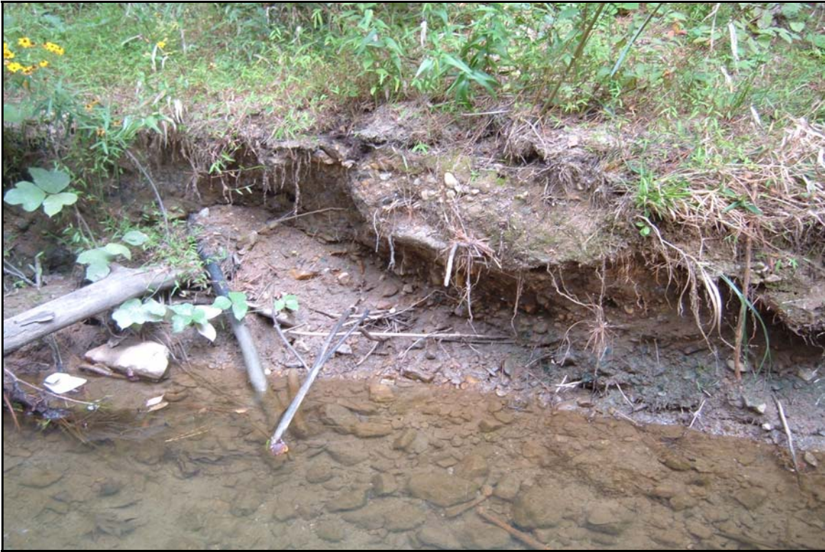
SP1 – Bank erosion. Photo taken near station 15+65 on left bank. 10/5/06 - MY 02
