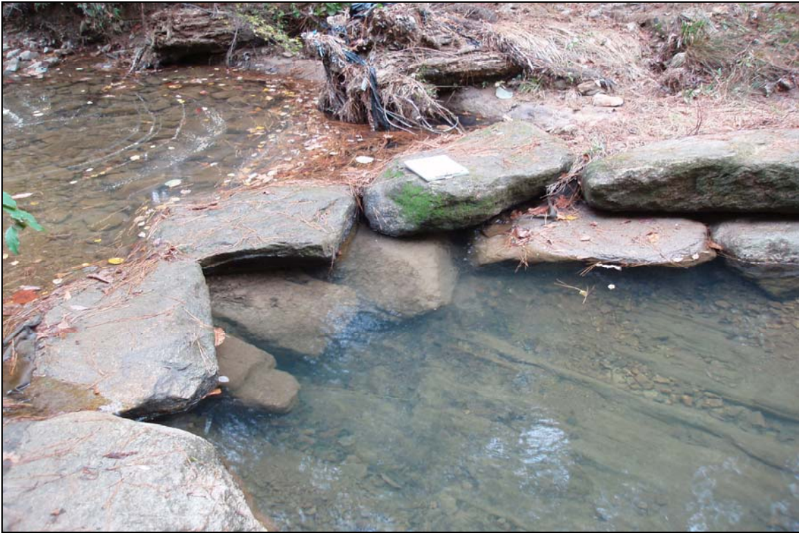
SP3 - Piping through boulders in cross vane. Photo taken near Station 16+00. 11/12/07 - MY 03
