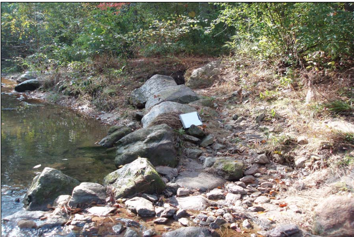
SP2 - Back arm scour on arm of J-hook. Photo taken near Station 13+50. 11/12/07 - MY 03
