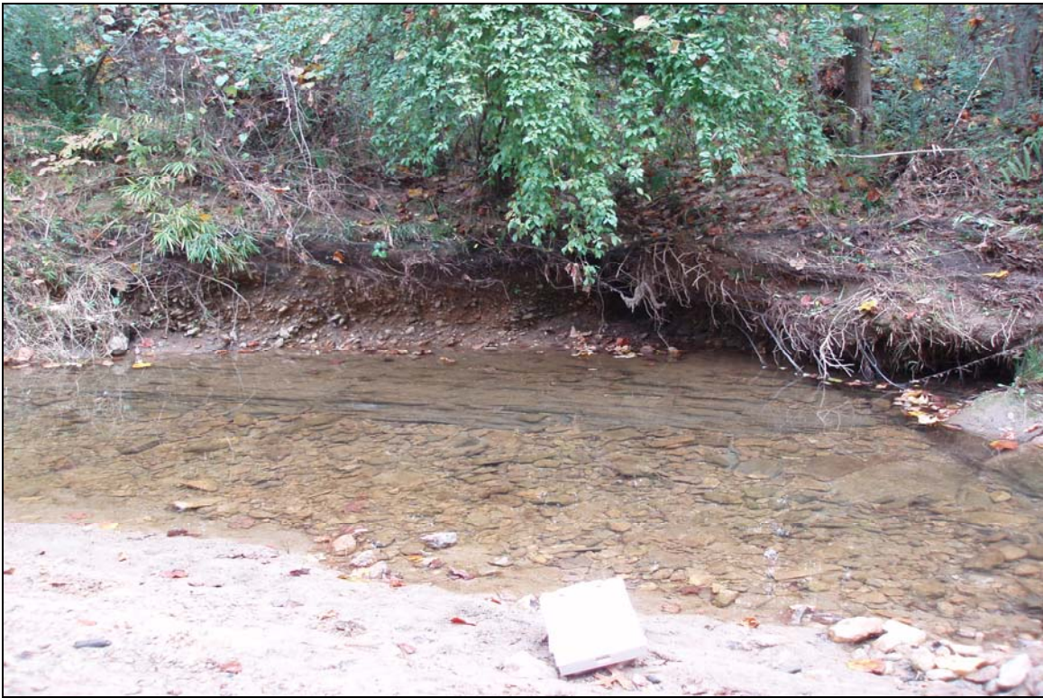
SP1 - Bank erosion. Photo taken near Station 17+95 on left bank. 11/12/07 - MY 03
