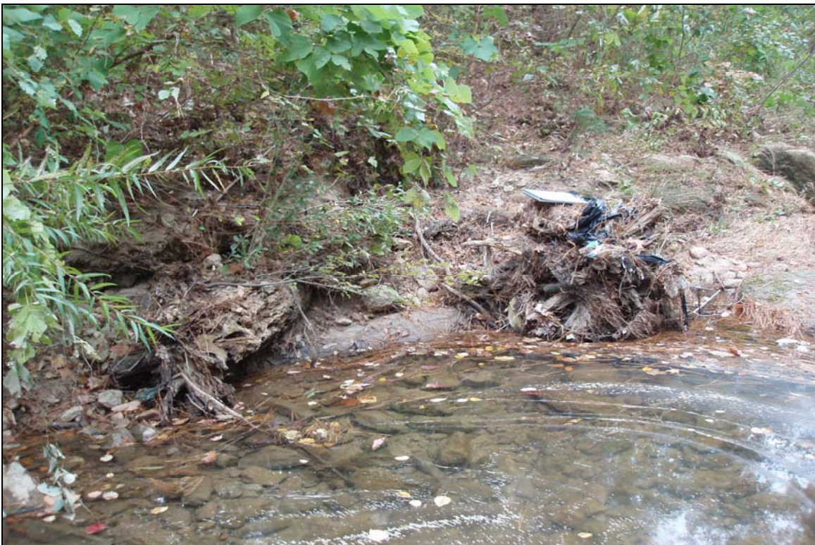
SP4 - Scour behind root wads. Photo taken near Station 16+00. 11/12/07 - MY 03
