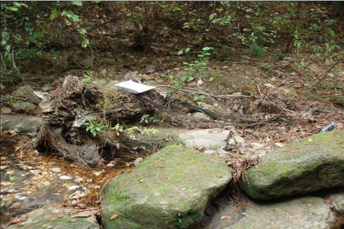
SP4 - Scour behind failed root wads. Photo taken near Station 16+00. 10/28/08 - MY 04
