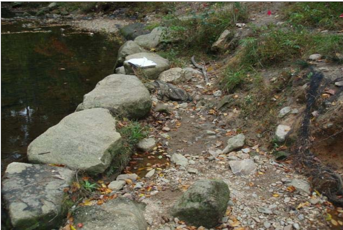
SP2 - Back arm scour on arm of cross vane. Photo taken near Station 12+60. 10/28/08 - MY 04
