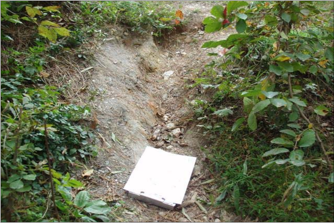
VP5 - Erosion from path worn into stream bank from pedestrian access to the stream. Photo taken near Station 01+00. 10/27/08 - MY 04
