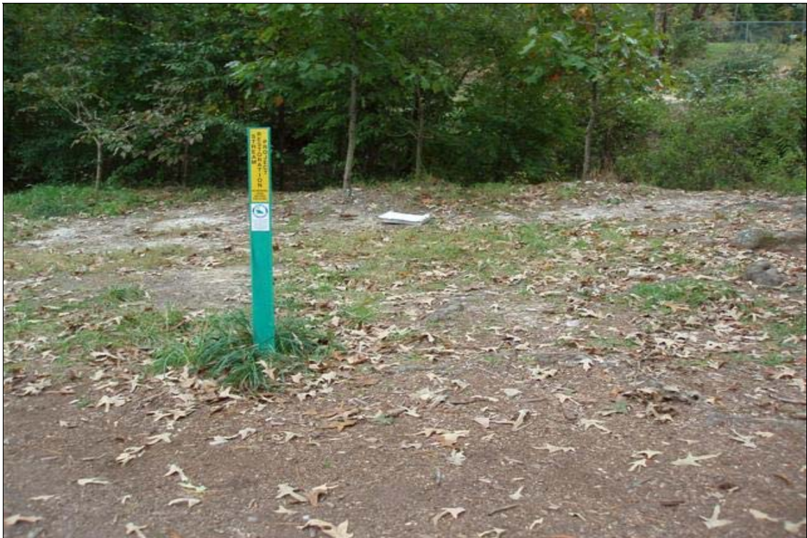
VP4 – Easement area mowed and worn by pedestrian traffic. Photo taken near Station 02+50. 10/27/08 - MY 04
