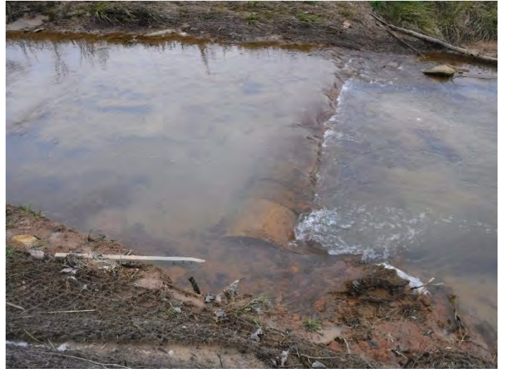
Bull Creek R3 Structure Failure at Station 157+00 – Looking from Right bank (12/30/2020)
