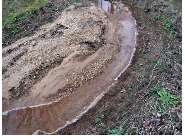
UTC3 Aggradation at Station 408+52 – looking upstream (12/30/2020)
