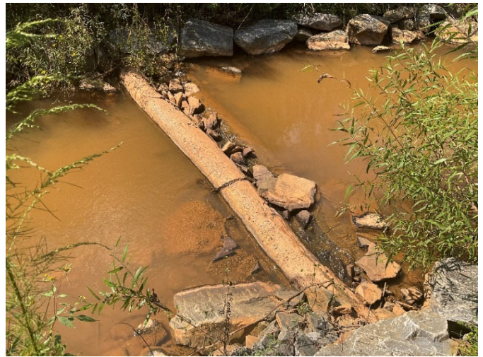
Bull Creek Reach 3: log roller riffle at station 164+00 with one of its header logs dislocated from its footer log (09/19/2022)
