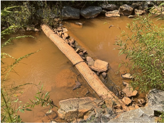
Bull Creek Reach 3: Log roller riffle at station 164+00 with one of its header logs dislocated from its footer log (09/19/2022)
