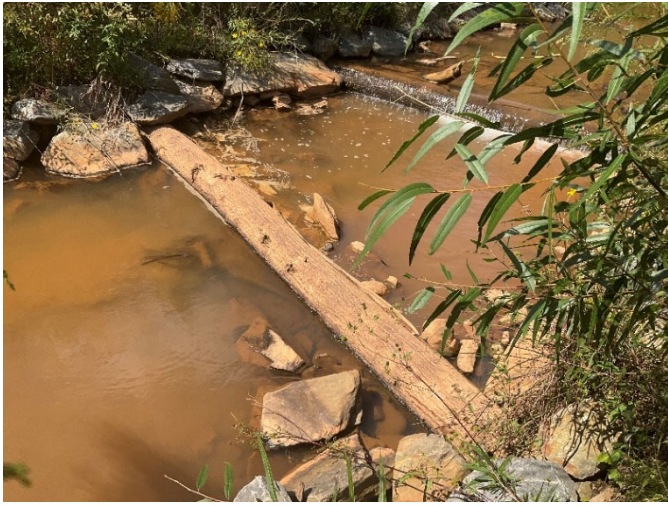
Bull Creek Reach 3: Log roller riffle at station 164+00 with piping under one of the structure's logs (09/19/2022)
