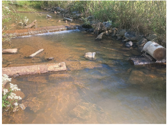
Bull Creek Reach 3: Log cut at station 164+00, water is able to flow freely (09/06/23)
