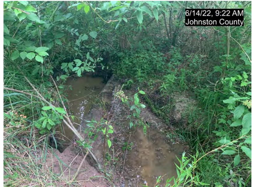
SPA2 (after repair), June 14, 2022 (MY-05)
