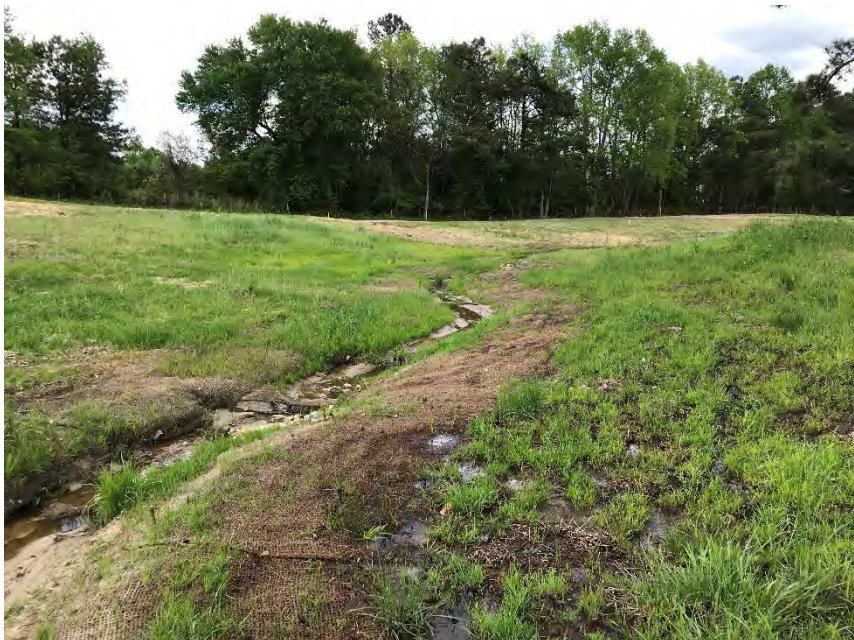
PS-3, R1, facing upstream, Sta 17+50, April 27, 2018 (MY-00)
