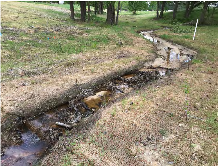
PS-7, R2, facing upstream, Sta 28+25, April 27, 2018 (MY-00)
