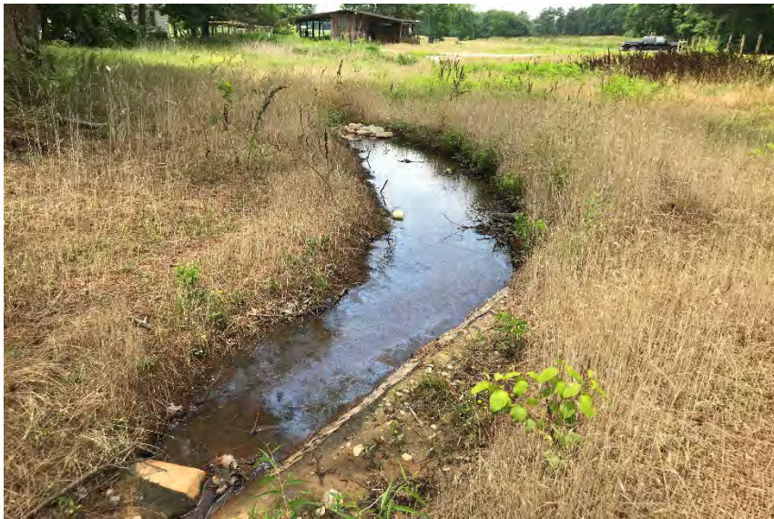
PS-1, R1, facing downstream, Sta 11+50, June 11, 2018 (MY-00)
