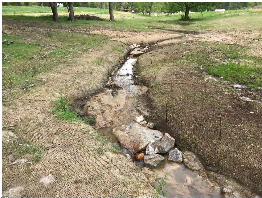
PS-5, R2, facing upstream, Sta 26+50, April 27, 2018 (MY-00)
