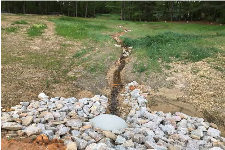
PS-2, R1, facing upstream, Sta 13+50, April 27, 2018 (MY-00)
