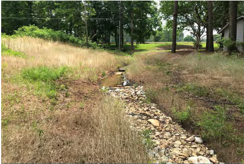
PS-1, R1, facing upstream, Sta 11+50, June 11, 2018 (MY-00)
