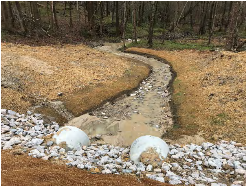
PS-10, R4, facing downstream, Sta 40+00, March 20, 2018 (MY-00)
