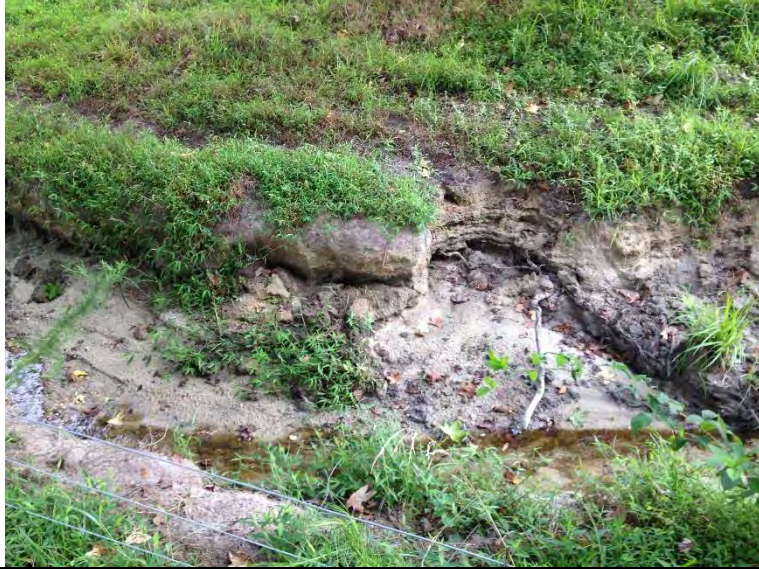
Reach 2 - Eroded bank after Hurricane Matthew (10/19/16)
