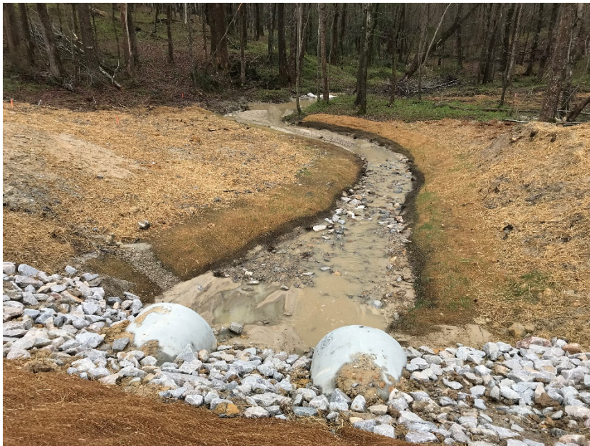
R4, facing downstream, Sta 40+00, March 20, 2018 (MY-00)
