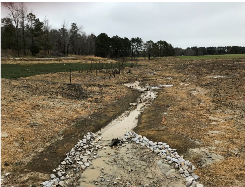
R3, facing upstream, Sta 39+50, March 20, 2018 (MY-00)
