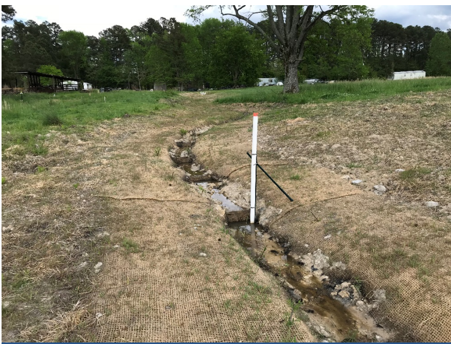
R5, facing upstream, old crest gage, Sta 13+50, Apr 27, 2018 (MY-00)
