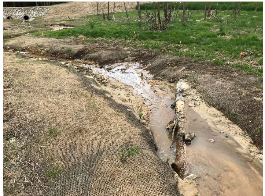
R3, facing downstream, Sta 37+75, April 27, 2018 (MY-00)
