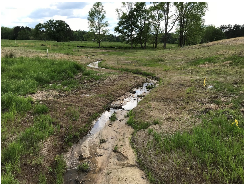
R1, facing downstream, Sta 17+50, April 27, 2018 (MY-00)
