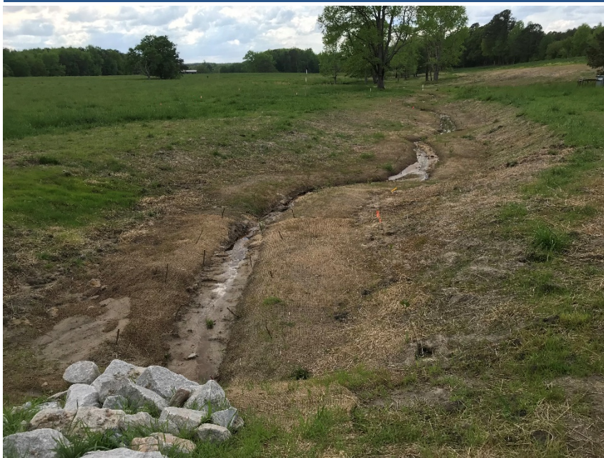
R5, facing downstream, Sta 10+00, April 27, 2018 (MY-00)
