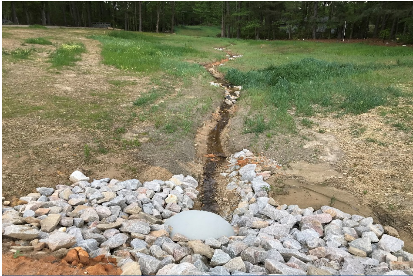
R1, facing upstream, Sta 13+50, April 27, 2018 (MY-00)
