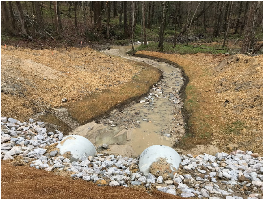
R4, facing downstream, Sta 40+00, March 20, 2018 (MY-00)
