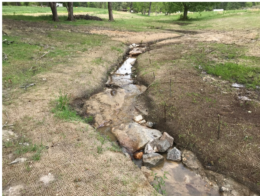
R2, facing upstream, Sta 26+00, April 27, 2018 (MY-00)
