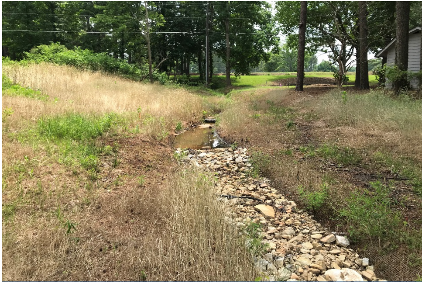
R1, facing upstream, Sta 11+50, June 11, 2018 (MY-00)
