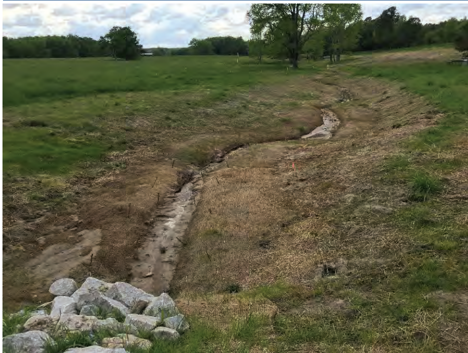
R5, facing downstream, Sta 10+00, April 27, 2018 (MY-00)
