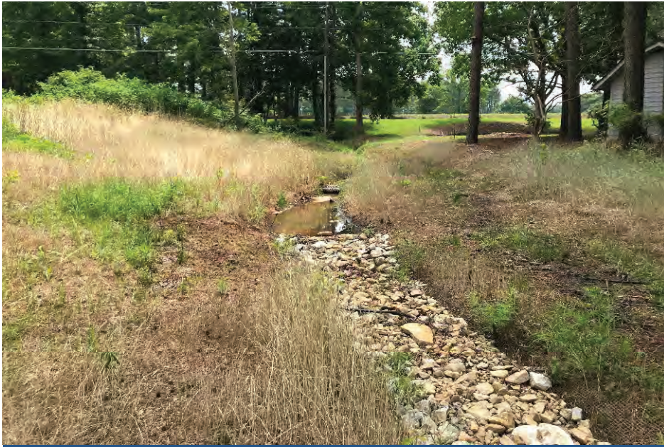
R1, facing upstream, Sta 11+50, June 11, 2018 (MY-00)
