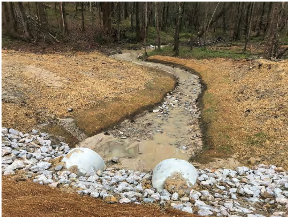
R4, facing downstream, Sta 40+00, March 20, 2018 (MY-00)
