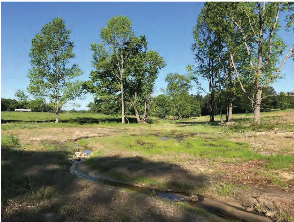
R2, facing downstream, Sta 18+50, April 30, 2018 (MY-00)
