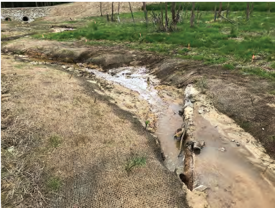
R3, facing downstream, Sta 37+75, April 27, 2018 (MY-00)
