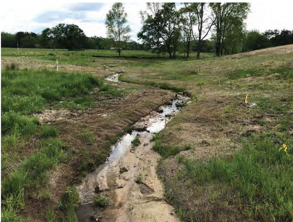
R1, facing downstream, Sta 17+50, April 27, 2018 (MY-00)
