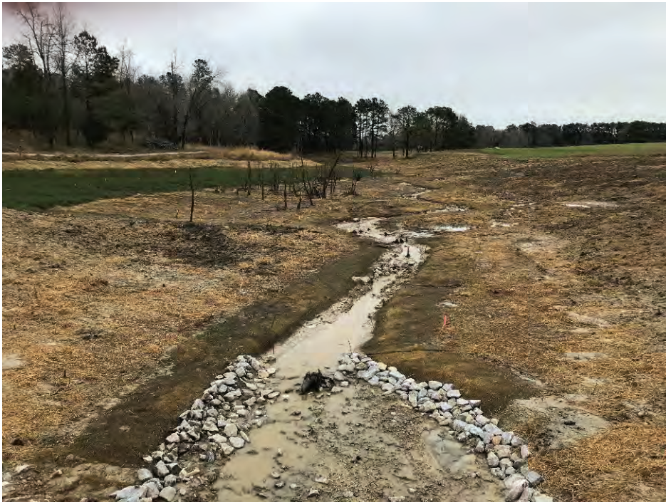
R3, facing upstream, Sta 39+50, March 20, 2018 (MY-00)
