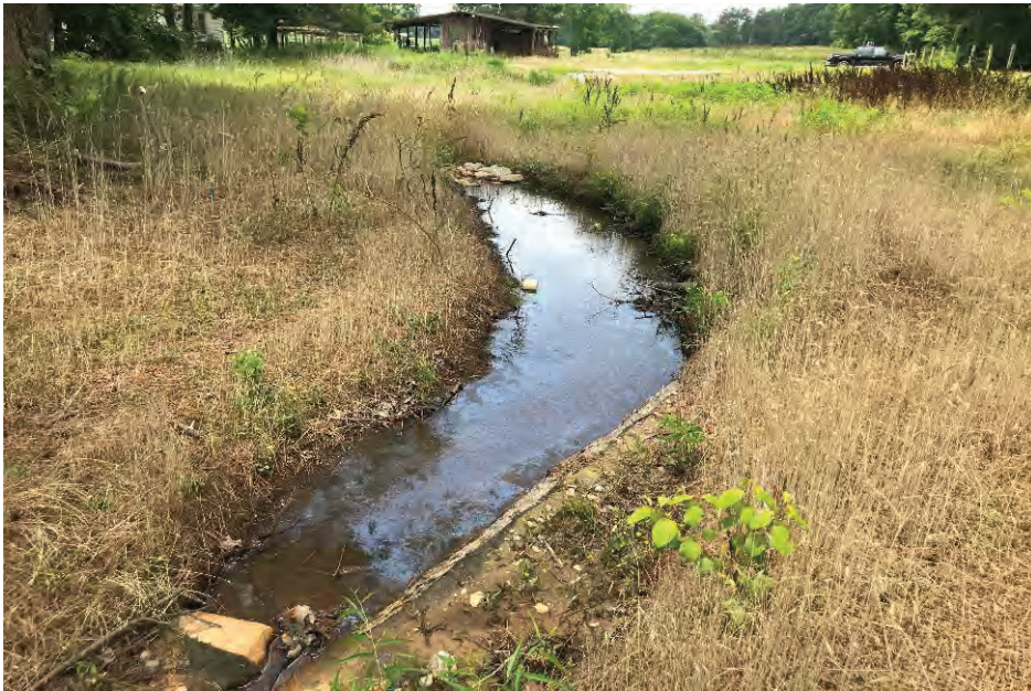
R1, facing downstream, Sta 11+50, June 11, 2018 (MY-00)
