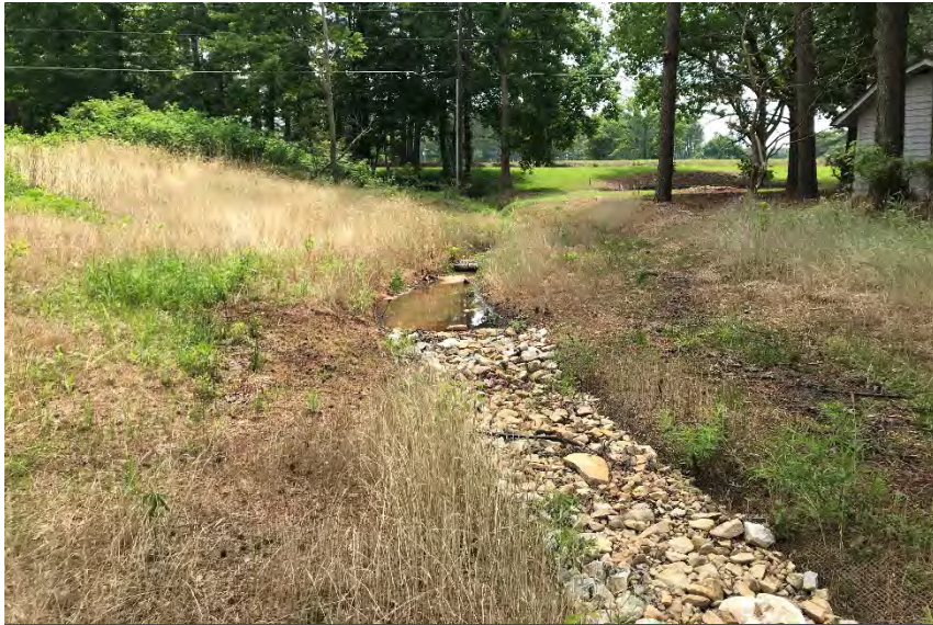
PS-1, R1, facing upstream, Sta 11+50, June 11, 2018 (MY-00)
