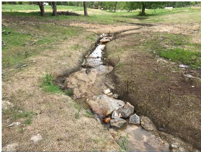
PS-5, R2, facing upstream, Sta 26+50, April 27, 2018 (MY-00)
