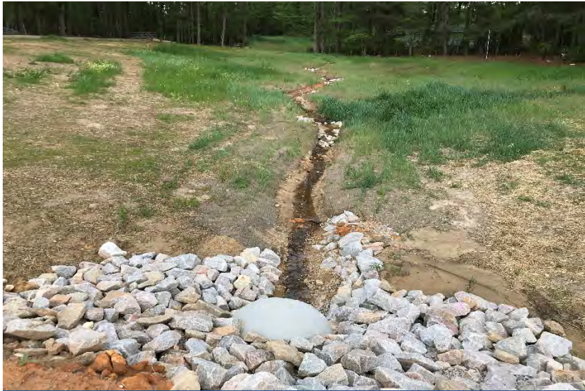
PS-2, R1, facing upstream, Sta 13+50, April 27, 2018 (MY-00)
