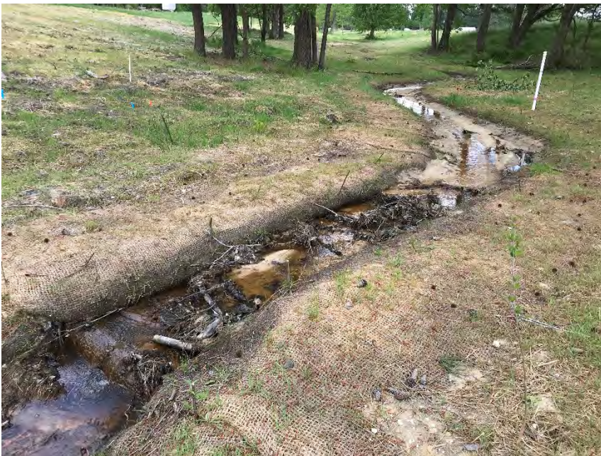
PS-7, R2, facing upstream, Sta 28+25, April 27, 2018 (MY-00)
