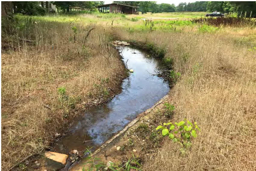
PS-1, R1, facing downstream, Sta 11+50, June 11, 2018 (MY-00)
