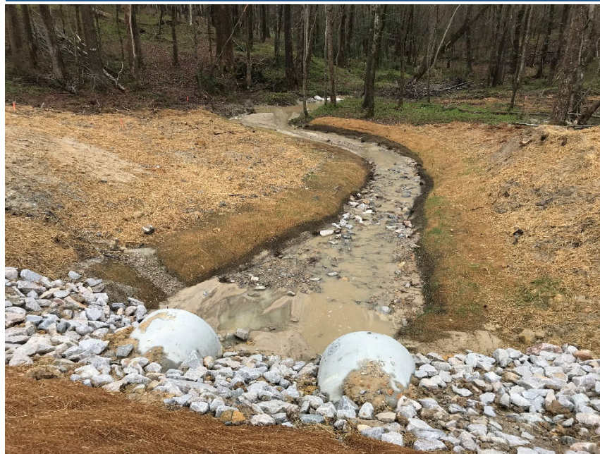
PS-10, R4, facing downstream, Sta 40+00, March 20, 2018 (MY-00)
