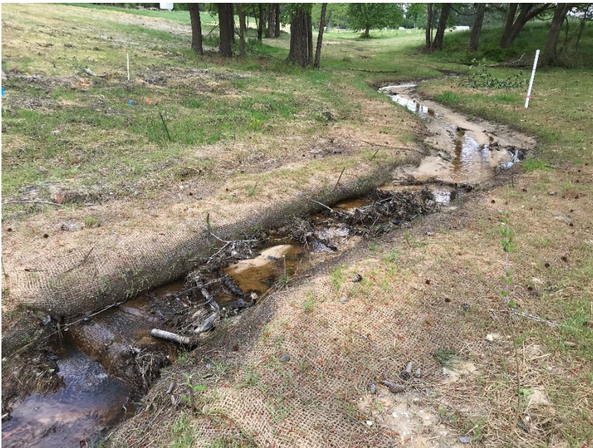
PS-7, R2, facing upstream, Sta 28+25, April 27, 2018 (MY-00)
