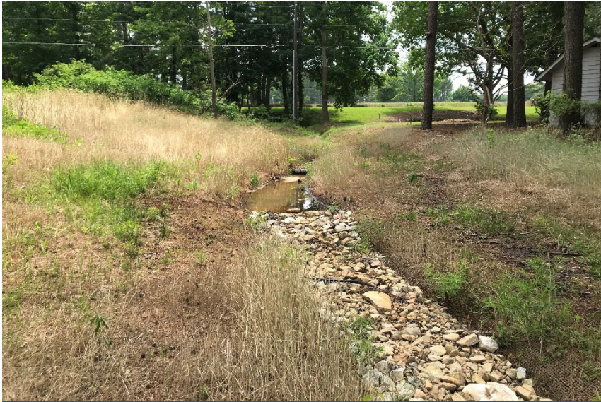
PS-1, R1, facing upstream, Sta 11+50, June 11, 2018 (MY-00)
