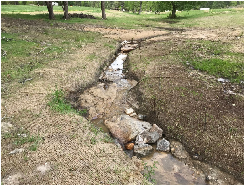
PS-5, R2, facing upstream, Sta 26+50, April 27, 2018 (MY-00)
