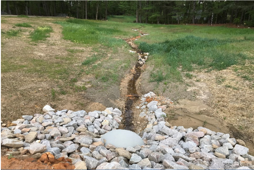
PS-2, R1, facing upstream, Sta 13+50, April 27, 2018 (MY-00)
