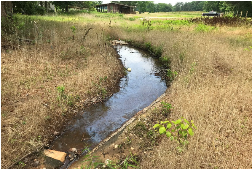
PS-1, R1, facing downstream, Sta 11+50, June 11, 2018 (MY-00)
