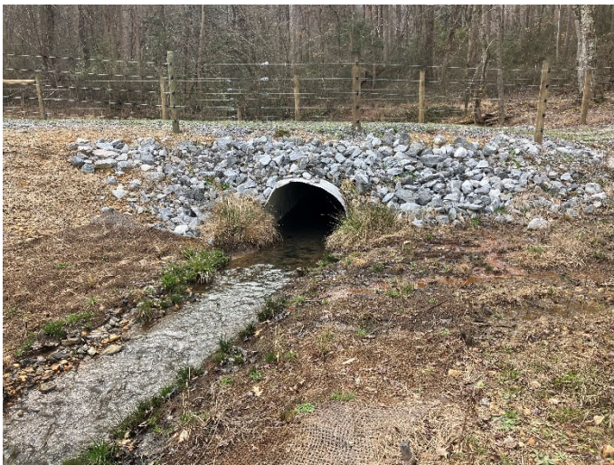
PP13 – view upstream—UT2 (2/20/2023)
