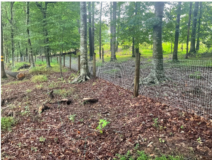
UT1 – Fence repair (8/29/2023)
