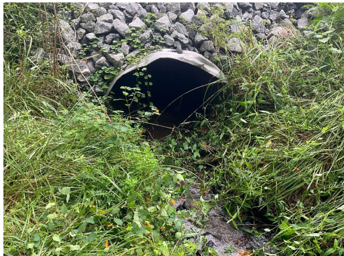
PP13A – view downstream—UT2 (8/29/2023)
