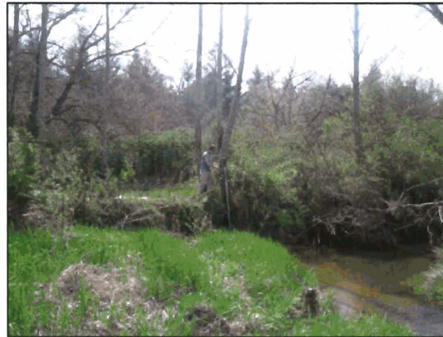
7. Crest Gauge Looking Downstream 7.3.2007
