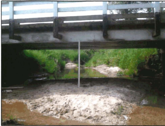
5. Mid-Channel Bar at RD Bridge 7.3.2007
