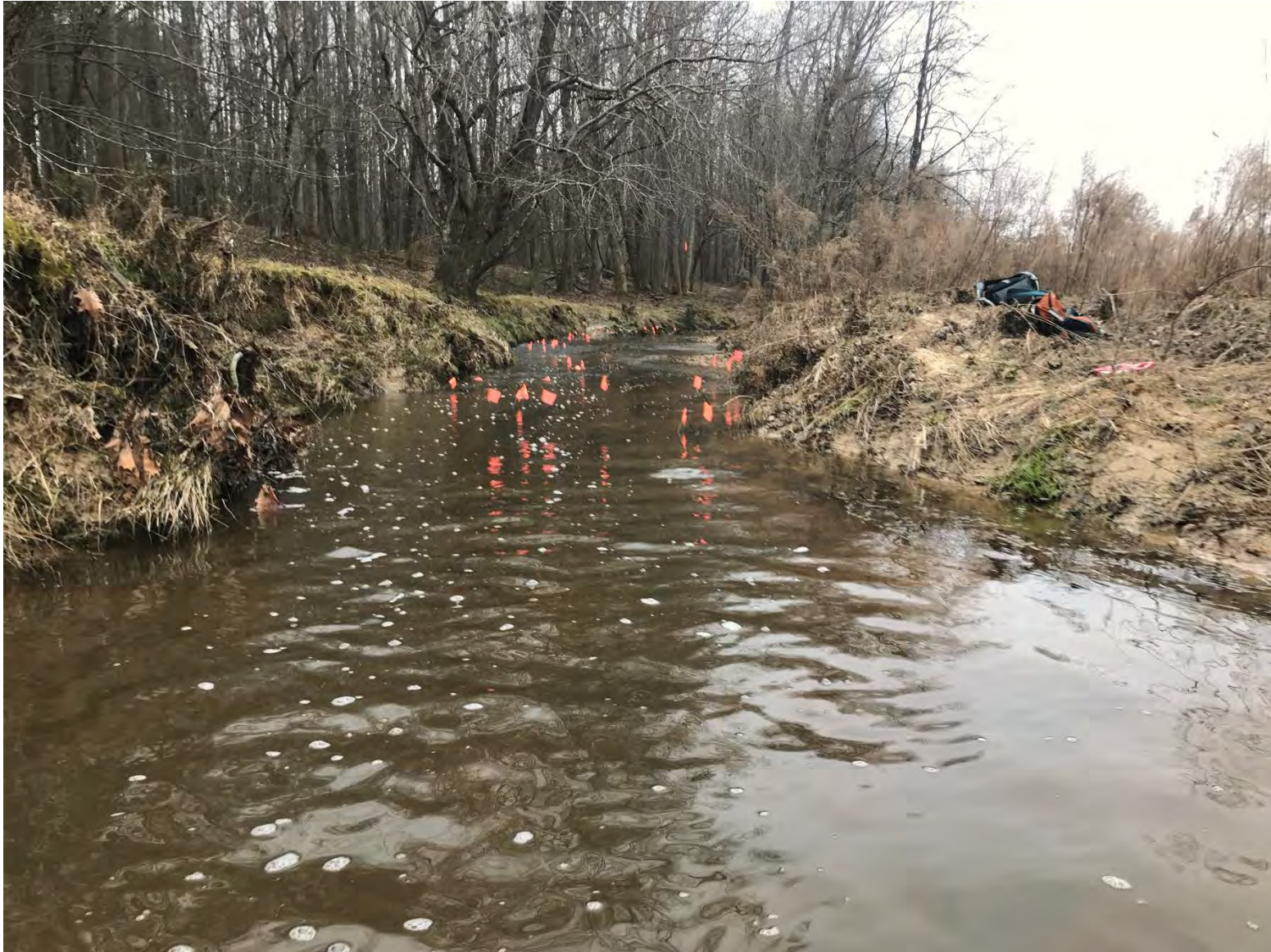
Reach 7 (@ Station 600) facing upstream.
