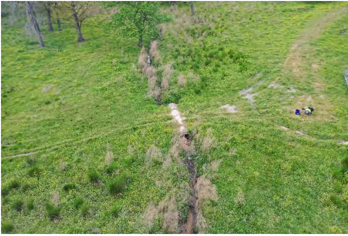
Micah Creek – existing culvert
