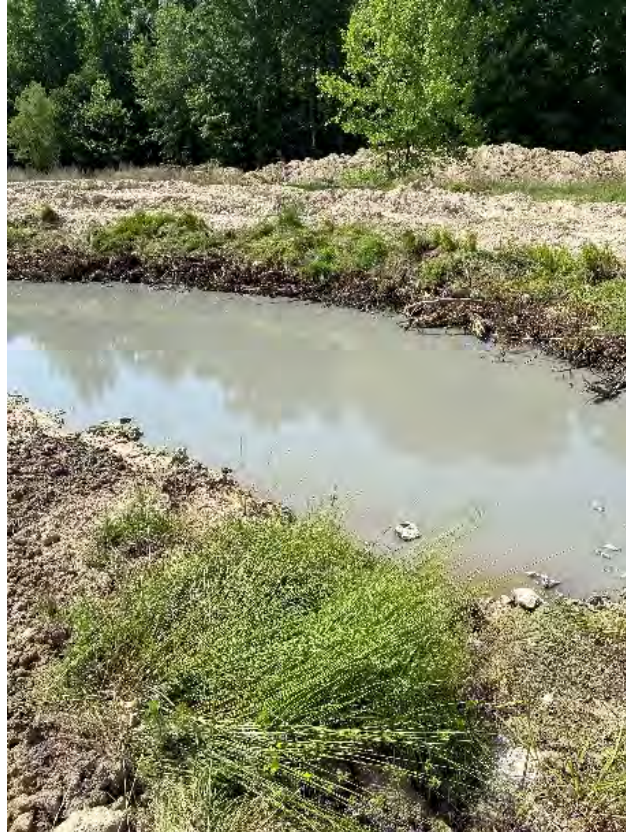
Lunker Box Installation (8/04/2022)
