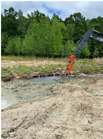
Lunker Box Installation (8/04/2022)
