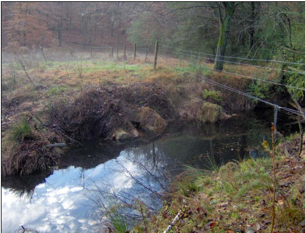
Bank Erosion at Wallace Branch, STA 10+00 11/27/07 Photo No. 20
