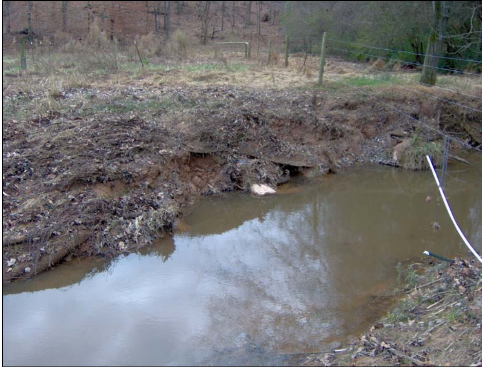
Bank Erosion at Wallace Branch, STA 10+00 12/03/06 Photo No. 19
