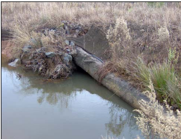
Piping at Log Vane on Lick Creek, STA 29+50 11/27/07 Photo No. 23
