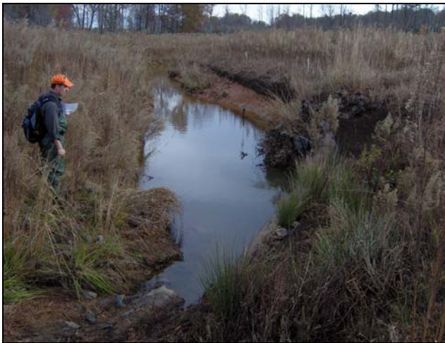
Piping at Log Vane on Lick Creek, STA 29+50 11/27/07 Photo No. 22
