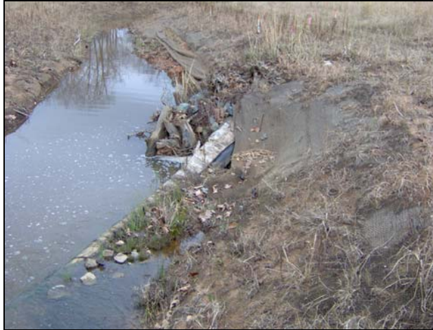
Piping at Log Vane on Lick Creek, STA 29+50 12/03/06 Photo No. 21
