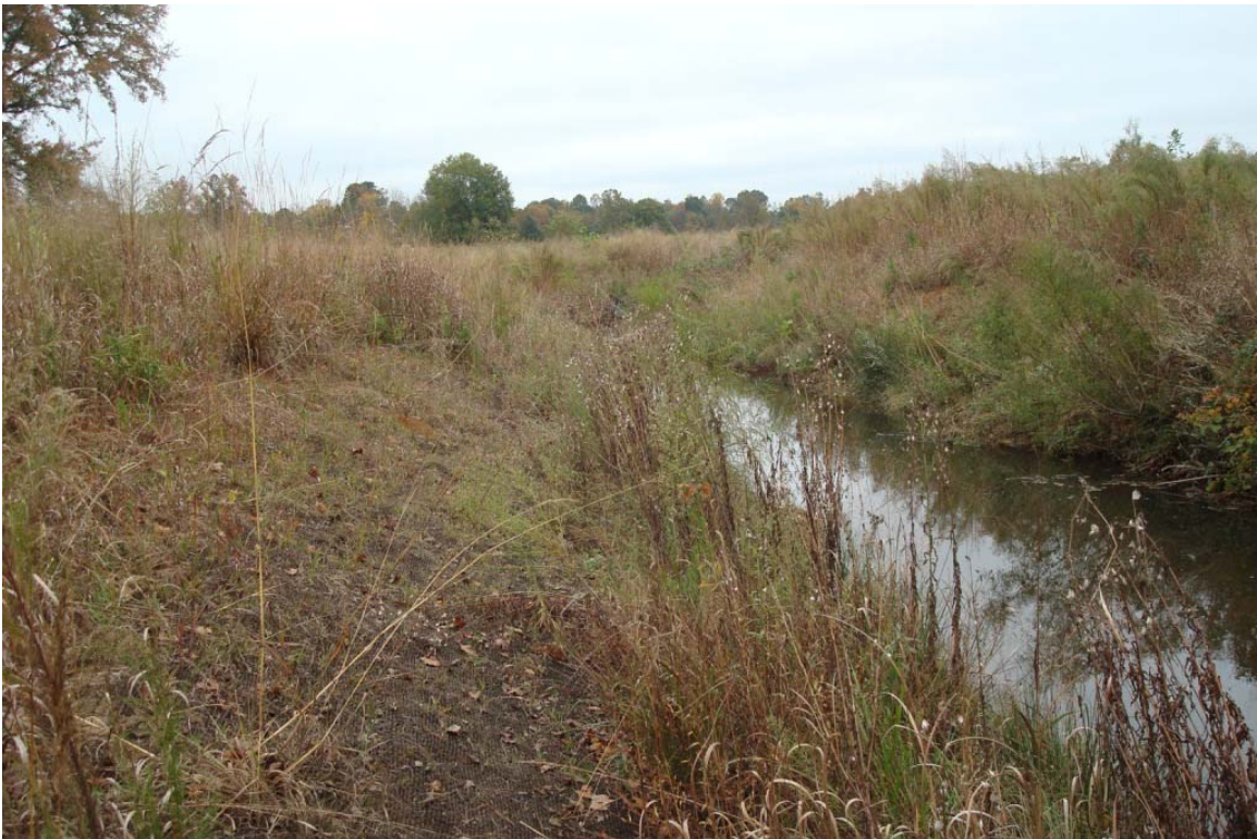
Weak Bank Vegetation on Wallace Branch, Sta 42+40
