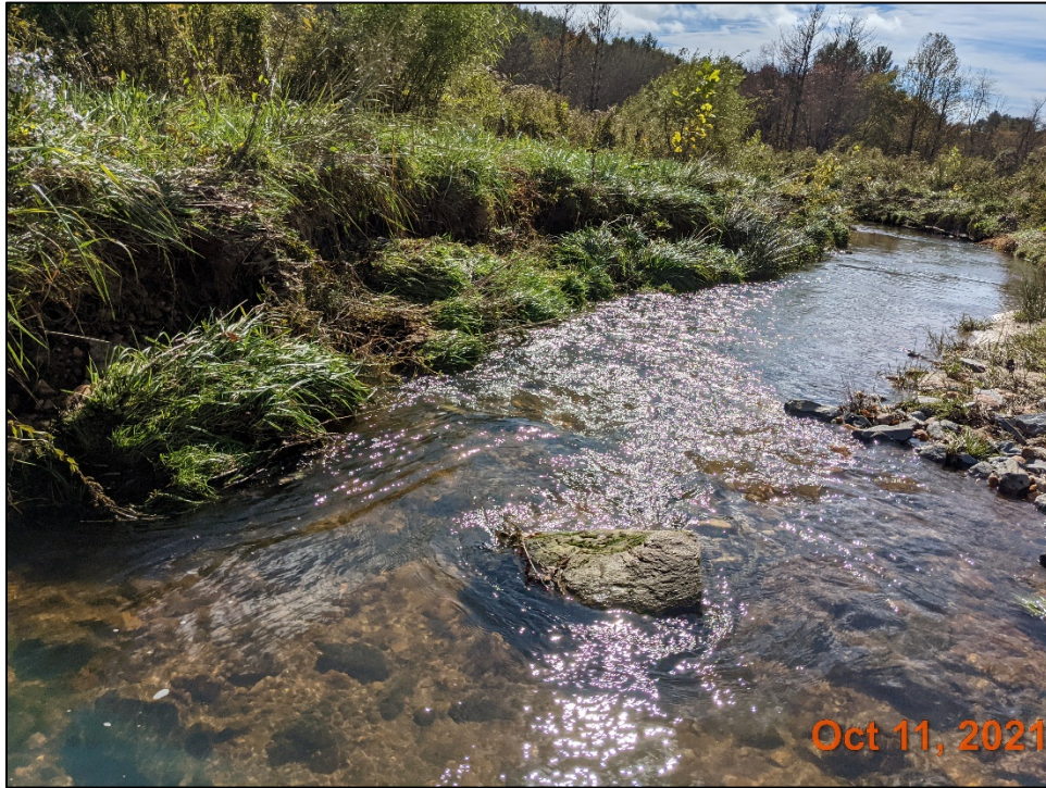
LPCII Reach 2A undercut bank and slump, Station 110+25
