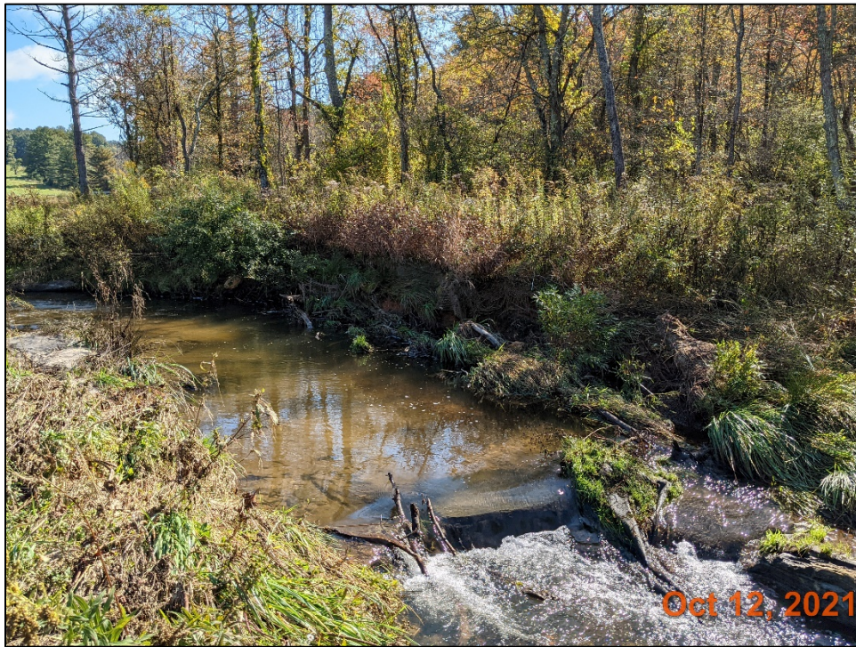
LPCII Reach 2A Bank Scour, Station 120+75
