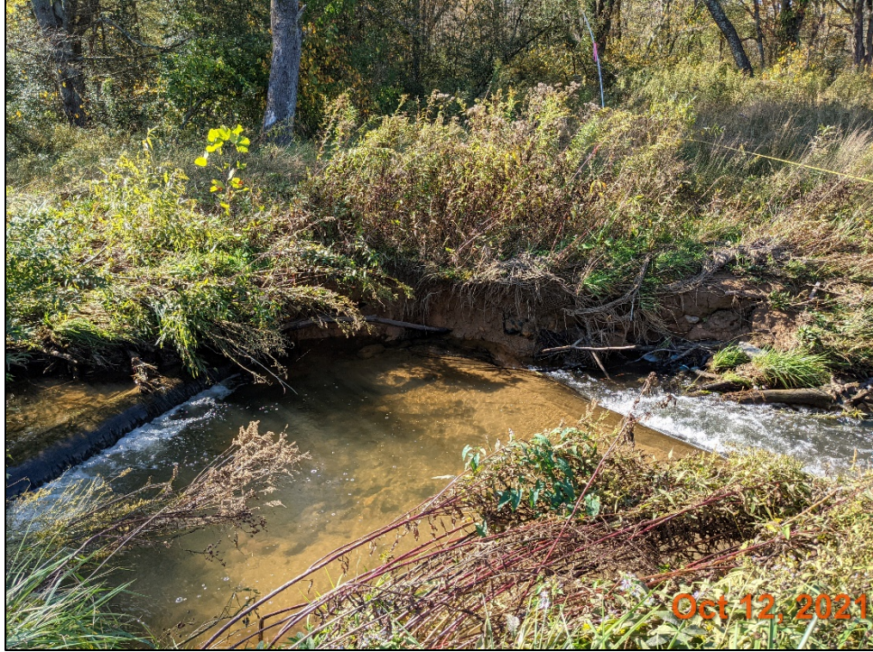
LPCII Reach 2B, Bank Scour, Station 121+50
