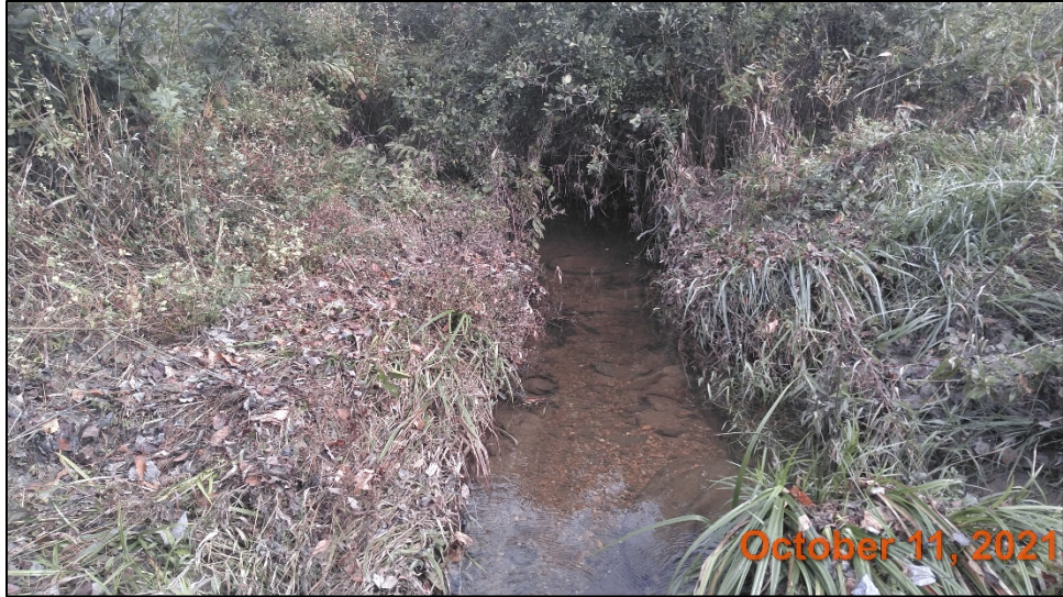
1. Wrack lines and sediment deposits, LPCII Tributary A.
