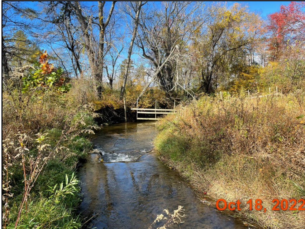
Little Pine Creek II – Permanent Photo Station 12a, Looking Downstream
