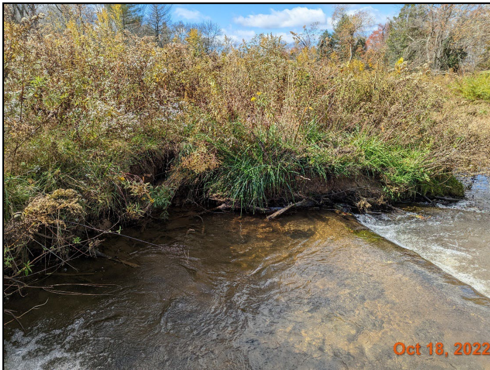
Little Pine Creek II Reach 2A –Bank Erosion Station 118+00 facing left descending bank
