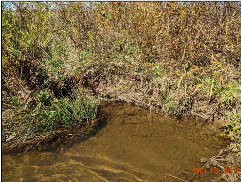
Little Pine Creek II Reach 2A – Slump Bank Station 113+60
