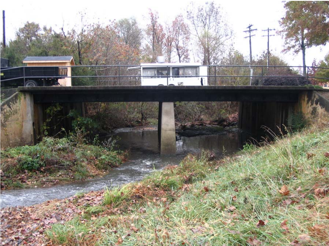
Little Alamance Creek downstream end of project at Overbrook Road.
