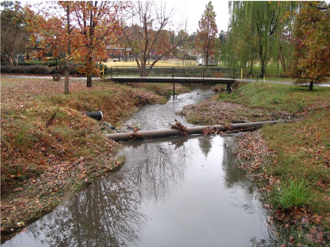
Sewer line and pedestrian/vehicle bridge crossing Little Alamance Creek
