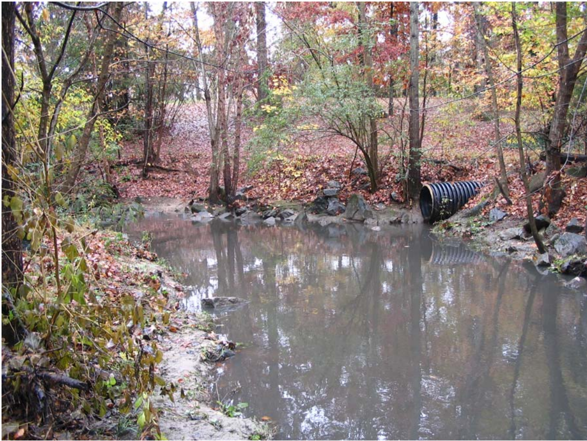
One of several culverts entering Little Alamance Creek. Note Rip rap banks.
