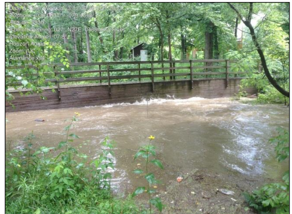
View of Bridge at XS 4 July 3, 2013
