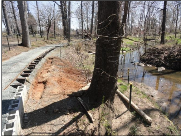
Photo Station 1, rail line at bollard 172, facing east; April 3, 2013
