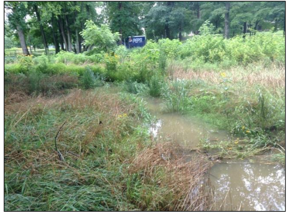
View from PS 2, level spreader July 3, 2013
