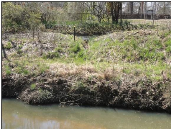
Photo Station 3, rail line discharge, facing south; April 3, 2013
