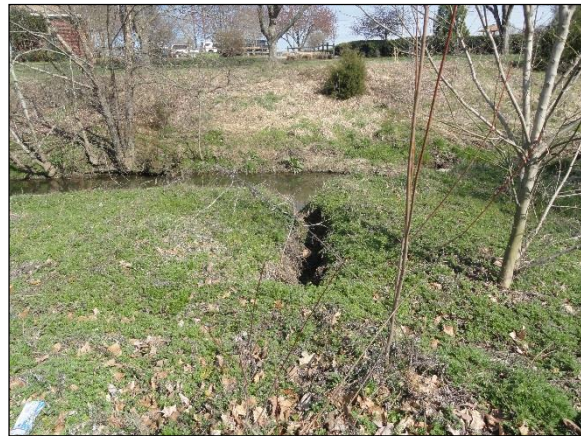
Photo Station 4, discharge at bollard 312, facing west; April 3, 2013
