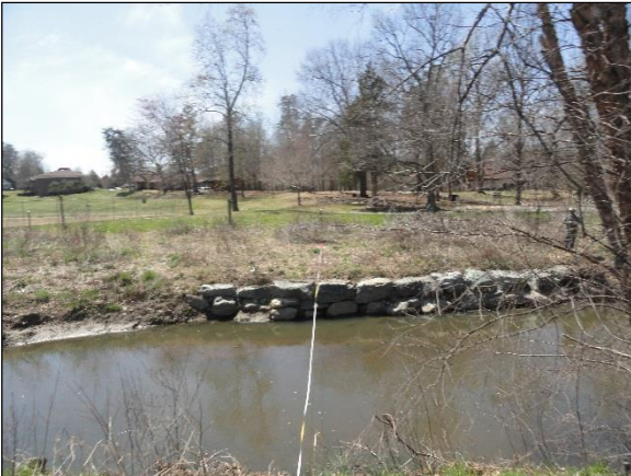
Photo Station 13, XS 7, facing right bank; April 3, 2013
