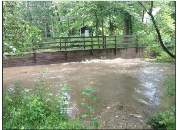
View of Bridge at XS 4 July 3, 2013
